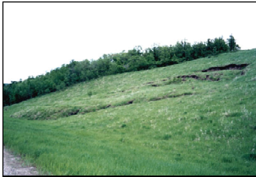
Fig. 6. Failure in cut slope near Virden , Manitoba (Blatz et al. 2004)
