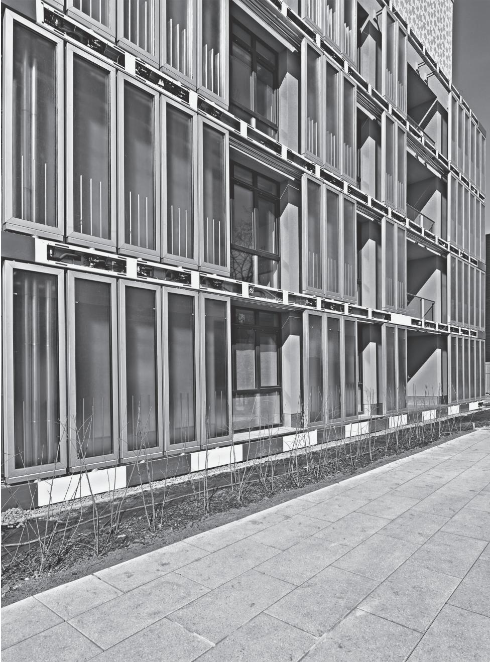
*Figure 9.4* BIQ building, Hamburg, by Arup, exploits algae in façade
