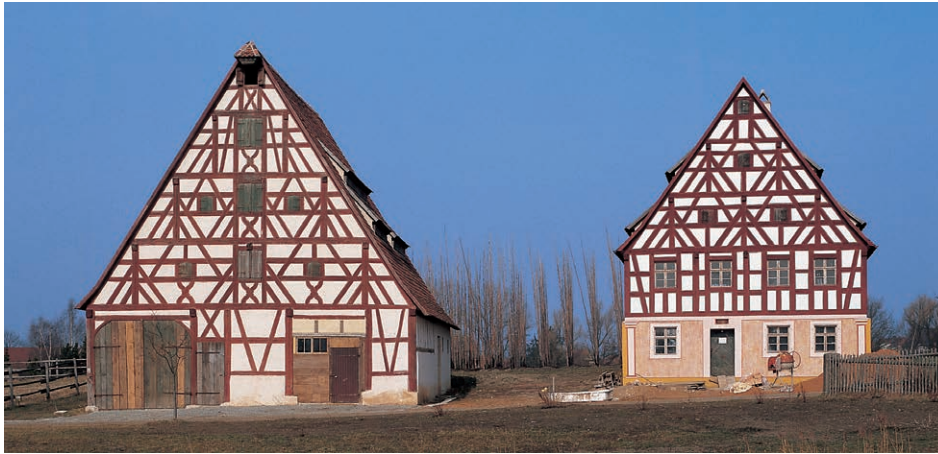
A 6 Farmhouses, open-air museum, Bad Windsheim, Germany
