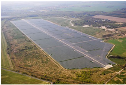
PV as large as airports? (Saxony, Germany)
