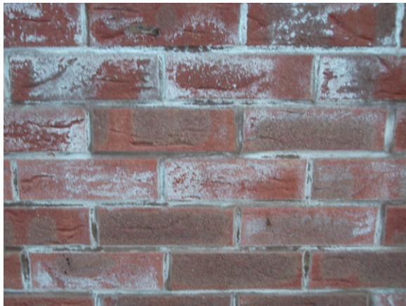
Figure 16.3 Brick efflorescence.
