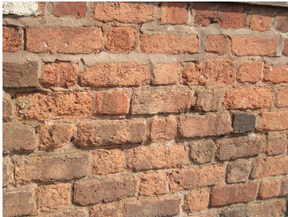
Figure 16.2 Brick spalling.
