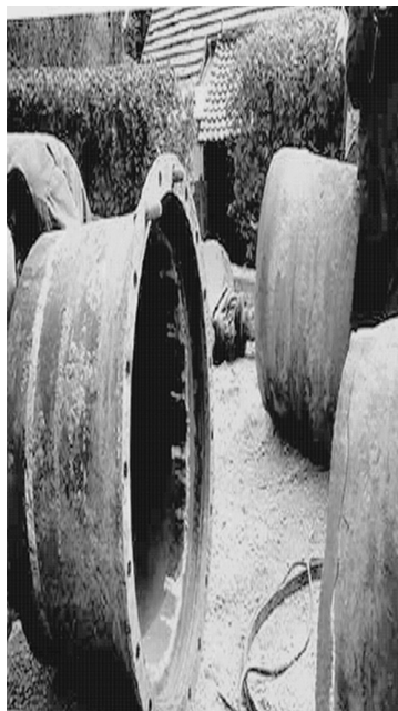
FIGURE 20.5 Digging of mechanical joint of a ductile cast iron pipe of 900 mm diameter.
