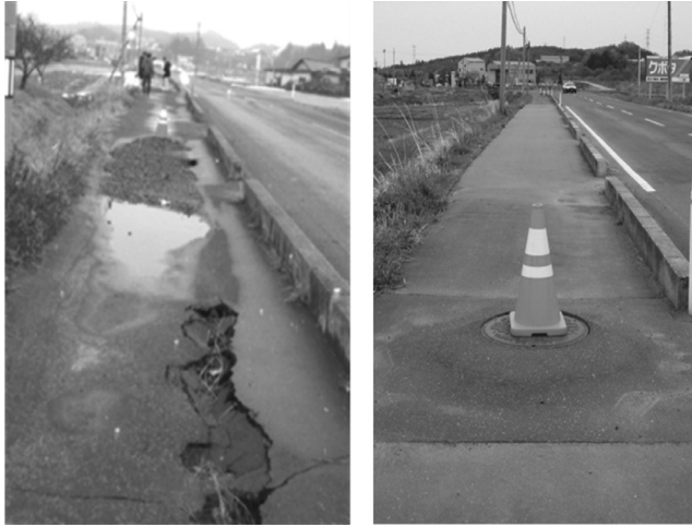
PHOTO 21.13 Effects of backfill solidification as liquefaction countermeasure observed in Kurihara city, Miyagi, prefecture in the 2011 off the Pacific coast of Tohoku earthquake. (The section in the left photo had not been solidified, while the one in the right photo had been solidified.) (Courtesy of Japan Sewage Works Association, Tokyo, Japan.)
