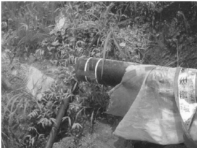
FIGURE 20.37 Pulling out of mechanical joint (K type) of ductile cast iron pipe.
