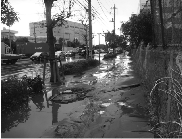
PHOTO 21.12 Liquefaction in Shin-Kiba, Koto ward, Tokyo, caused by the 2011 off the Pacific coast of Tohoku earthquake. (Courtesy of Japan Sewage Works Association, Tokyo, Japan.)
