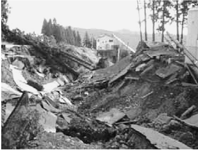
FIGURE 20.27 Landslide near the purification plant.
