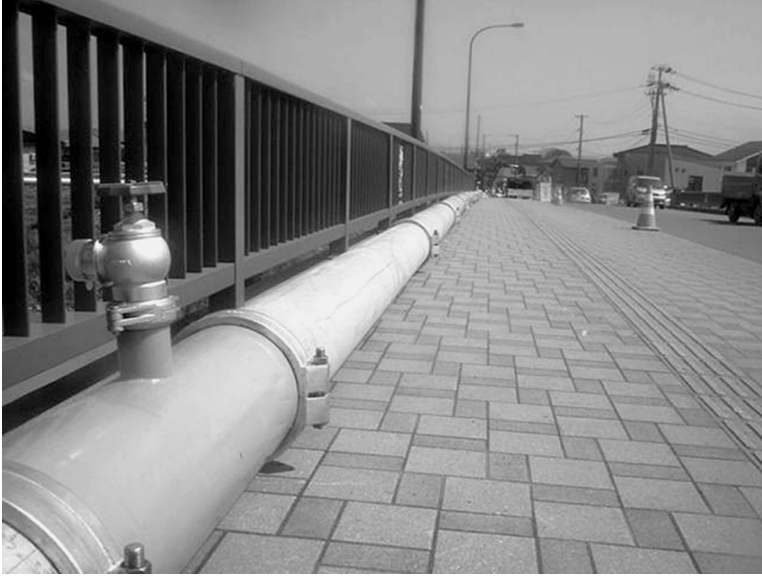
FIGURE 14.13 Temporary pipe laying in the 2007 Niigata Chuetsu-Oki earthquake.
