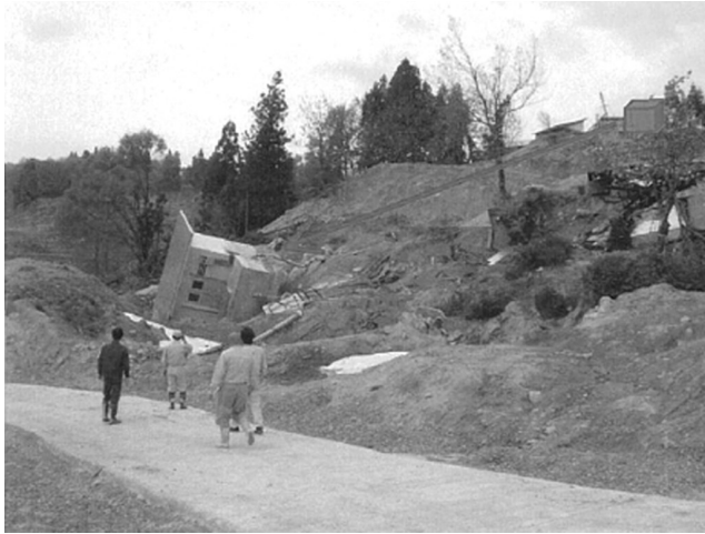
FIGURE 20.31 Landslide at No. 5 pumping station.
