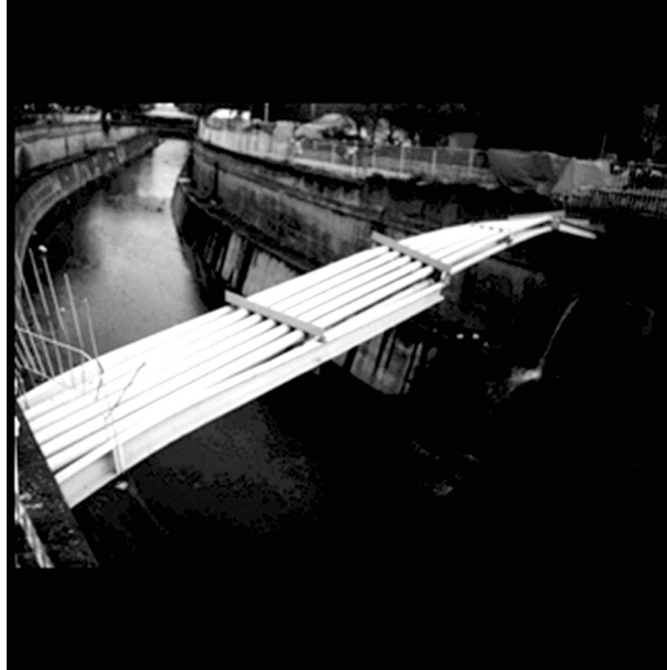
FIGURE 24.3 Damage to a private bridge.
