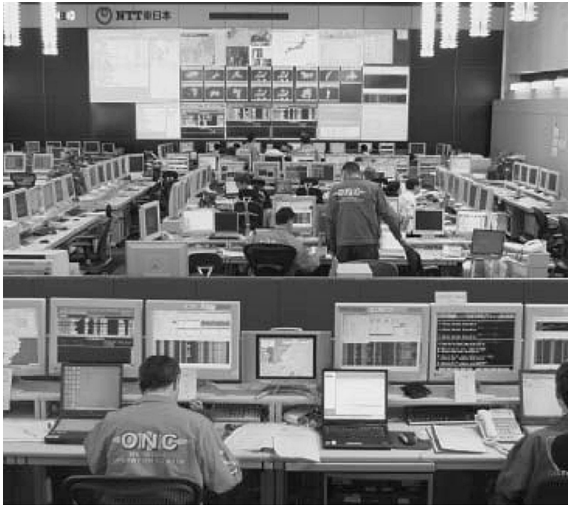
FIGURE 24.13 Network operation center.
