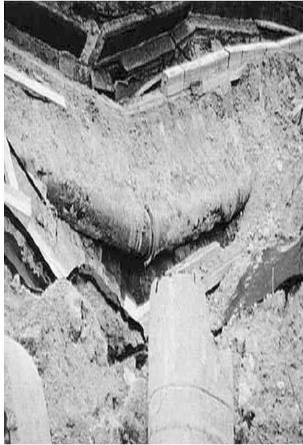
FIGURE 20.14 Pulling out of cast iron pipe of 450 mm diameter.
