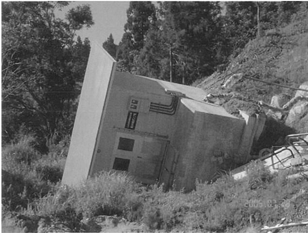
FIGURE 20.30 No. 5 pumping station slipping down due to slope failure.
