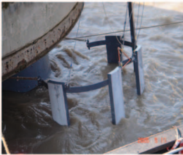
FIG.3 Installation of cathode protection system
