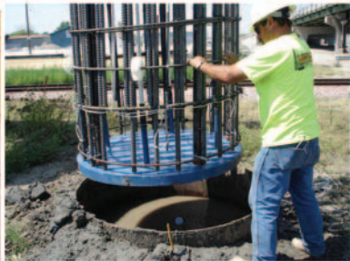
Figure 2. Grout plate affixed to toe of cage
