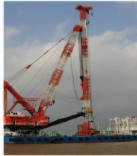
FIG.4 Haili 801# pile-sinking barge
