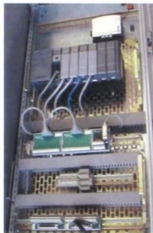
FIGURE 1-15 PLC in an industrial environment. (Courtesy of Famic UK, Ltd.)
