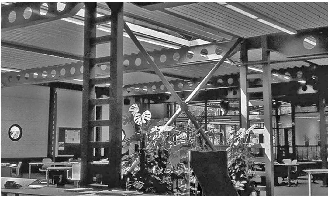
Figure 6.32. Battened columns
