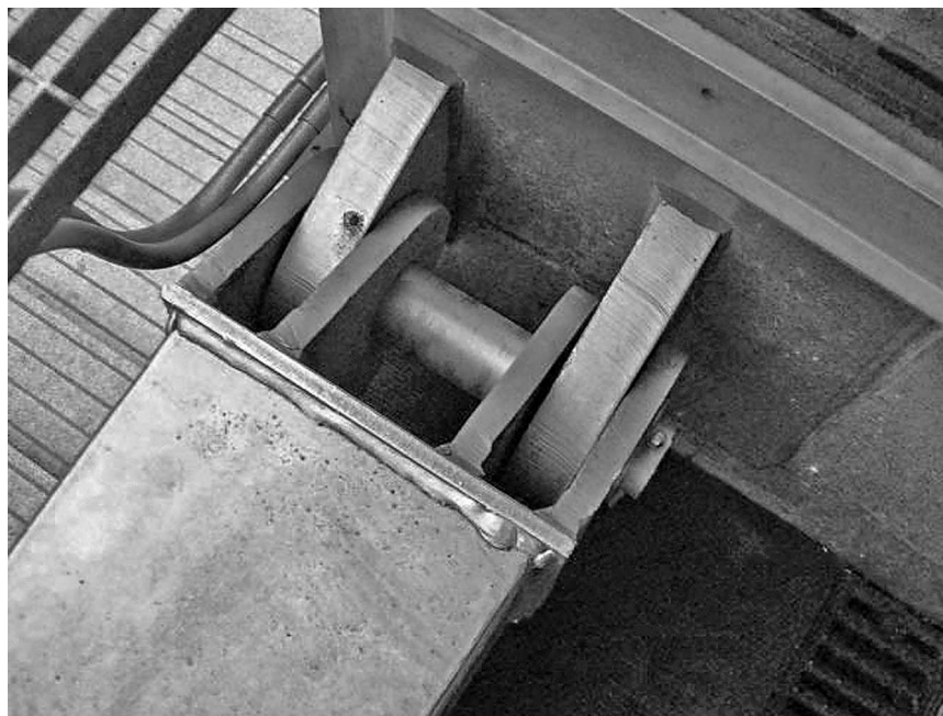
Figure 12.4. Pin connection
