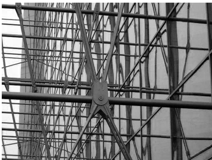
Figure 5.3. External diagonal bracing system (Sanomatalo Building, Helsinki)
