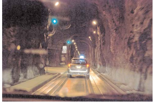
FIGURE 7 Whittier Tunnel interior: combined-use for road and railway vehicles.
