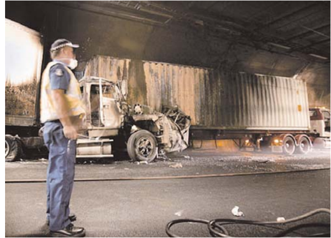
FIGURE 4 Burnley Tunnel (Australia) after fire.
