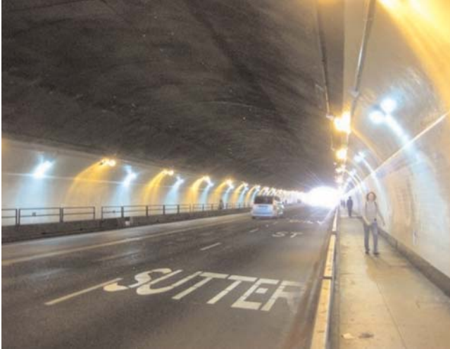
FIGURE 5 Tunnel with pedestrian walkways all along the tunnel for pedestrian crossings (San Francisco).
