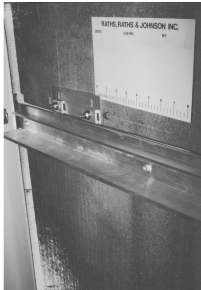
FIG. 3—View of aluminum J-section used to stiffen the upper J-section.
