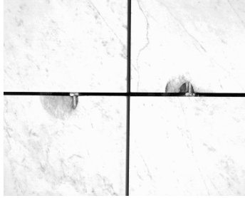
FIG. 9—Cracking at anchoring points due to excessive expansion in relation to the dimensions of “dilatation” joints.
