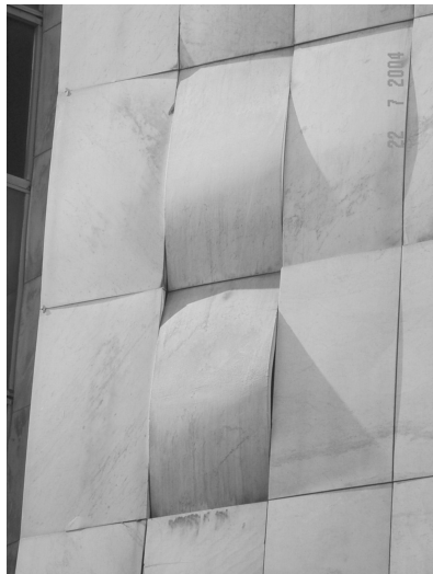
FIG. 15—Zagrepcanka building in Zagreb. Close-up of the façade with panels showing significant different bowing behavior. Photo by Jan Anders Brundin.
