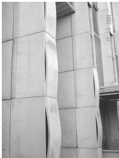
FIG. 2—Bowling of marble panels on Zagrepcanka business tower in Zagreb, Croatia. Photo by Jan Anders Brundin.
