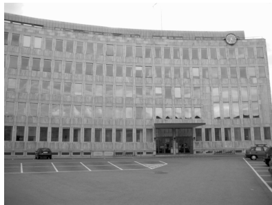
FIG. 9—Lyngby City Hall, Denmark. The 60-year-old marble façade is still in very good condition. Photo by Bent Grell.
