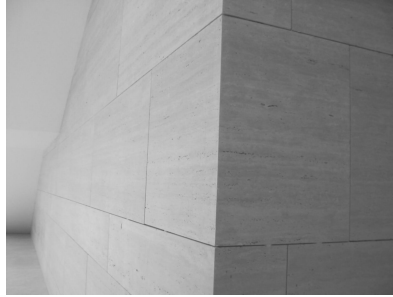
FIG. 1—View of vein-cut travertine wall panels in Museo dell’ Ara Pacis in Rome, Italy.
