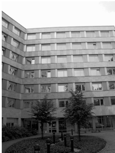
FIG. 8—A Carrara marble façade on Malmo City Hall, Sweden in perfect condition. Photo by Bent Grelk.
