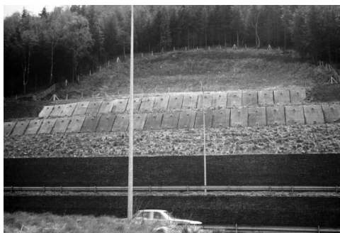
Figure 6.37 Precast slabs used with anchors to provide a retaining structure at the toe of a failing slope (South Wales).
