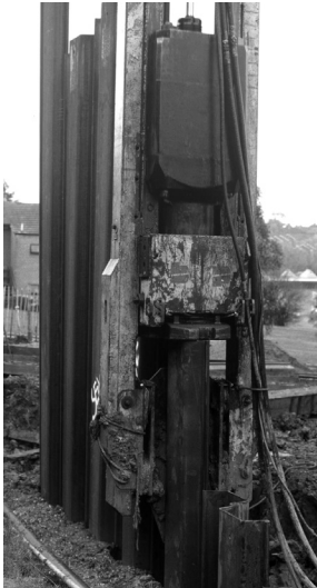
Figure 6.15 Driving Larssen steel sheet-piles.
