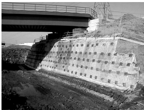
Figure 6.39 Soil-nailed wall along Midland Expressway, UK. (Image courtesy of Phi Group.)
