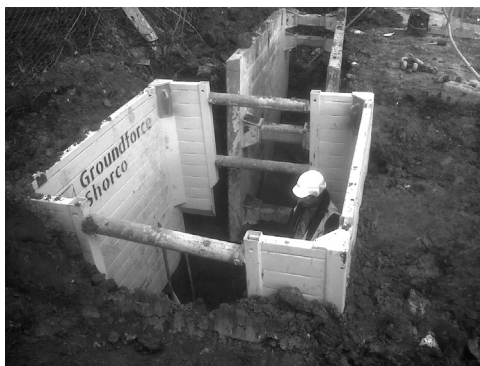
Figure 6.13 Trench support provided by manhole and trench shields (image courtesy of VP plc).
