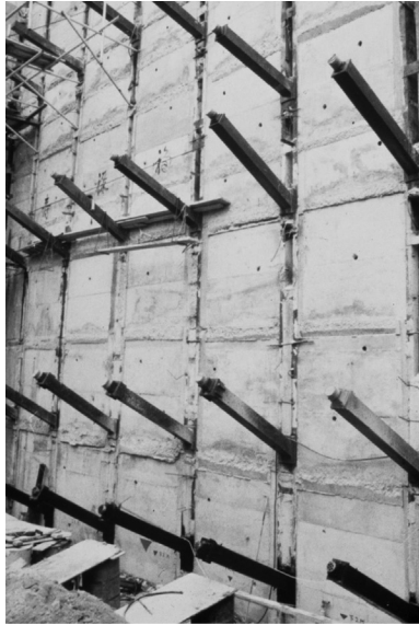
Figure 6.27 Top-down construction using anchored steel H piles in-filled with cast in situ concrete planking (Hong Kong).
