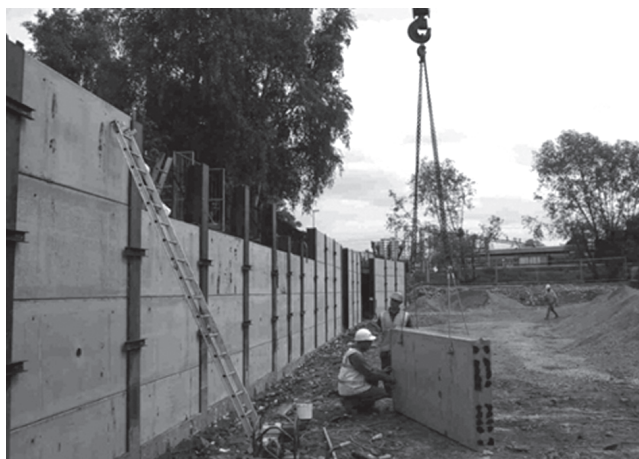
Figure 6.26 King post wall. (a) Plan showing steel H-piles and concrete panels. (b) Wall construction, using pre-cast panels. (Image courtesy of ElecoPrecast.)
