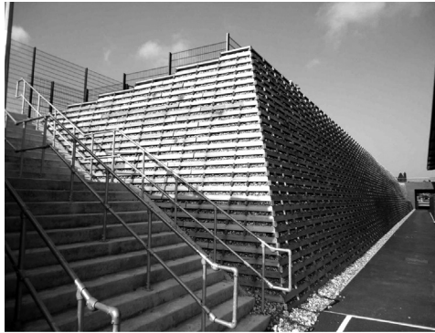
Figure 6.7 Large timber crib wall at University of Surrey.
