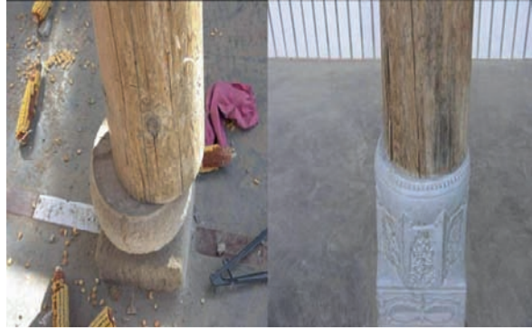
Fig. 47 Different displacements of wood columns of two adobe-wood houses in Haoping village, Wudu district, Longnan city
