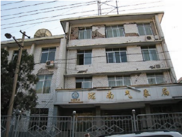
Fig. 20 The weather bureau of Longnan City in Wudu district
