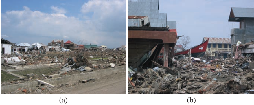
Fig. 12 Destruction of entire residential districts of timber framed structures in Banda Aceh, Indonesia
