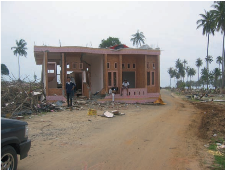
Fig. 13 A single-story house, displaced by water pressure due to lack of proper anchorage, Banda Aceh, Indonesia (See also Color Plate 16 on page 215)
