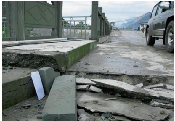
Fig. 28 The settlement of 30 cm at the top the dam of the Zipingpu reservoir
