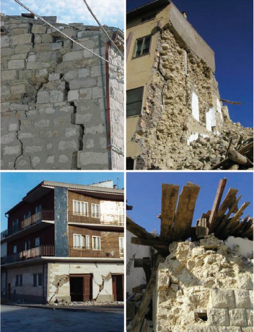
Fig. 6 Typical damage of masonry buildings in S. Giuliano di Puglia
