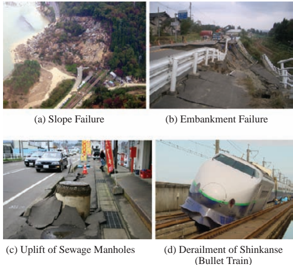
Fig. 8 Disaster by the 2004 Niigata earthquake
