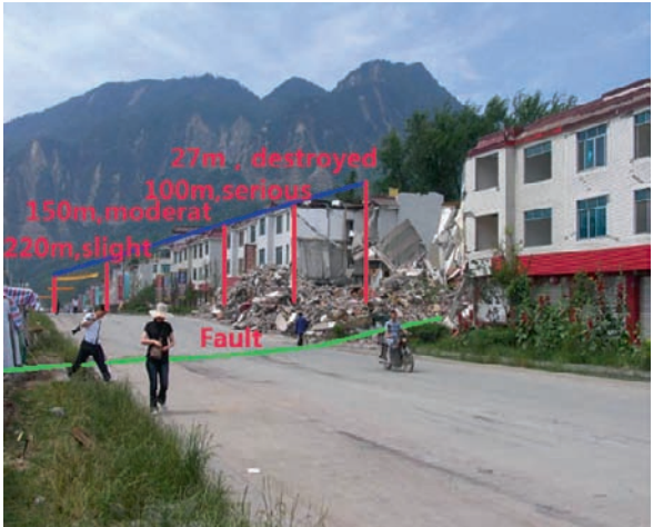
Fig. 38 The fault rupture crossed the Xiaoyudong town
