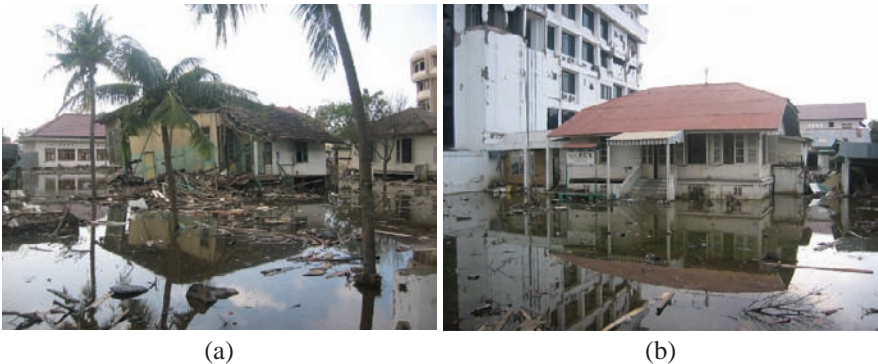
Fig. 11 Timber framed structures in Banda Aced, Indonesia
