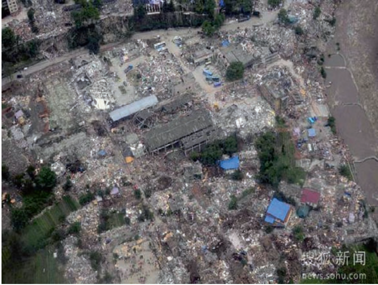
Fig. 3 The Yingxiu town, Wenchuan county, destroyed by the Wenchuan earthquake. (From news.sohu.com)
