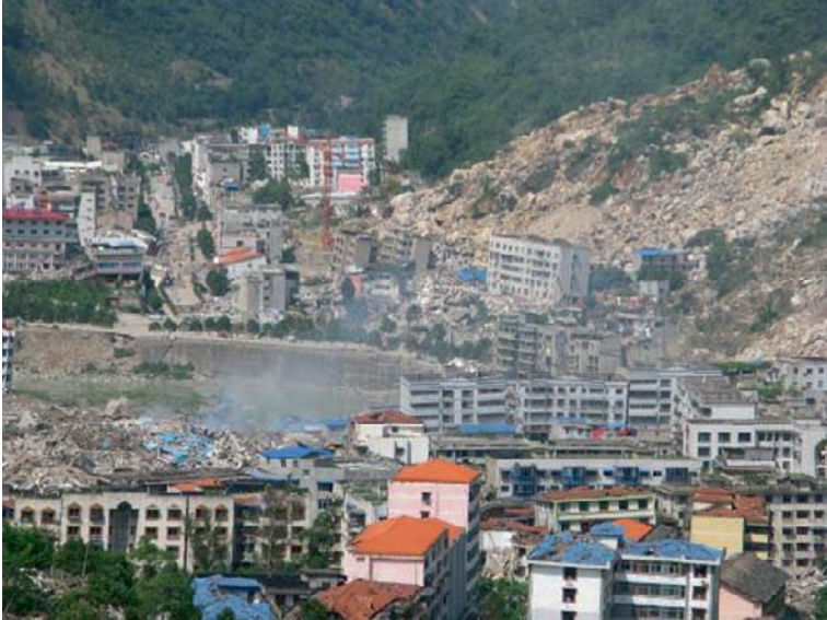
Fig. 2 The Beichuan county, destroyed by the Wenchuan earthquake
