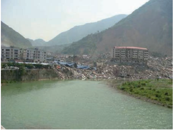
Fig. 37 The fault rupture crossed the Beichuan county. (Towards to SW)
