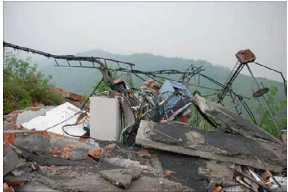
Fig. 33 A set of communication cables was pulled down
