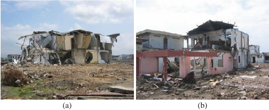
Fig. 10 Failure of confined masonry in Banda Aced, Indonesia
