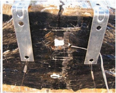
b) Fracture of sheet, Beam 5
