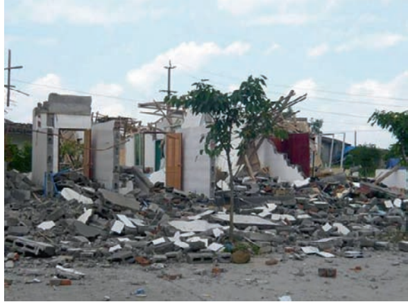
Fig. 21 Collapsed houses in a village located in Jiulong town, Mianzhu city
