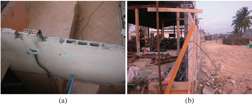
Fig. 8 (a) Typical 50 mm thick concrete block and clay brick masonry units; (b) construction of confined masonry in Khao Lak harbor town in Thailand
