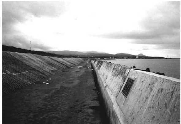
Fig. 16 Opening about 0.5–1.0 m wide behind the sea wall and sand ejected as a result of liquefaction in Ansei area
