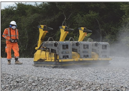
Remotely operated vibrating plate compactors (three heavy duty compactors fixed in a line)
