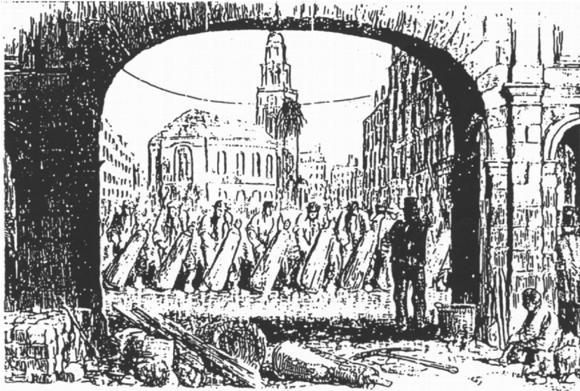
Figure 1.2 Earthworks in the Strand, London, 1851. Note the foreman in the foreground beating time (from Binnie, 1987)
