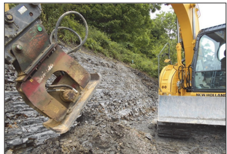
Excavator boom-mounted vibrating plate compactor
