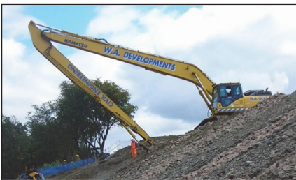
Long reach excavator
