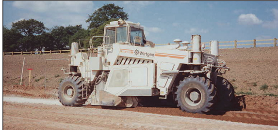
Self-propelled soil stabilisation plant (direction of travel from right to left mixing the binder spread across the ground surface into the soil)
