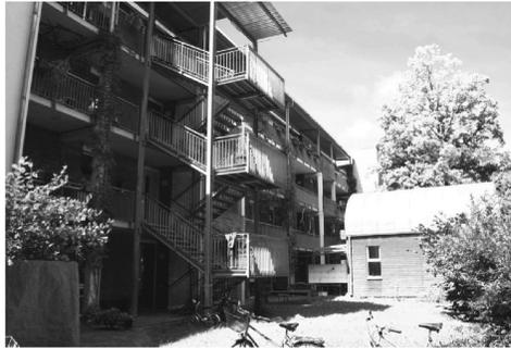
Figure 16.12 Staircases and passageways on a Type B LEN building.
