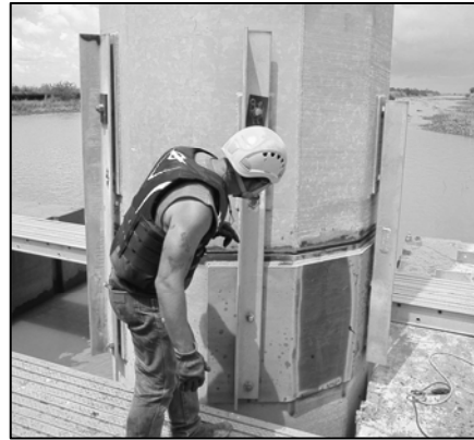
Figure 5 – 2-Piece Pile Support
