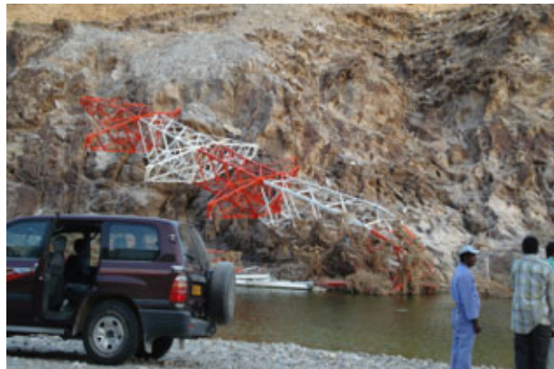
Exhibit No. 5: Damaged Tower
