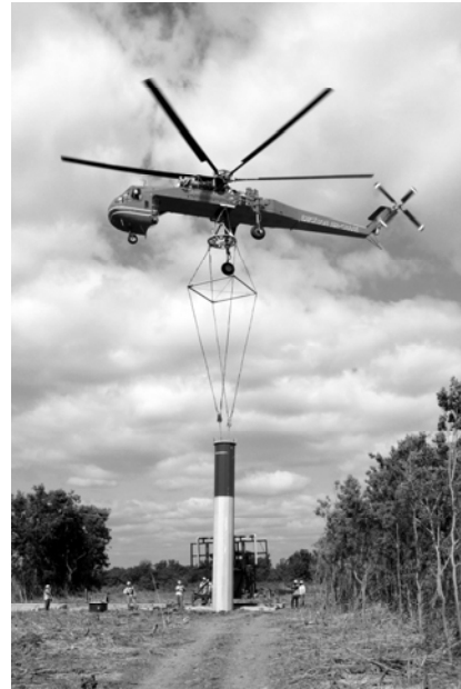
Figure 7b – Positioning Pile
