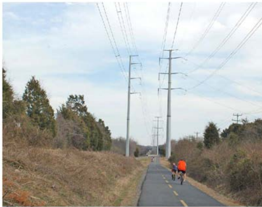
Figure 28: Multi-circuit line and public ROW use (bicycle trails).
