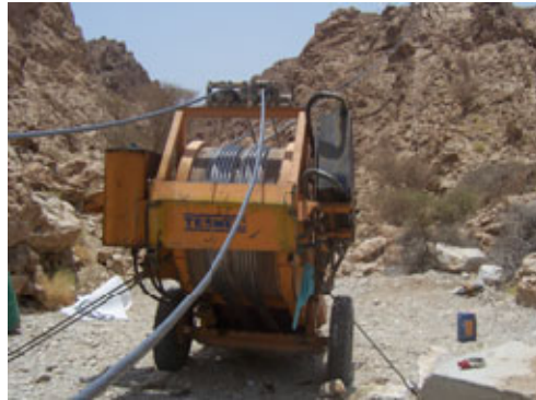
Exhibit No. 20: Stringing of the Conductors
