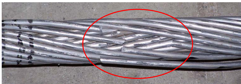
Figure 4 – Fatigue Failures of ACSS Conductor Supported by a Standard Suspension Clamp installed over a set of armor rods
