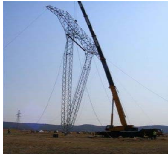
Exhibit No.30: Tower erection by crane.
