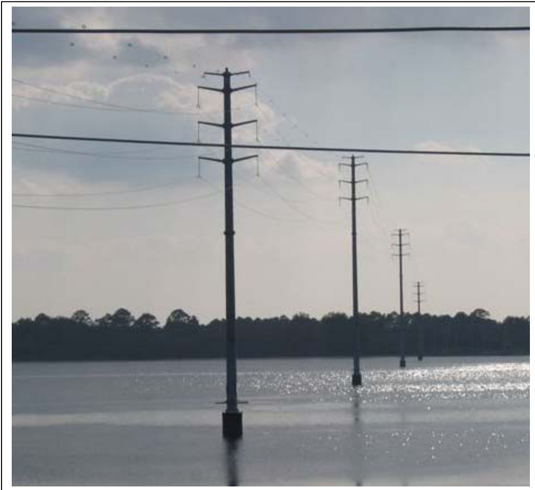
Figure 7. Completed Caissons and Poles with Wires in Place
