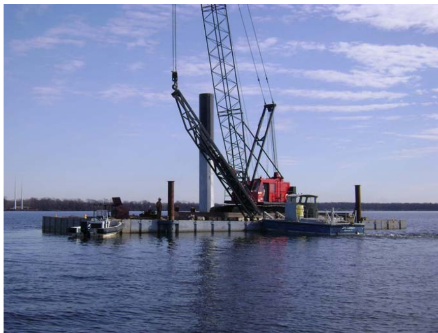
Figure 4 - Barge and Hammer in Position to Drive Caisson
