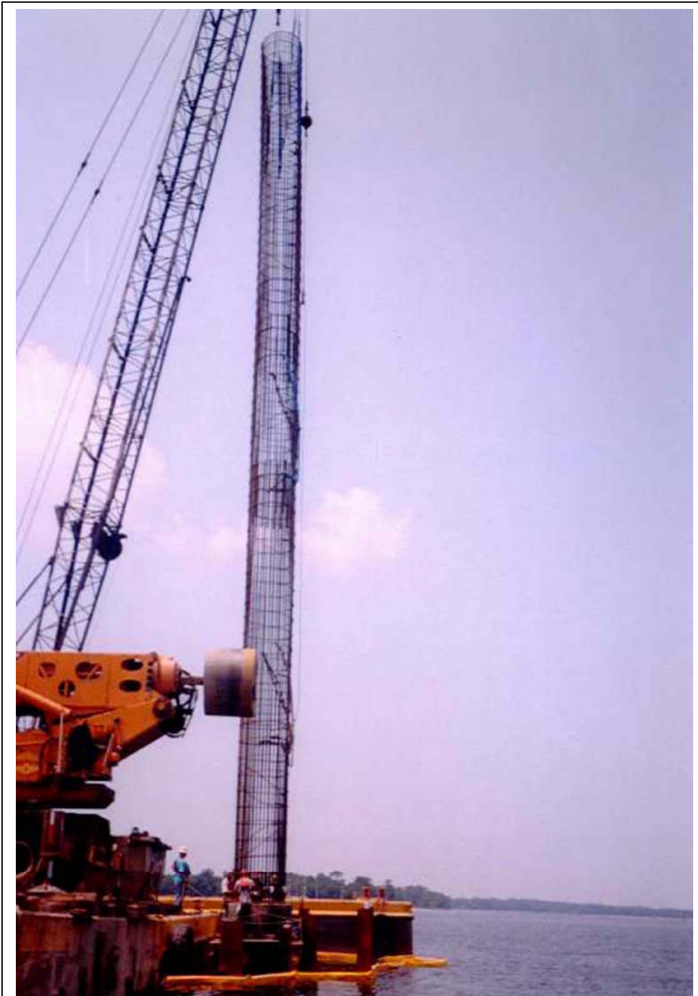
Figure 5. Reinforcement Bar Cage Placed Inside Caisson
