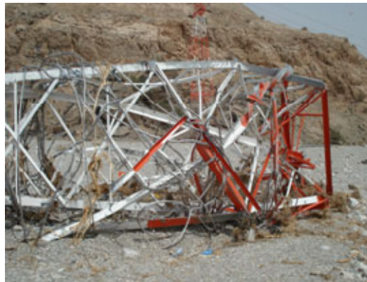
Exhibit No. 7: Damaged tower
