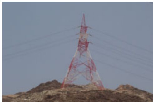
Exhibit No. 21: New Transmission line diverted on the hill
