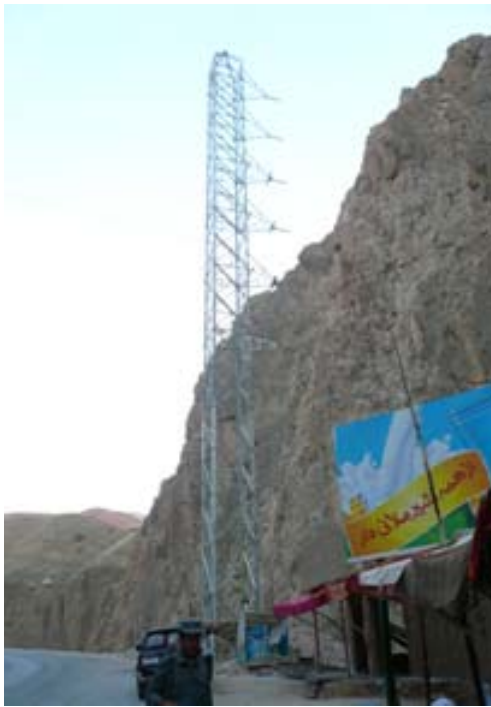
Exhibit No.10: Fully erected tower
