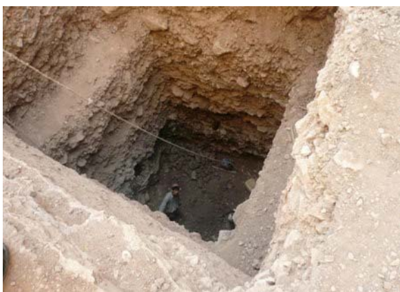
Exhibit No.4: Foundation excavation
