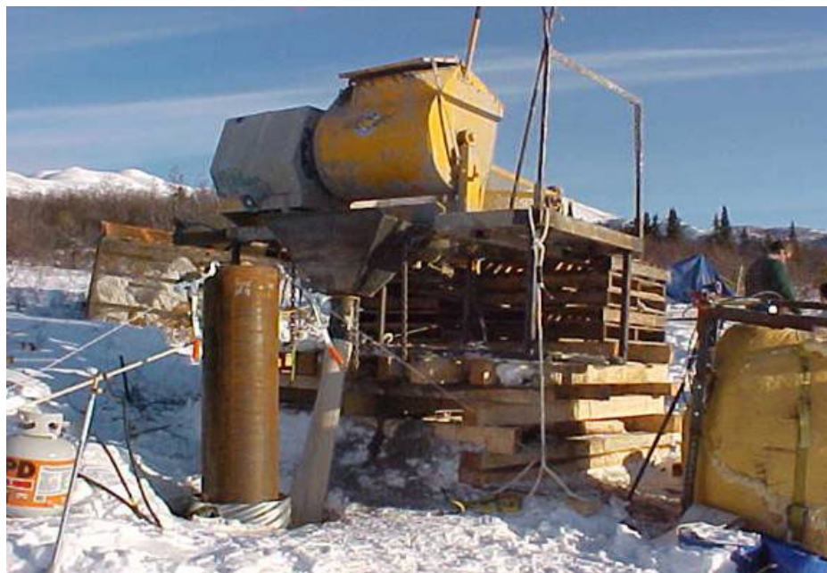
Fig. 3a (top) Work Pad Cribbing on sideslope. Fig. 3b (bottom) Foundation pile grouting setup on cribbing.
