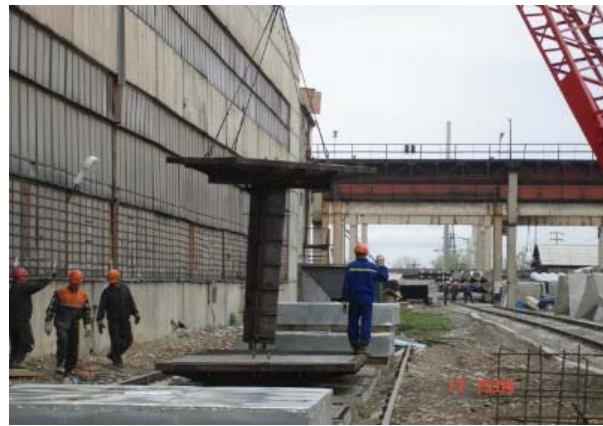
Exhibit No.23: Casting of foundations in factory
