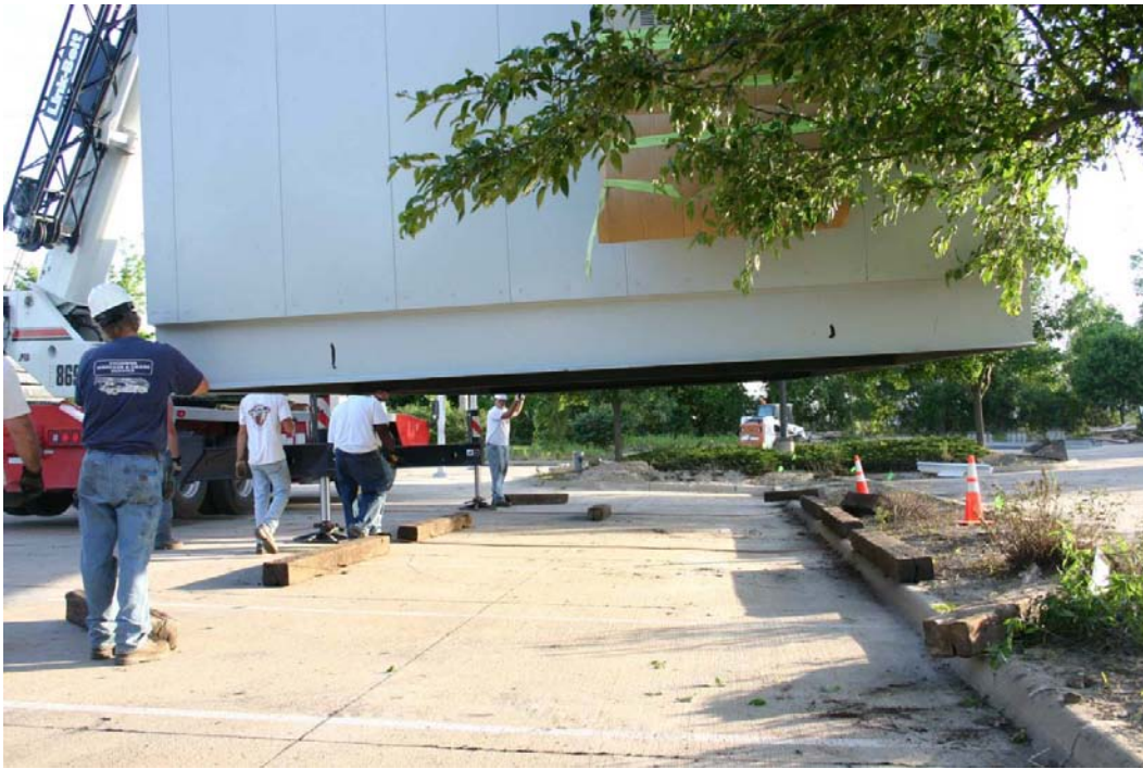
Figure 3 - Setting the 15kV Switchgear on Railroad Ties
