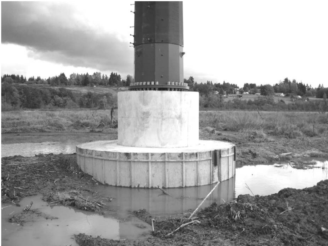
Figure 5 - Ebey Slough Micropile Deadend Foundation
