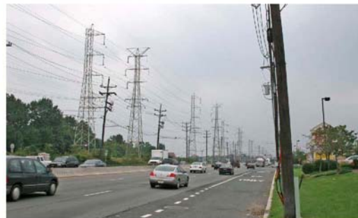
Figure 9: Low visual-quality, linear features (roads) should be paralleled or considered where possible.
