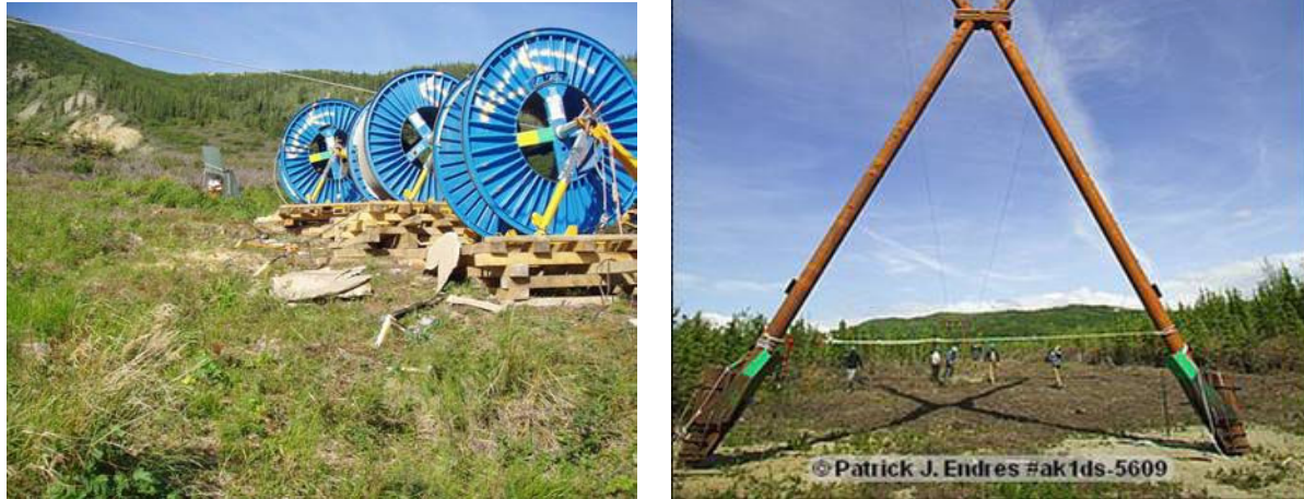
Fig 10a (above left) Wire pulling setup Fig. 10b (above right) Helicopter tower set. (Used with Permission)
