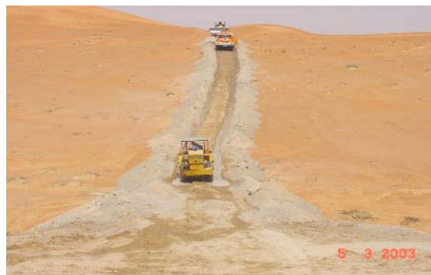
Exhibit No.13: Preparation of Access Road.
