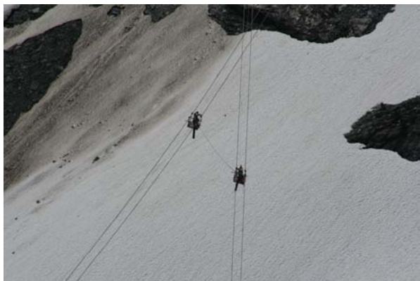
Figure 9 Catwalk sections were flown to the men on the growing catwalk by an A-Star B2.
