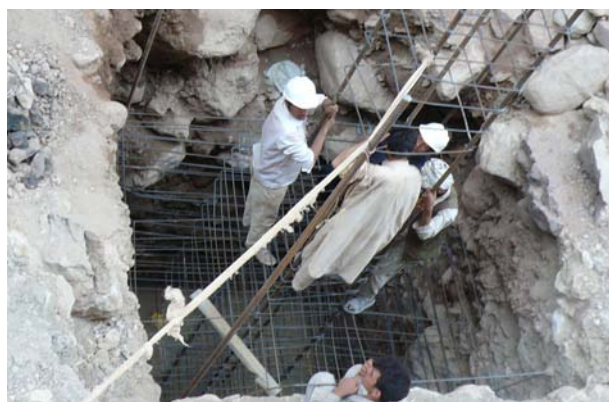
Exhibit No.6: Fixing the reinforcement bars
