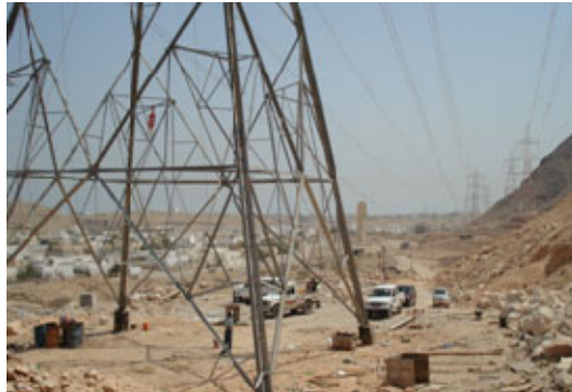
Exhibit No. 18: Construction of the newly designed transmission towers
