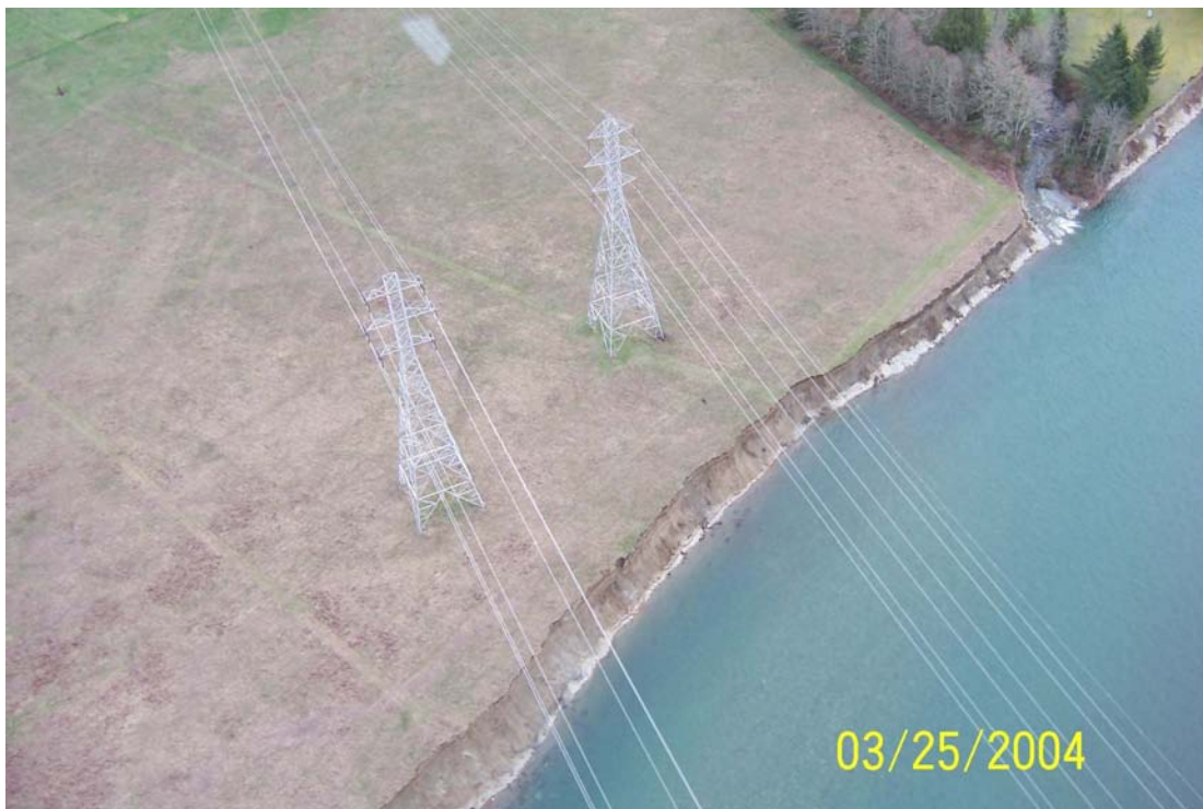
Figure 2. Proximity of 230kv towers to river bank. Photograph by unknown Seattle City Light staff.
