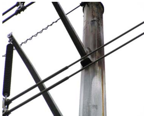
Severe Exterior Corrosion
