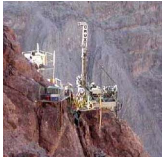
Helicopter positioned limited access rig Figure 7
