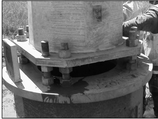
Figure 4 – Typical Baseplate Connection
