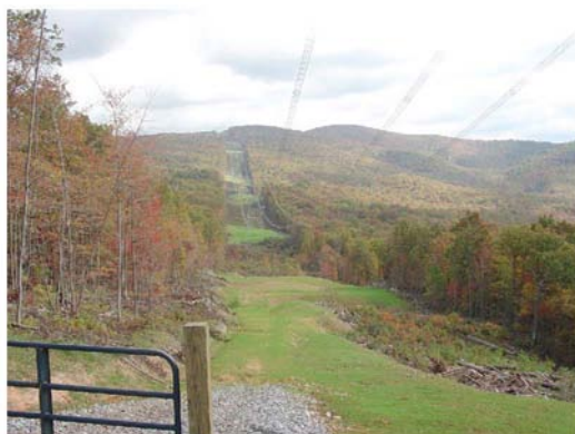
Figure 26: 765kV ROW - Restoration and revegetation
