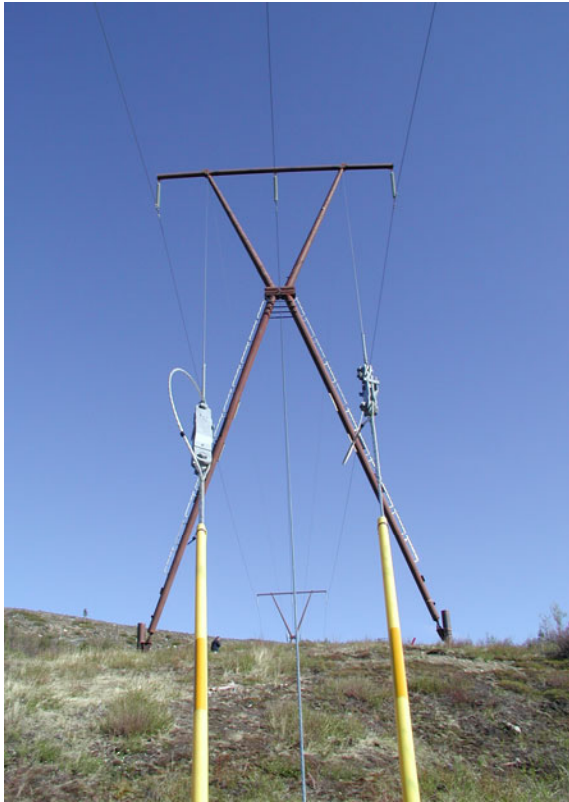
Fig. 8a (left) X-tower with shear release mechanism
