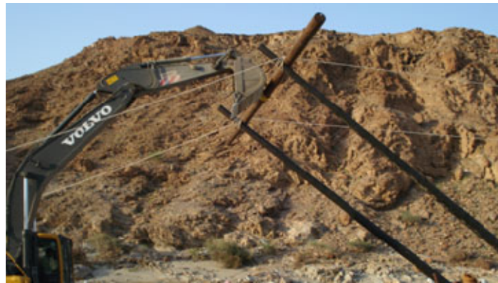
Exhibit No. 12: Erection of the wooden frame.
