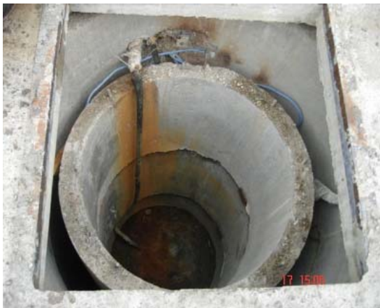
Exhibit No.22: Electric heating system for foundation chimney.
