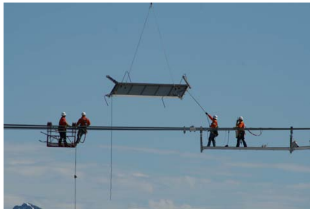
Figure 8 Crews in Carts bundled the small cables into larger cables and rigged the parallel pairs towards each other at yoke plate positions
