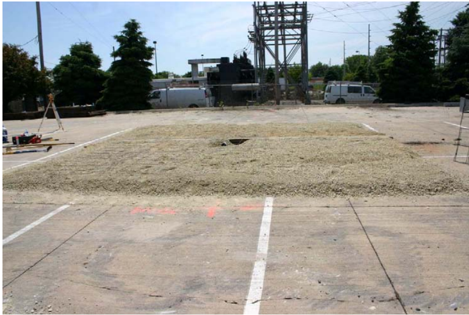
Figure 2 - Road Stone Foundation for the Power Transformer
