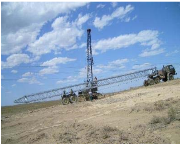
Exhibit No.24: Assembled tower being transported to site
