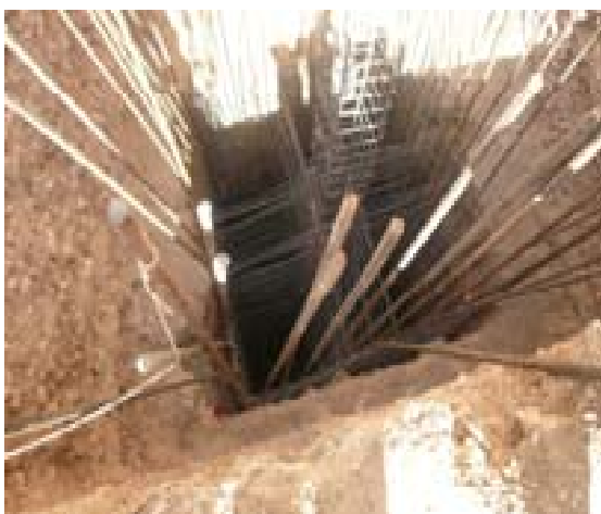
Exhibit No.5: Placing the reinforcement bars
