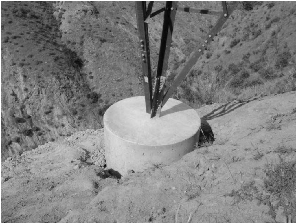
Figure 6 - TRTP Micropile Suspension Tower Leg Foundation
