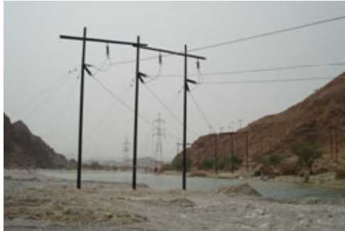
Exhibit No. 17: Emergency line Restoration in 8 days
