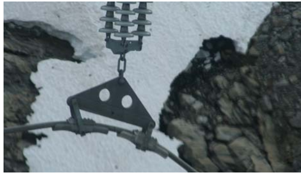
Figure 6 SAPs played a fundamental role in determining the required strap lengths to keep the shoes from interfering with the yoke plate.
