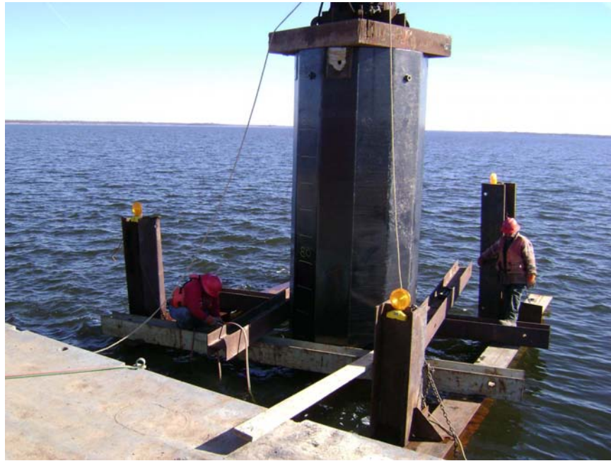
Figure 5 - Pile Caisson in Stabilizer Being Driven by Hammer
