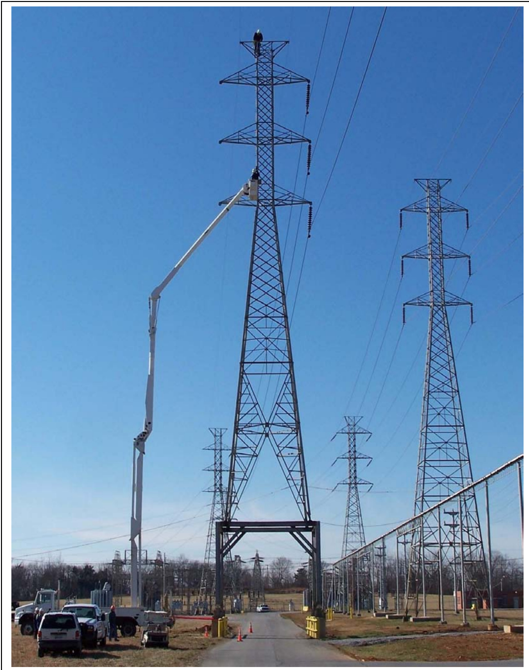
Figure 1. Tangent Tower Supported By A Portal Frame (Linemen taking dimensions, individual member sizes, and connection configuration on this energized tower)
