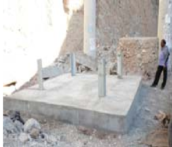
Exhibit No.9: Block foundation with stubs
