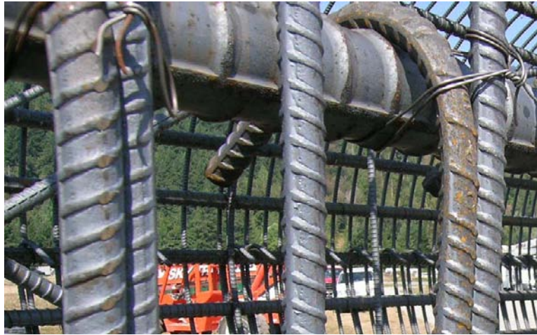
Figure 3: End of hoops turned into the core.
