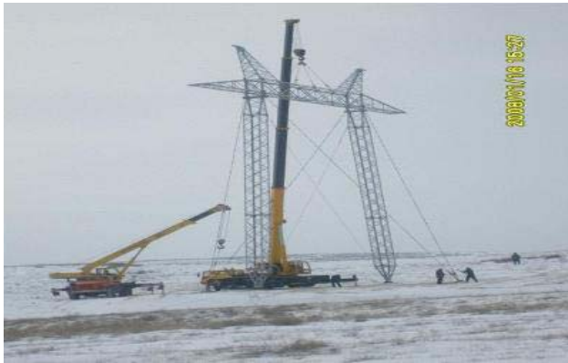
Exhibit No.26: Erection by crane
