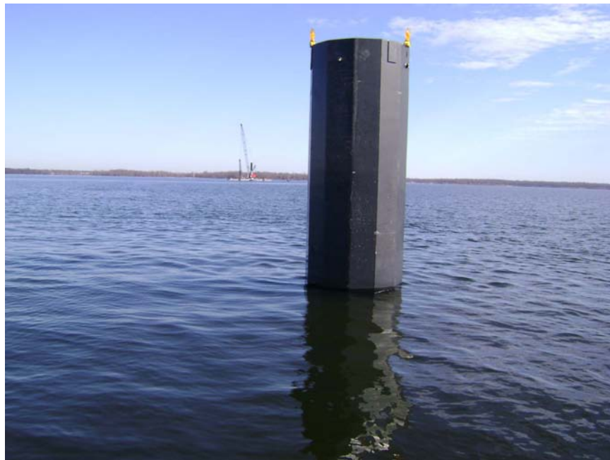
Figure 6 - Installed Caisson Ready to Accept Single Pole Structure
