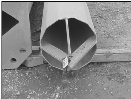
Figure 3 – Typical Slip Alignment Guide
