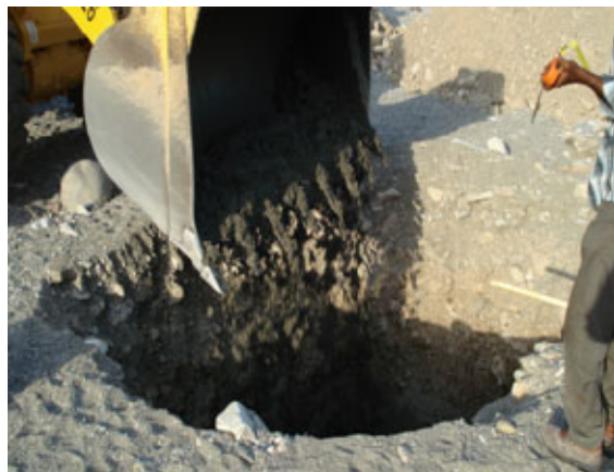
Exhibit No. 15: Excavating the soil
