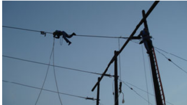
Exhibit No. 14: Stringing the conductors
