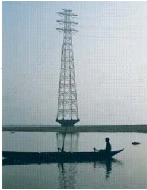
Exhibit No. 35: Brahmaputra River crossing tower
