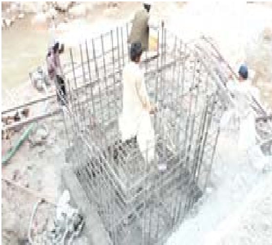
Exhibit No.8: Foundation in progress
