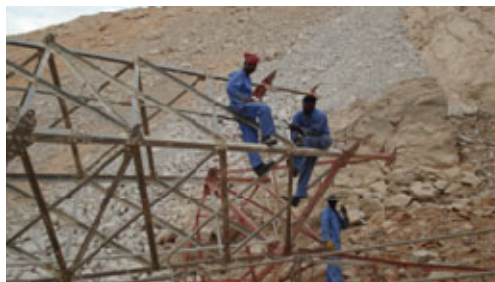
Exhibit No. 19: Erection of the new transmission towers
