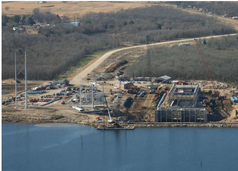
Figure 3 - West Shore Pumping Station and Line Structures
