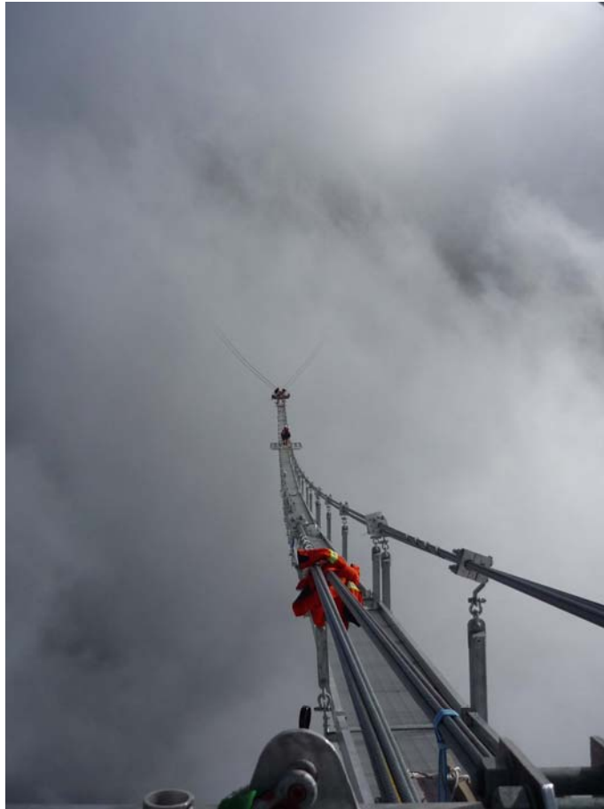
Figure 10 The nearly complete Catenary on a spooky day. The helipad is near the catwalk midpoint and the crew is finalizing the distant yoke plate assembly.
