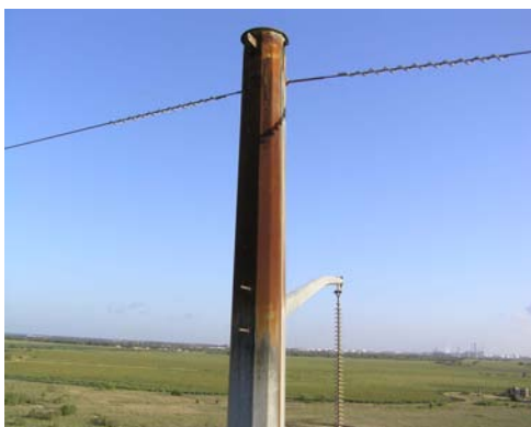
Severe Exterior Corrosion
