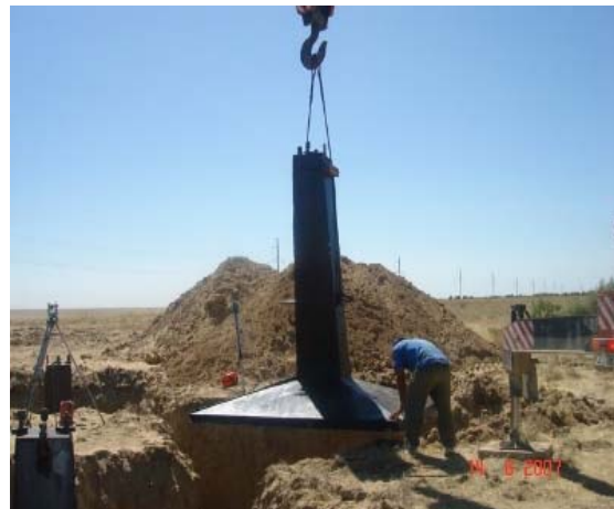
Exhibit No.25: Precast foundation being lowered into excavated pit
