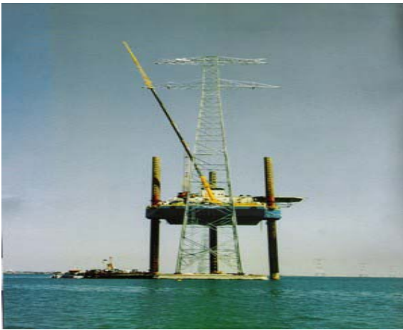
Exhibit No.17: Erection of tower in Arabian Sea
