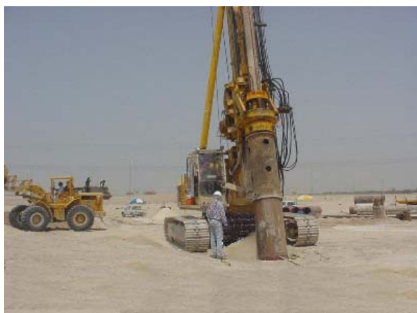
Exhibit No.14: Driving battered pile
