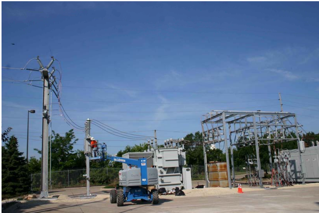
Figure 5 - Cedar Temporary Substation nearing completion
