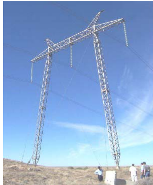
Exhibit No.27: 500 kV S/C complete and energized
