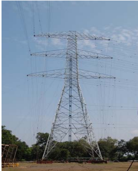
Exhibit No. 16: 400 kV quad multi circuit undergoing prototype testing
