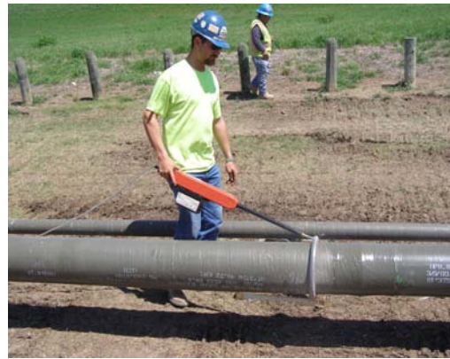
Figure 5. 2 kV "jeep" testing of coated pipe. Searching for voids in coating
