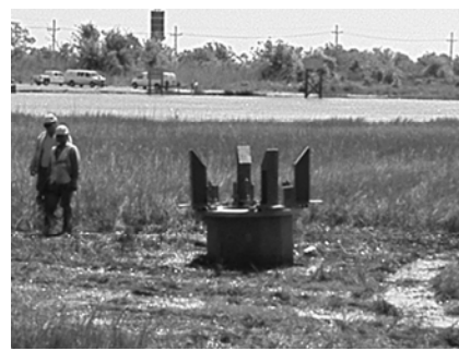
Figure 8a – Pole Guides
