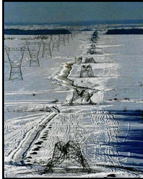
Figure 5 Loss of a 735 kV Line in Quebec (1998 Ice Storm)
