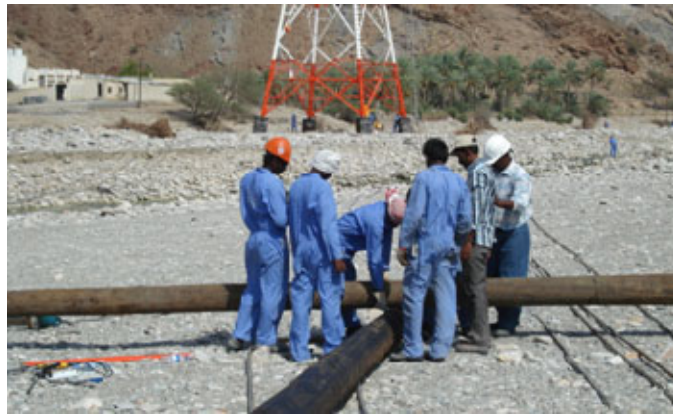
Exhibit No. 11: Unique solution for immediate Restoration of power by using wooden frame
