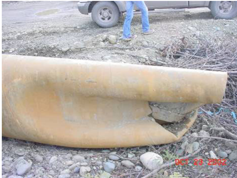
Fig. 9 One of several pile damaged during installation
