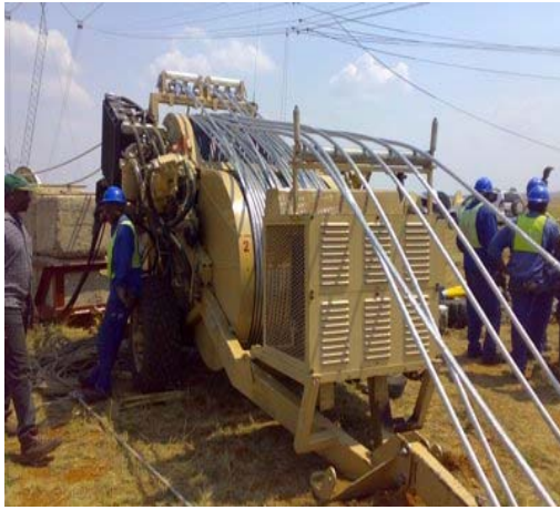
Exhibit No.29: Stringing machine for pulling six conductor bundle.
