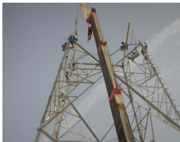
Exhibit No. 15: Erection by crane
