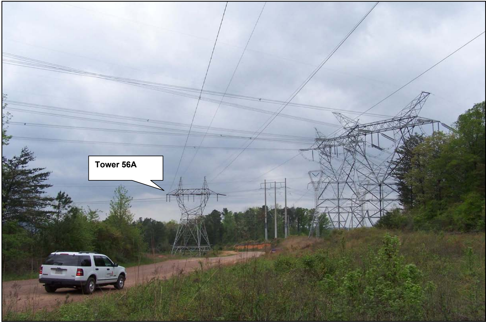
Figure 4: Conductor in Span A crossing (2) 500 kV transmission lines and a roadway
