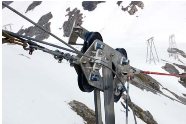
Figure 7 A pulling trolley pulled all cables but the first, on which it rode. We put 40 miles on this rig making 26 round trips.
