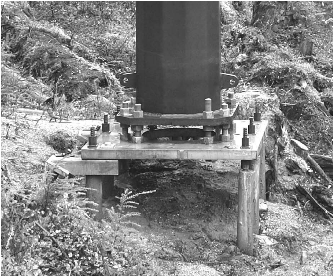
Figure 2 - Swan-Tyee Intertie Micropile Foundation
