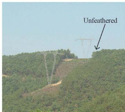
Figure 24: The 765kV ROW before feathering mitigation.
