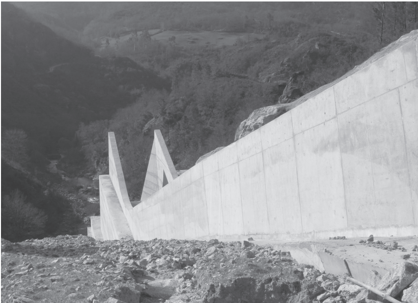
Figure 5.8 Paradela Dam (Portugal) spillway including a narrow flip bucket (Layout 2) downstream of a long chute (Photo Michael Pfister).
