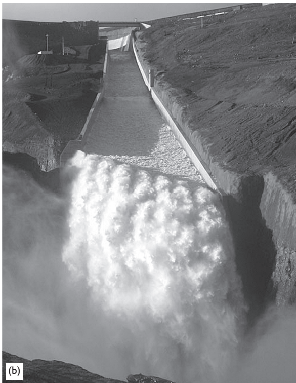
Figure 5.7 Chute end of Kárahnjúkar Dam spillway (Iceland, plain end-overfall with oblique take-off lip equipped with baffles) with (a) roll-waves initiated by small a discharge, and (b) in operation with a discharge of some 300 \text{ m}^3/\text{s} (Photos Landsvirkjun, Iceland).
