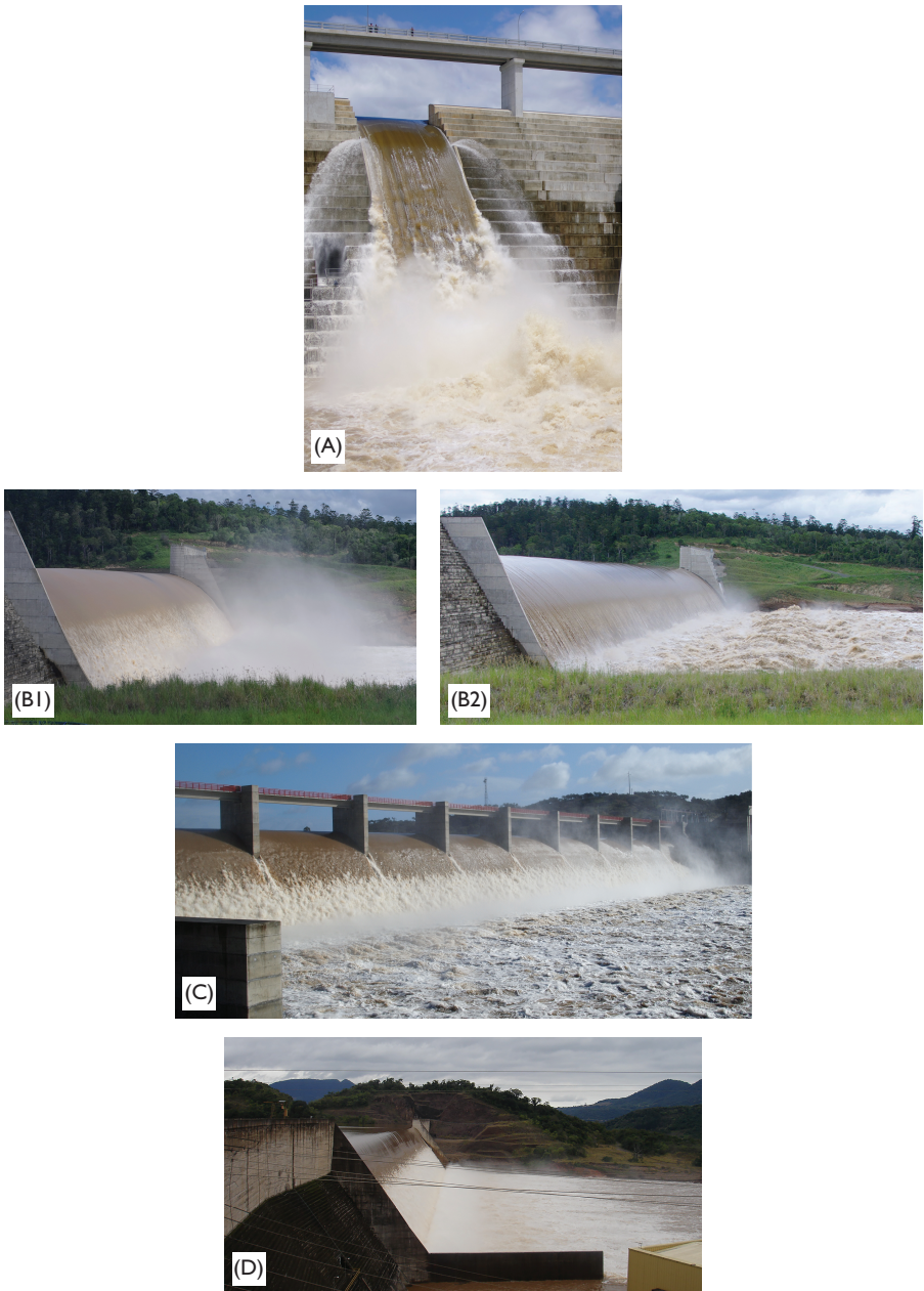
Figure 3.10 Prototype stepped spillway operations. (A) Hinze dam spillway ( \theta=51.3^\circ , h = 1.2 m, Q = 200 m 3 /s, d_s/h = 2.5 on 29 Jan. 2013). (B1) Paradise dam spillway ( \theta = 57.4^\circ , h = 0.62 m, Q = 2,320 m 3 /s, d_s/h = 2.85 on 5 Mar. 2013). (B2) Paradise dam spillway ( \theta = 57.4^\circ , h = 0.62 m, Q = 6,000 m 3 /s, d_s/h = 5.4 on 30 Dec. 2010). (C) Pedrógão dam ( \theta = 53.1^\circ , h = 0.6 m, on 10 Jan. 2010) (Courtesy of EDIA). (D) Dona Francisca dam ( \theta = 53.1^\circ , h = 0.6 m, in July 2011) (Courtesy of Marcelo Marques).
