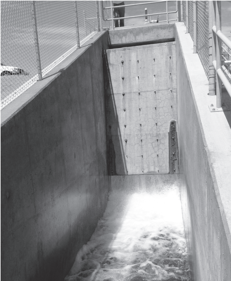
Figure 6.8 Modified hanging baffle dissipator in Arizona, USA. The hanging baffle is slightly angled away from the incoming jet. The bolts that anchor the steel plating can be seen. The increased drop height of the dissipator was a site constraint.
