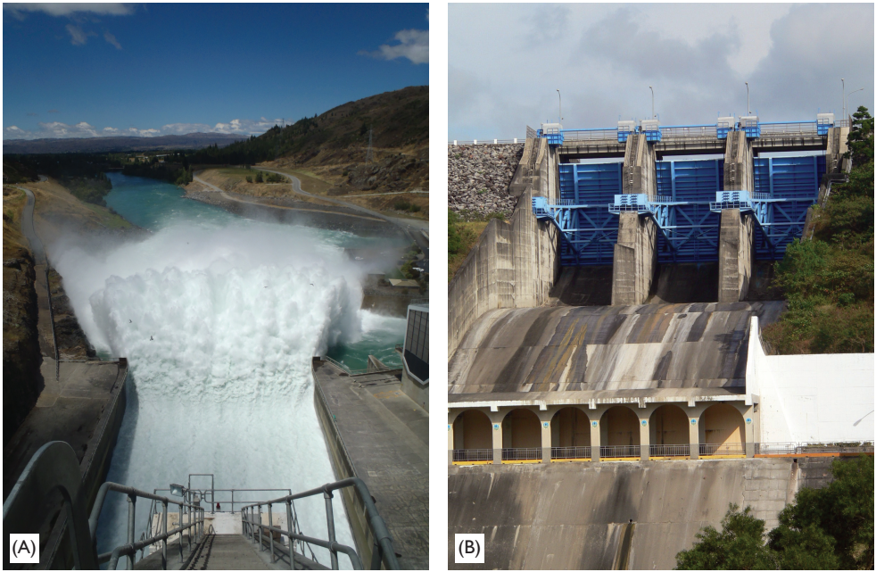
Figure 1.4 Flip bucket spillway systems. (A) Clyde dam spillway (New Zealand) (Courtesy of Graham Quinn & Contact Energy). (B) Mudan dam spillway (Taiwan) on 21 November 2006.
