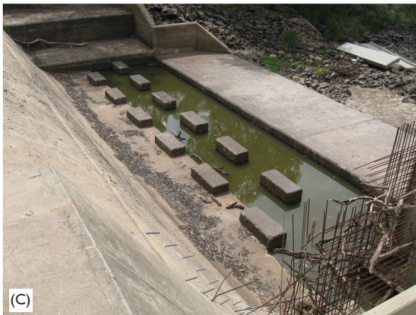
Figure 4.14 Photographs of hydraulic jump stilling basins (A) Hinze dam spillway stage 3 (Australia) on 25 April 2013 (Courtesy of Davide Wüthrich): the stilling basin was designed based upon a physical study and each block is 3.2 m high. (B) Stilling basin in Jeju Island (Korea): on 26 May 2013 at low tide and on 28 May 2013 after a storm. (C) Loundoun weir stilling basin (Australia) on 16 January 2009 (Courtesy of Damien Roman).
