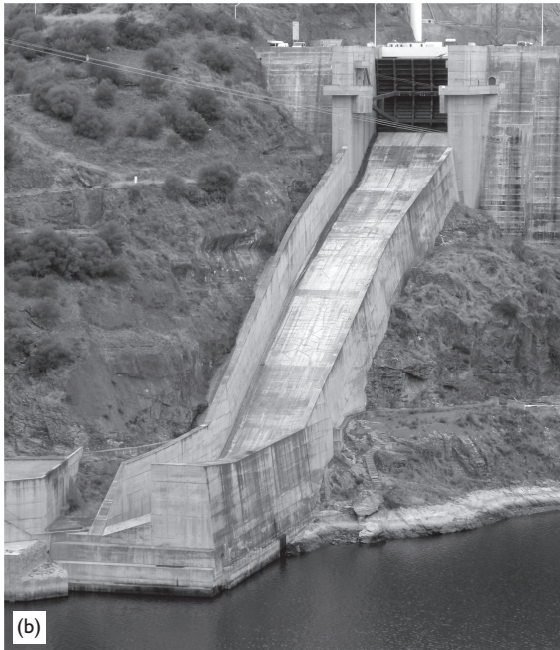
Figure 5.6 Alqueva Dam (Portugal) spillway with (a) an insert at the take-off lip (left spillway, bucket Type 5), and (b) a vertical deflector on the bucket of the right spillway (Layout 4, both Photos Michael Pfister).
