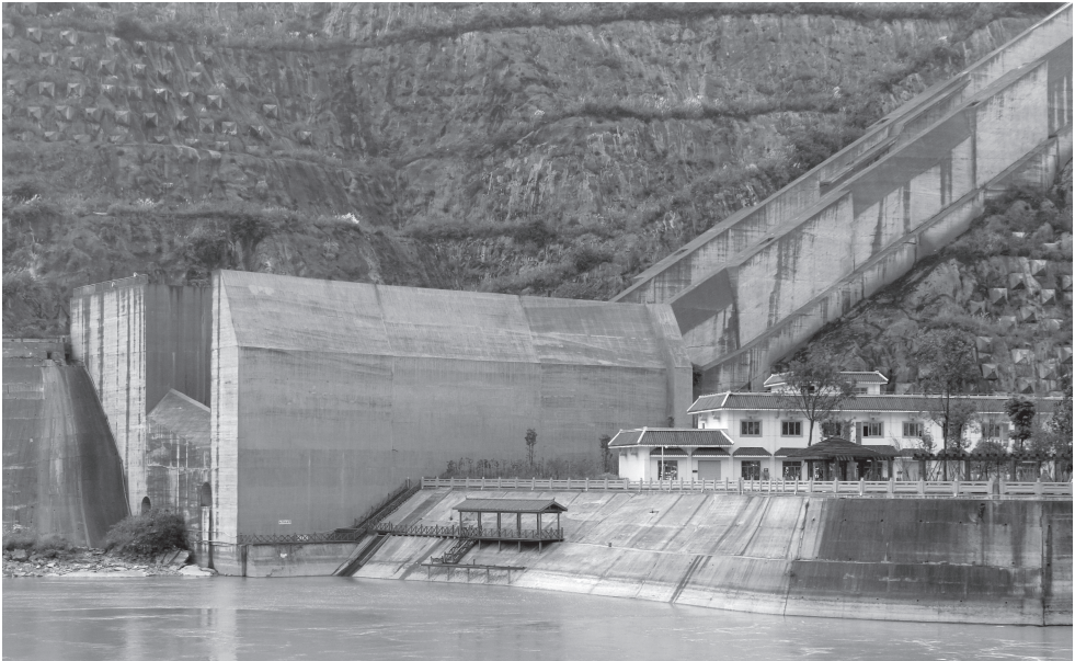
Figure 5.5 Principal spillway of Zipingpu Dam (China) with a bucket Type 2 (Photo Michael Pfister).
