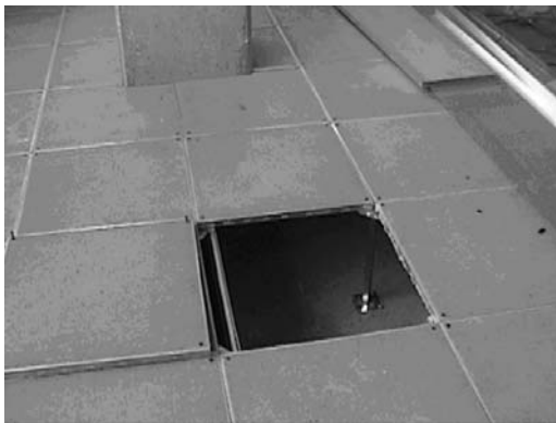
Figure 4.27 Image of a UFAD installation
