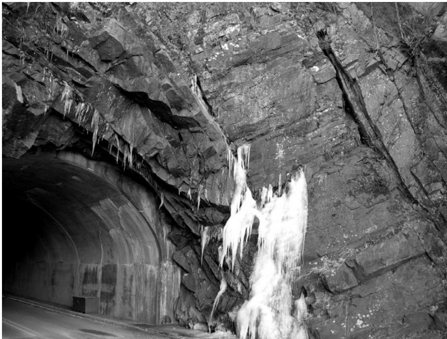
FIGURE 2-8 Tunnel and road cut in Paleozoic metamorphic rocks 5 mi south of the entrance to the Shenandoah National Park at Route 211 and the Skyline Drive near Sperryville, Virginia. The water flowing out of the fractures in the fault zone is frozen.
