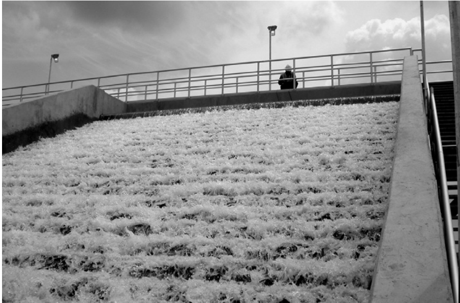
FIGURE 10.9-12 Twin Oaks aerator. (Copyright Gregg Eckhardt, printed with permission.)
