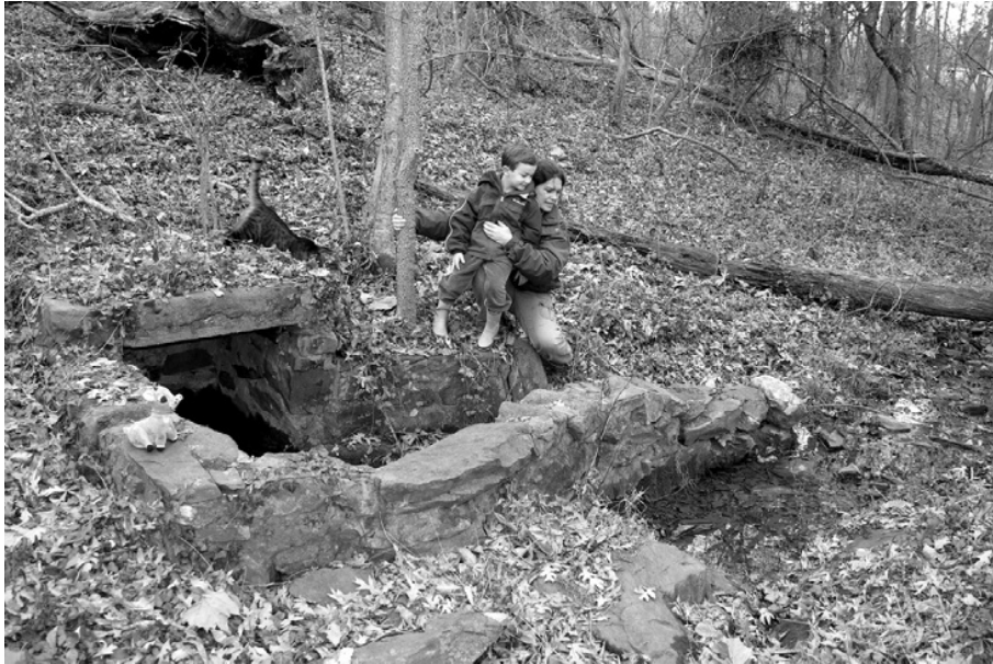
FIGURE 2-10 Simple capture of a small spring issuing from fractures in Paleozoic metamorphic rocks of the Piedmont physiographic province, the United States. This spring was tapped before the Civil War for the water supply of a farmhouse in Virginia. Many other similar springs are still used as sources of both potable and nonpotable water, although drilled wells are now the main form of water supply in the region.
