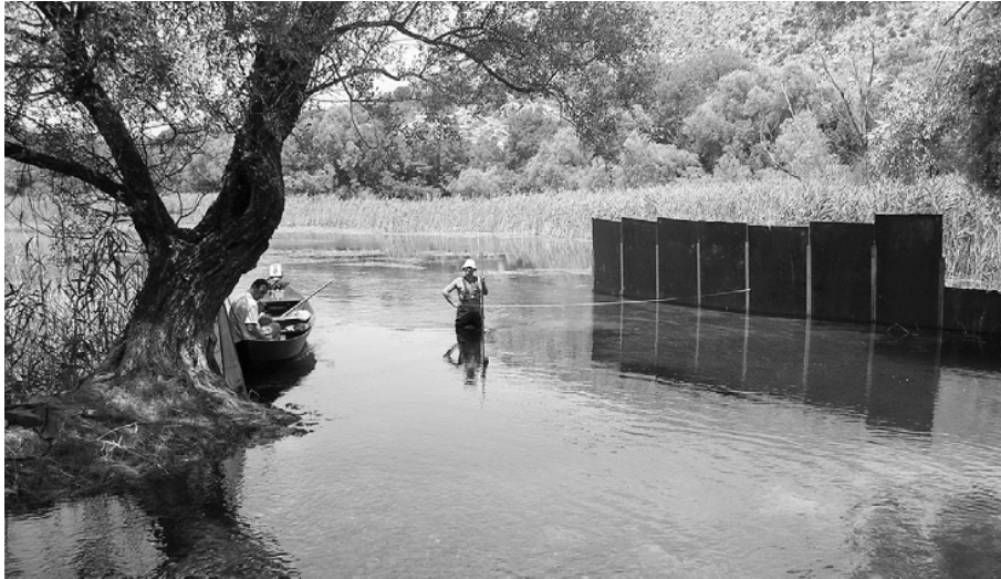
FIGURE 10.5–7 The installed panel system for streaming the flow of Bolje Sestre.
