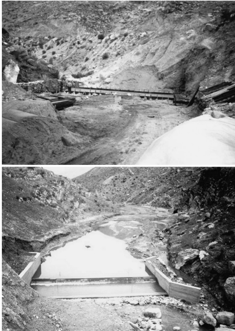
FIGURE 9–8 Subsurface dam Gali Basera in northern Iraq. The goal is to store water coming from numerous smaller springs along the alluvial valley. The stored water is utilized throughout the year and contributes to the recharge of the underlying karstic aquifer. (Top) View from the upstream side, concrete barrier under construction; (bottom) view from downstream, after the construction was completed.
