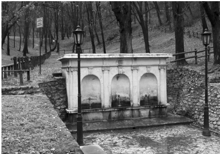
FIGURE 9–24 Spring capture surrounded by wooden fence. The sign on the pole indicates the first sanitary protection zone (Haiduk Spring in Kosutnjak Belgrade, Serbia).
