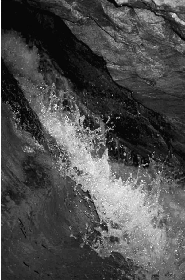
FIGURE 10.2–12 Large Kläffer draining into the gallery of the water main.
