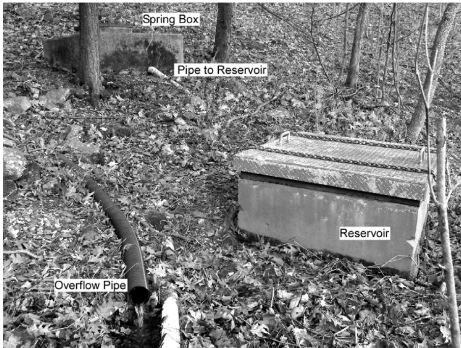
FIGURE 2-9 Capture of a permanent spring issuing from Paleozoic metamorphic rocks and used for the public water supply, Skyline Drive, Virginia.
