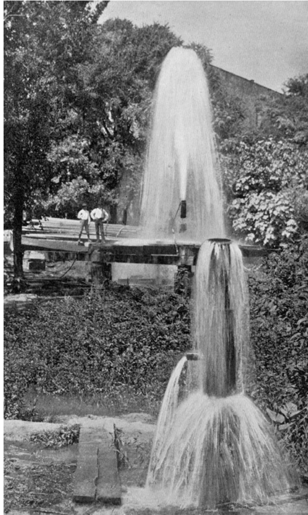
FIGURE 10.9-1 The first large Edwards Aquifer wells, drilled in San Antonio. (From Hill and Vaughan, 1896.)
