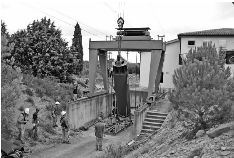
FIGURE 5-27 Replacement of pumps at the Lez Spring. (Photograph courtesy of Jean Michel Valéry.)
