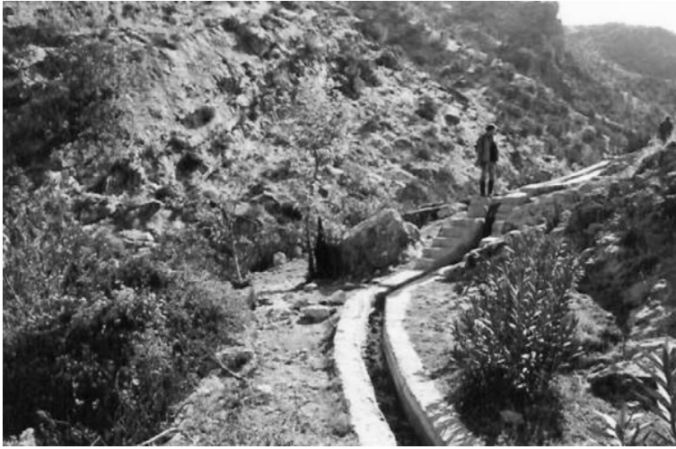
FIGURE 9-6 Typical concrete channel diverting springwater from the mountains toward the plain (Botas, Zakho, northern Iraq).
