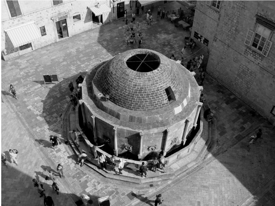
FIGURE 1–17 Great Fountain of Onofria in Dubrovnik, Croatia, designed and built by the Italian architect Onofria della Cave in 1440. Water for the fountain, which includes the water storage reservoir, was conveyed from a group of springs by a 12-km-long system of canals and aqueducts. (Photograph courtesy of Vojislav Ilic.)
