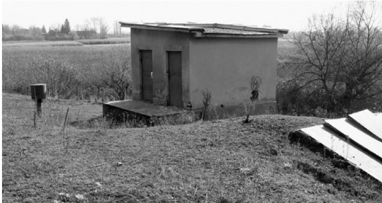
FIGURE 9–23 Maintenance room and reservoir covered by grass with one vent and metal cover entrance, Opicvet Spring near Sofia, Bulgaria.
