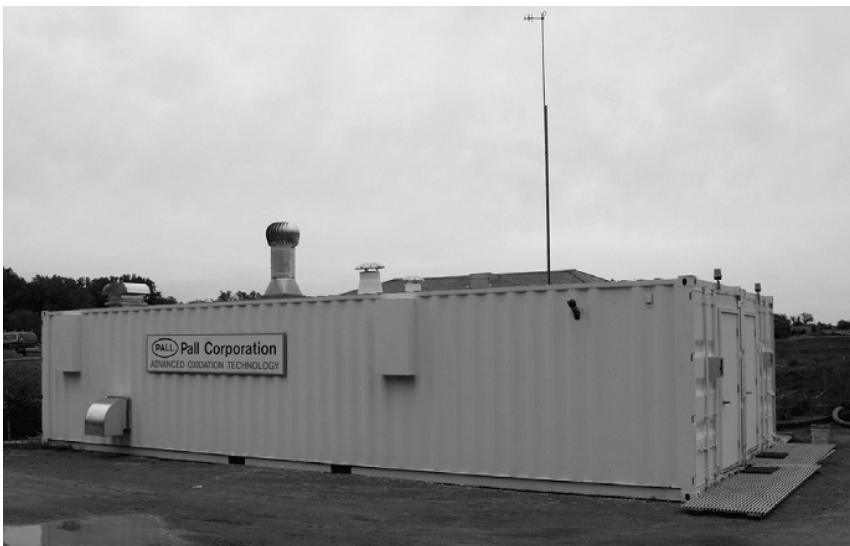
FIGURE 7-13 Mobile field unit for flow rate of 200 gpm. Design and engineering by Farsad Fotouhi, Pall Corporation.
