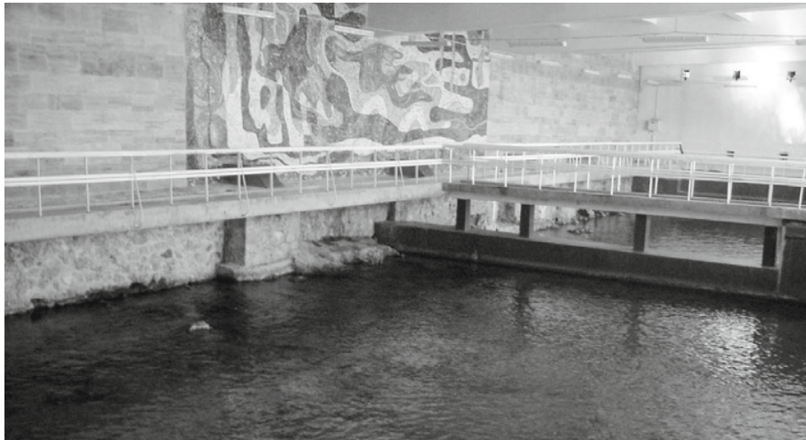
FIGURE 10.4-5 (a) Schematic of the main intake system of the Izvarna Spring (not to scale); (b) main intake basin. (Simplified from Constantinescu, 1980 , and Teodorescu, 1965 .)
