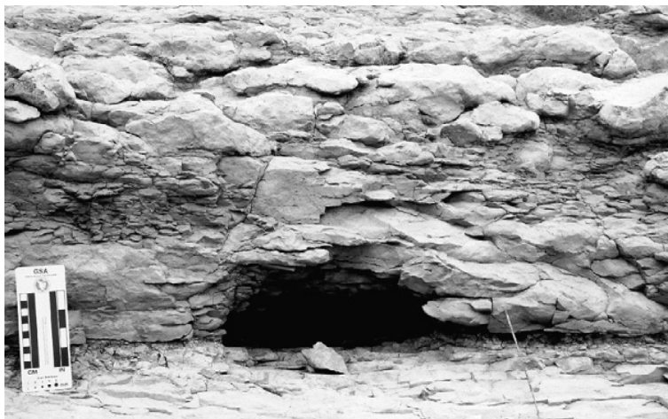
FIGURE 5-44 Small conduit, about 20 cm across, developed in fissured limestone.
