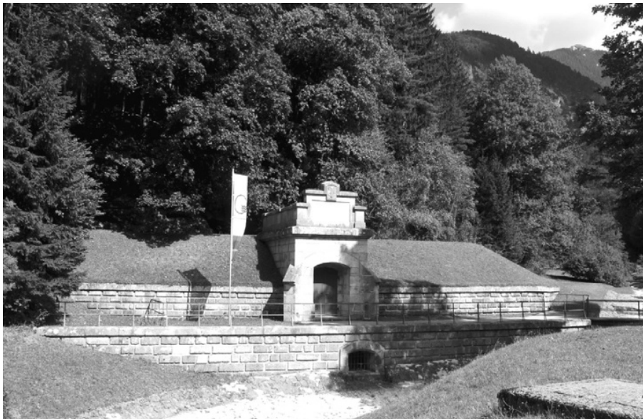
FIGURE 9-22 Kaiserbrunn spring used for the water supply of Vienna since the 19th century. The covered, grassed intake and reservoir are shown together with a large diameter overflow drain below the main entrance.
