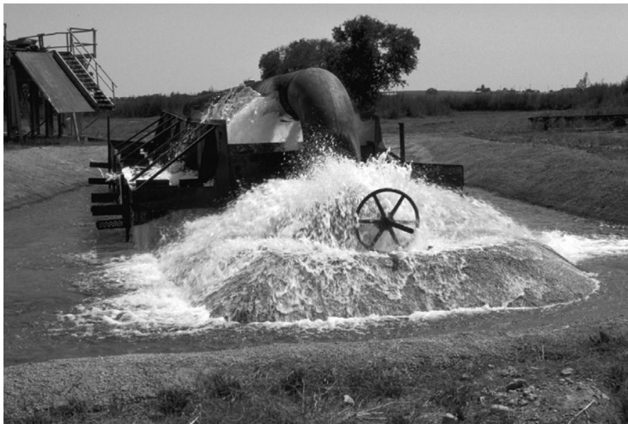
FIGURE 10.9-8 The world's largest water well drilled by Ronnie Pucek. The well, capable of producing more than 50 million gallons per day, was used for a catfish farm near San Antonio. (Copyright Gregg Eckhardt, printed with permission.)
