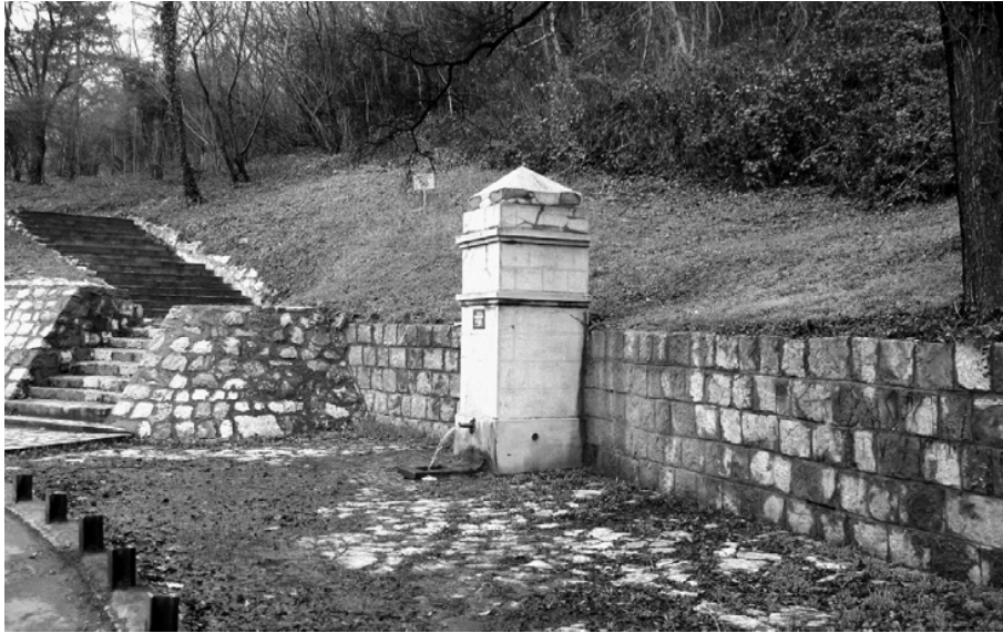
FIGURE 9-21 Long retention wall behind the spring capture, Topcider Spring, Belgrade, Serbia.
