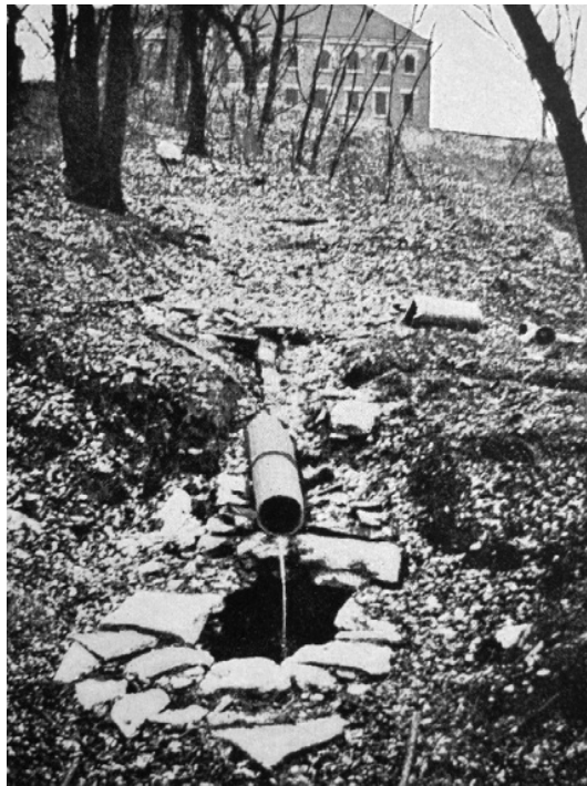
FIGURE 2-43 Continuous stream of sewage from a college building discharging into a sink from which it finds its way to the underground water channels. Photograph used to illustrate vulnerability of groundwater to contamination in an early USGS publication for public education. (From Fuller, 1910 .)
