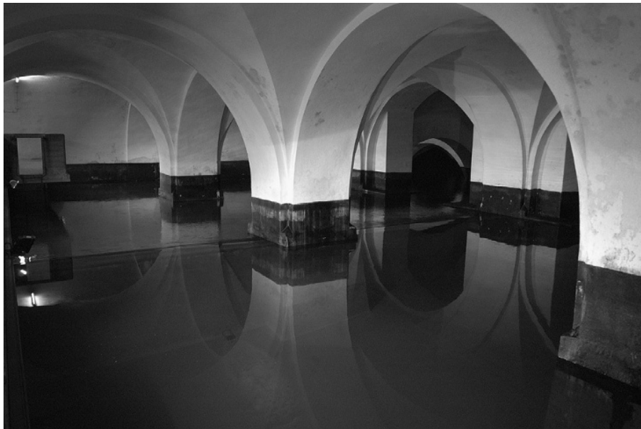
FIGURE 10.2–11 Reservoir at Vienna Rosenhügel with a volume of 120,500 \text{m}^3 .
