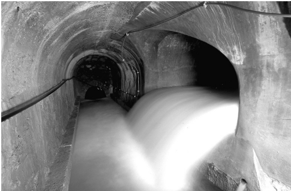
FIGURE 10.2-14 Partly flooded overflow gallery, the Kläffer Spring.
