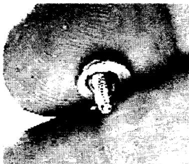
**Plate 17** *This Safety Earth Ground fixing is a 'ring type' – which is good – but the fixing screw is much too small to provide a reliable connection*
