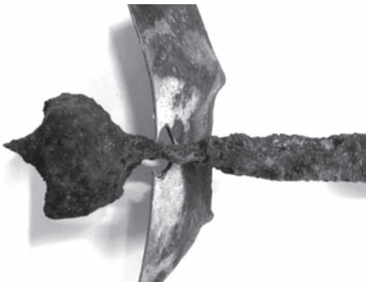
Figure 7: Deterioration of iron bolt caused by contact with copper sheet.
