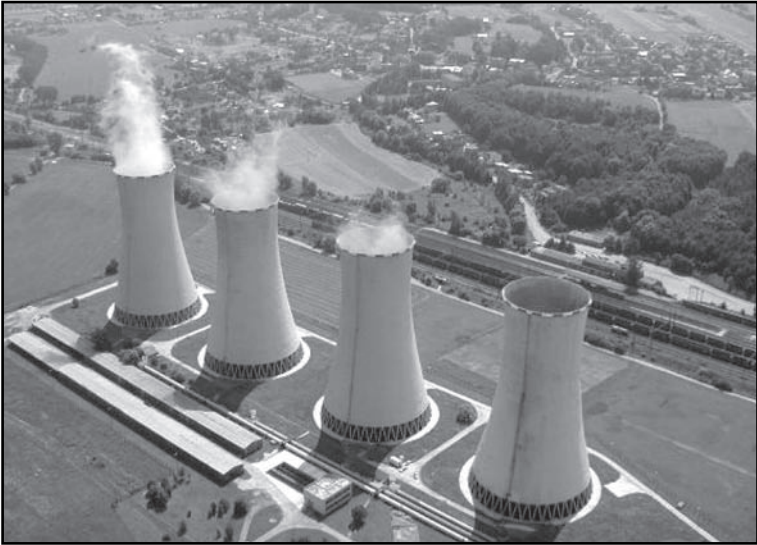
Figure 18: General view of four typically repaired draft cooling towers of the Ittersen type; the structures and the interior equipment of the towers are supported by concrete columns (Photo: J. Bydzovsky).
