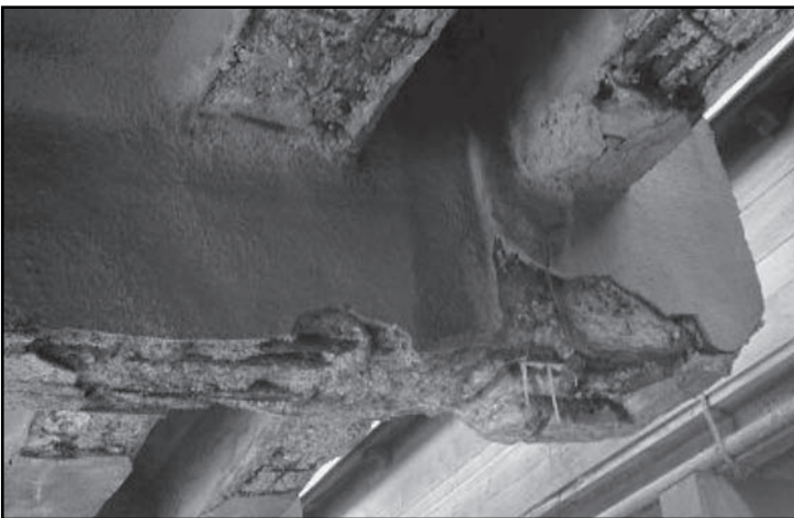
Figure 14: View of the horizontal elements of concrete skeleton monolithic hall in the chromium section of the production plant (Photo: J. Bydovsky).
