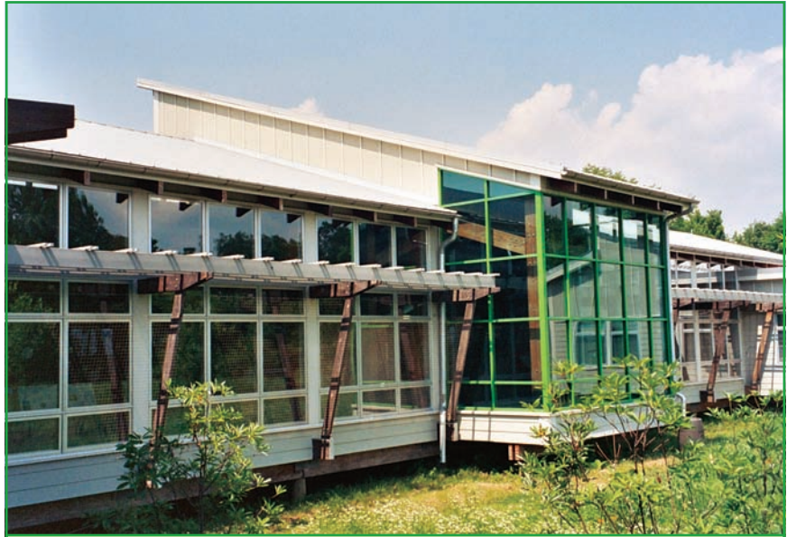
Passive solar homes use sunlight for natural lighting and heat. This house in Pennsylvania uses horizontal light shelves to reflect light into the rooms' interiors. The solarium that extends beyond the outer wall receives sunlight and reflects it. This serves the purpose of lighting the interior and providing heat. ( Cusano Environmental Education Center, John Heinz National Wildlife Refuge at Tinicum )
