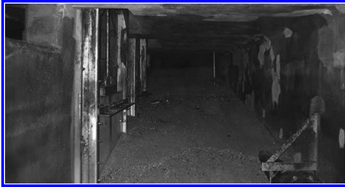
Figure 2. Sand accumulation upstream of the channel weir. The overflow weir can be seen on the left.
