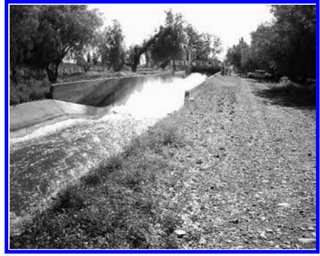
Figure 3. View of the partition structure from upstream.
