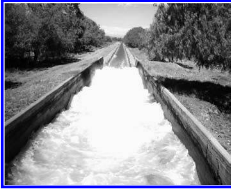
Figure 2. Upstream view from the partition structure.
