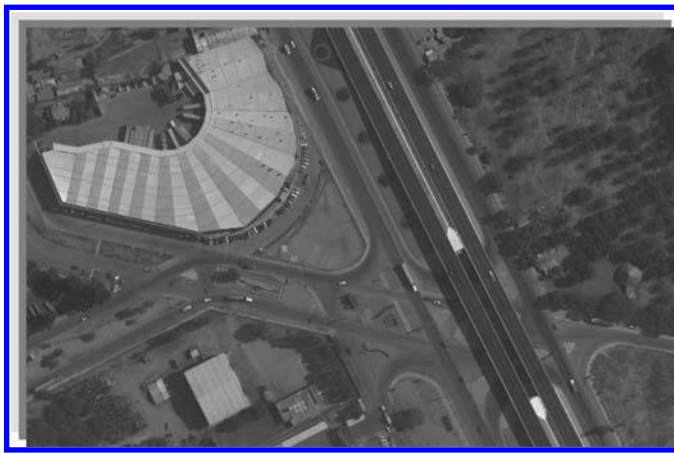
Figure 5. Highway and bridges in San Luis Potosí Industrial Zone (Mexico).
