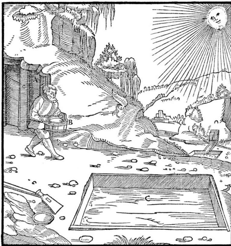
Fig. 10 Vitriol boiling (Agricola, De re metallica (1556))
