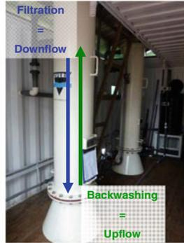
Picture 8: Flow direction during filtration and backwashing
