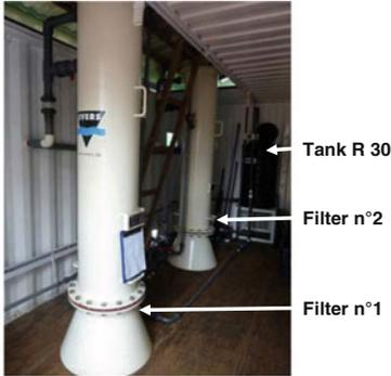
Picture 7: Filtration units inside the container (01/03/2010)
