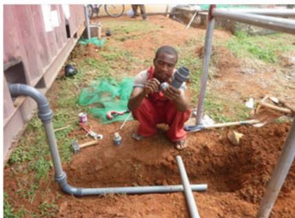
Picture 85: Plumber installing the pipes connecting the filtrations units to the overhead tank (11/02/2010)
