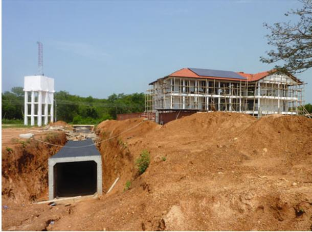
**Fig. 4.39** Large underground rainwater tanks at the Baobab Center
