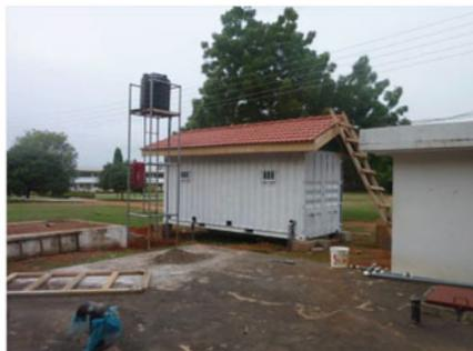
Picture 88: First white coat of paint applied on the outside walls of the container (12/02/2010)
