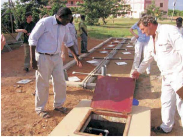
**Fig. 4.53** Sand filter for decentralized wastewater recycling
