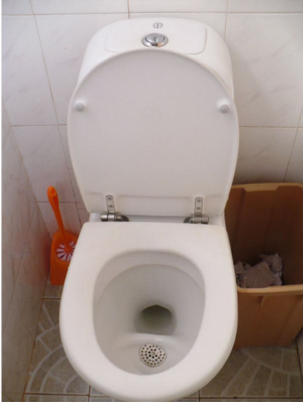
**Fig. 4.37** Low-flush toilets with urine separator (5 instead of 10 L)
