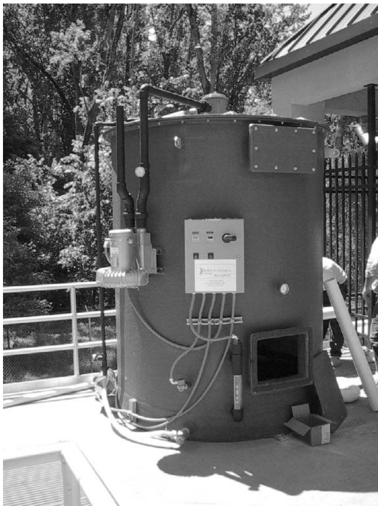
Fig. 15.4. BioReaction Industries single Apollo S200 biofilter system. (Photograph courtesy of BioReaction Industries, Tualatin, OR)
