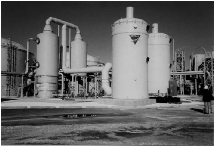
Fig.16.3. Bioreactors (right) treating odorous air from the strippers (left) at a brewery
