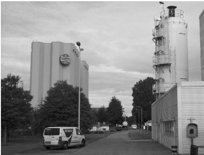
Fig. 16.1. Bioreactor treating odorous air from an anaerobic wastewater treatment plant
