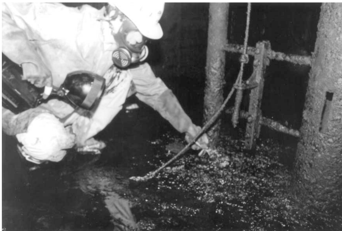
Figure 6 Cleaning sludge, including microbial biomass, from the inside of a contaminated fuel storage tank. (Picture printed with the permission of Howard Chesneau, Fuel Quality Services, Flowery Branch, Georgia, U.S.)
