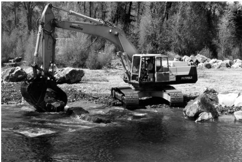
FIGURE 6.30 Contractor adjusting the boulder size and position while constructing a cross-vane in Colorado.
