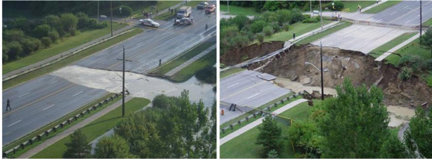
**Fig. 1.11** A caved-in culvert at Finch and Sentinel in the north of the city during the 2005 flooding
