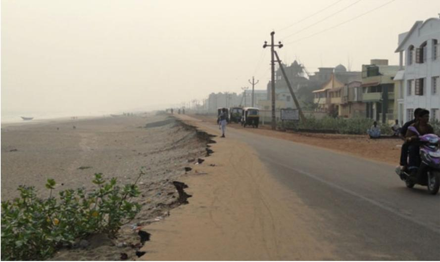
**Fig. 3.28** Storm surges not only cause loss of life but could also significantly damage the coastal infrastructure, as can be seen from this damaged coastal road
