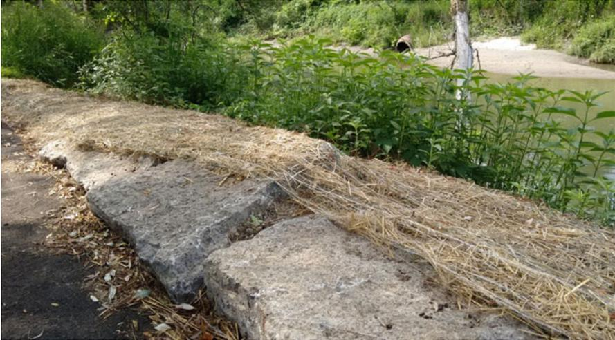
**Fig. 2.2** A quick fix to control erosion – a wire mesh mixed with hay around the slope (Photo by author)
