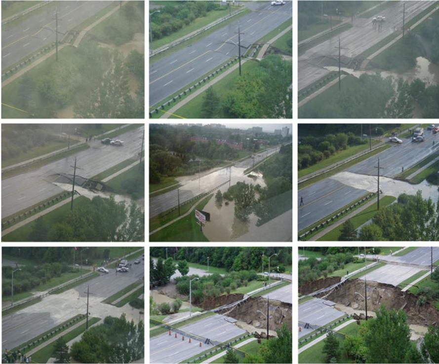
**Fig. 2.16** A section of the road caved in within a matter of hours near Finch and Sentinel in Toronto, near York University on August 19, 2005
