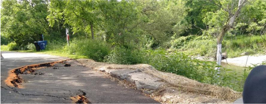
**Fig. 2.1** An example of erosion and subsidence along the Lower Don River in Toronto, Canada (Photo by author)
