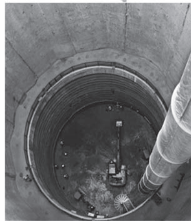
Figure 2. Construction process and lining of shafts (Contreras et al. , 2010).
