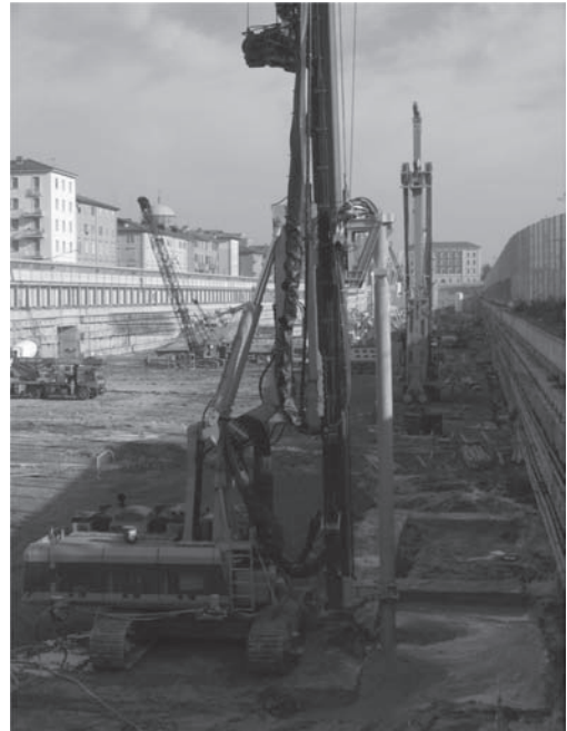
Figure 12. Soil improvement, Bologna, Italy.
