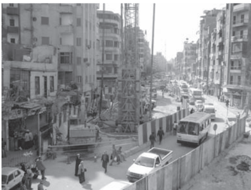
Figure 8. Production during half side diverted traffic.
