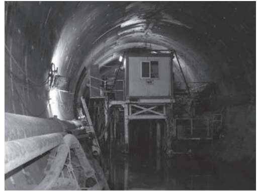
Figure 10. Backup trailers from the tunnel.
