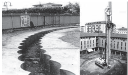
Figure 7. Guide walls and SoilMec equipment for CSP retaining wall construction.
