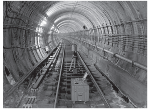
Figure 9. Laser scanner Leica HDS3000 in the Prague metro tunnel close to Mústek station (Pospíšil, J. et al, 2007).
