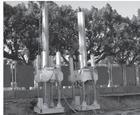
Figure 13. Stop-end extraction by hydraulic jacks.
