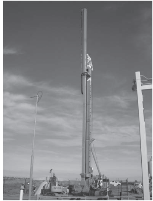
Figure 2. Kelly-guided CSM unit, USA.
