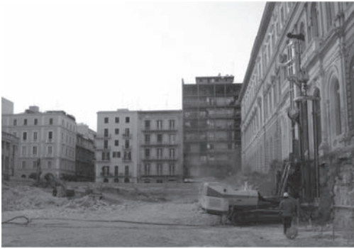
Figure 10. Drilling of the boreholes on the perimeter.
