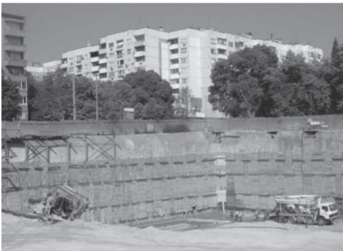
Figure 2. Northern part of the excavation.
