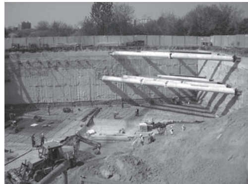
Figure 1. Construction site “Canal+”.
