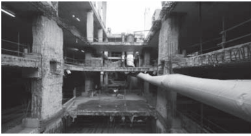
Figure 4. Excavation under third floor slab.
