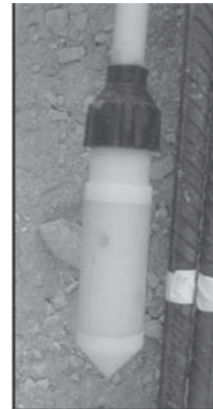
Figure 12. Grouting valve for installation of grout-plug.
