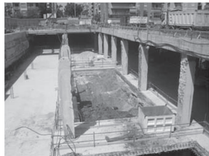
Figure 3. Roof opening and first floor slab.
