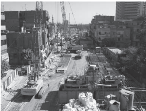
Figure 6. Site installation for cut-off-wall.
