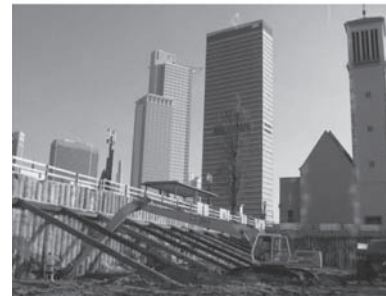
Figure 4. Building pit—cross section subway.
