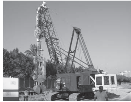
Figure 12. Soilmec BH12 clamshell.
