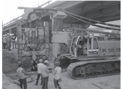
Figure 10. Low head room CBC-cutter under a existing bridge.
