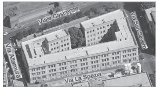
Figure 2. Building involved in this study.
