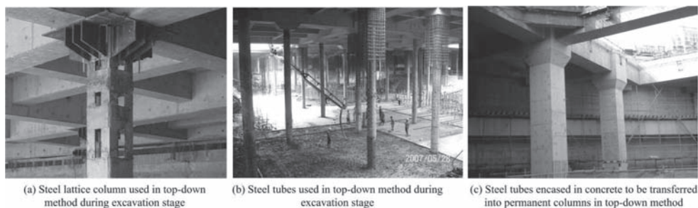
Figure 8. Steel lattice column and steel tubes used in top-down method.
