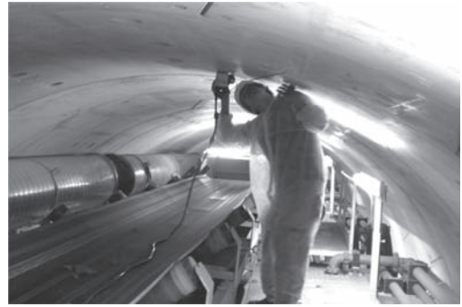
Figure 8. Execution of Georadar Tests above the machine backup.
