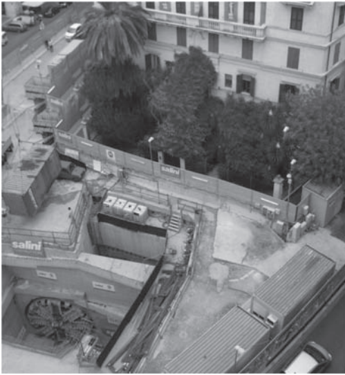
Figure 15. TBM breakthrough at the end of the tunnel, under building 1.
