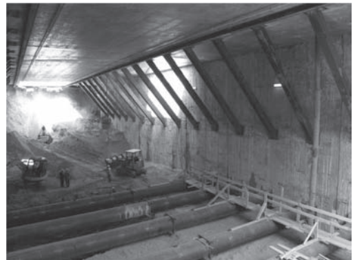
Figure 4. Top down excavation with temporary stiffening.
