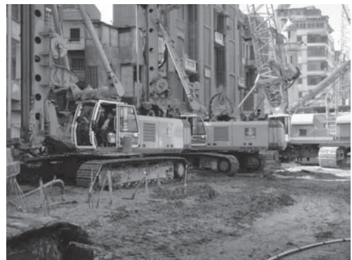
Figure 14. Installation of 60 m deep grouting hole for soft-gel-plug using BG28.
