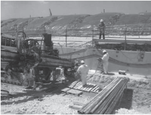
Figure 10. Rigs drilling for grouting.
