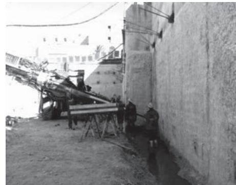
Figure 14. Anchors executions.
