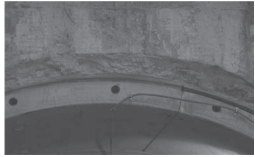
Figure 13. Detail of the tunnel crown in Fig. 12.
