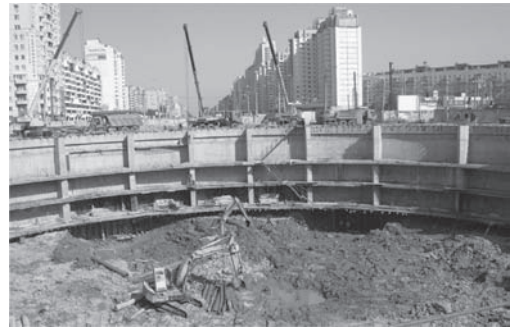
Figure 3. The beams, parts of ceiling and excavation of the ditch level by level.
