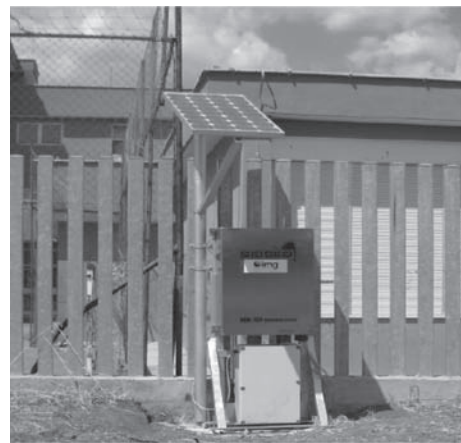
Figure 7. DAU (Data Acquisition Unit).
