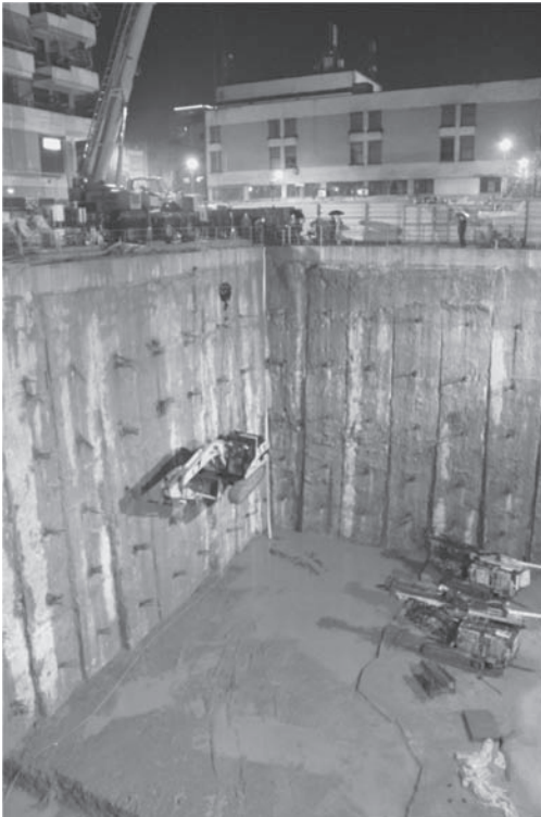
Figure 14. Deep excavation pit with multi anchored diaphragm wall in Tirana.
