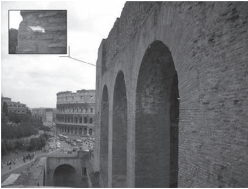
Figure 16. Basilica Maxentius. Particular of geodetic prism.
