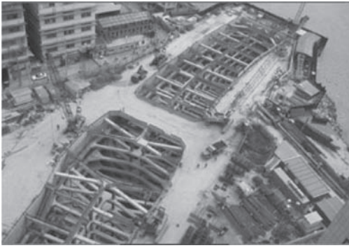
Figure 12. A photo of the construction site (from http://www.51xuewen.com/group/287/topic_11354.htm ).
