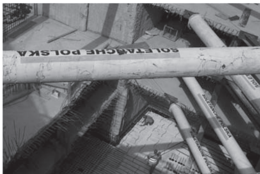
Figure 4. Construction site at Prosta St.
