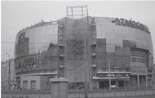
Figure 6. General view of the building with 4 level parking.
