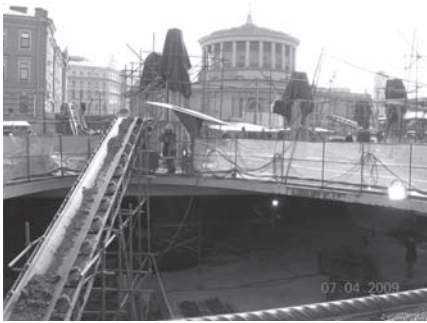
Figure 9. Excavation of the soil under the ceiling.
