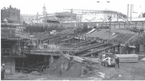
Figure 11. View of struts in the ditch.
