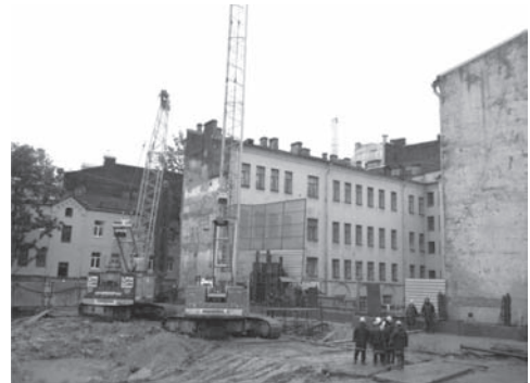
Figure 8. “Wall in ground” along one of the sides of the ditch.
