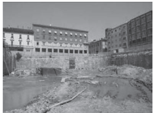
Figure 10. View on the job site.
