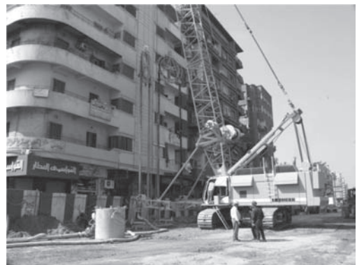
Figure 7. BAUER-cutter in front of occupied houses.
