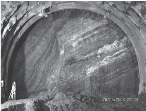
Figure 2. A South Toulon tunnel face.
