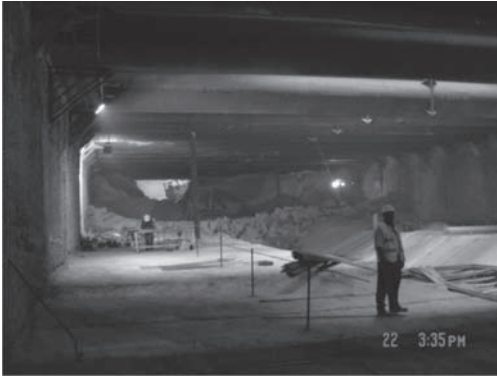
Figure 3. A view of Attaba station with temporary props.
