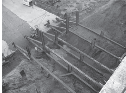
Figure 4. Execution of a partial excavation.
