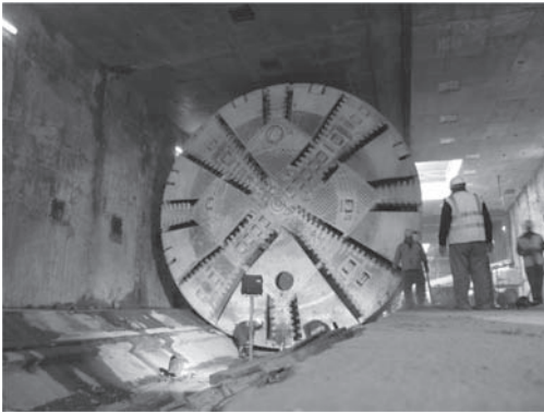
Figure 5. Slurry-shield-TBM during shifting.
