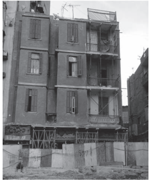
Figure 9. Old houses had to evacuated before starting cutting activities.
