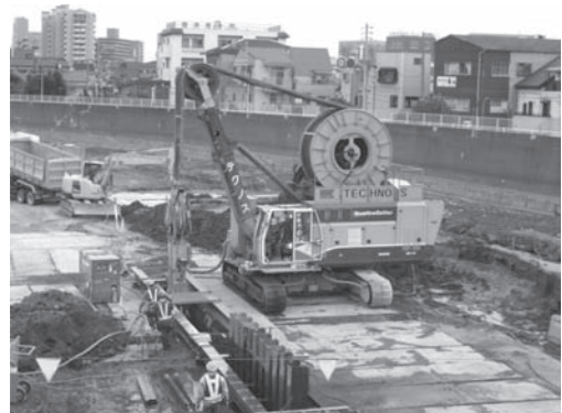
Figure 6. Wire-rope-suspended CSM unit, QuattroCutter Osaka, Japan.
