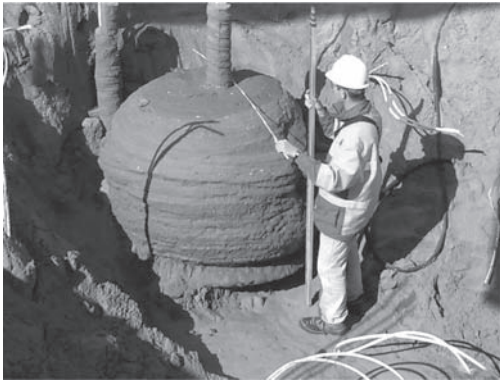
Figure 13. Chemical grouting body at a test field excavation.
