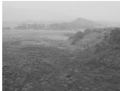
FIG. 2. View of Leuwigajah landfill failure in downstream direction.
