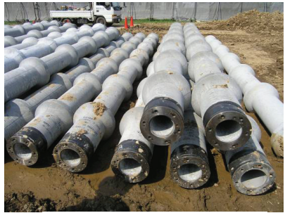
FIG.9. Shape of nodular pile.
