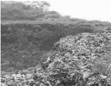
FIG. 1. Head scarp of failure of Leuwigajah landfill in Bandung of Indonesia.
