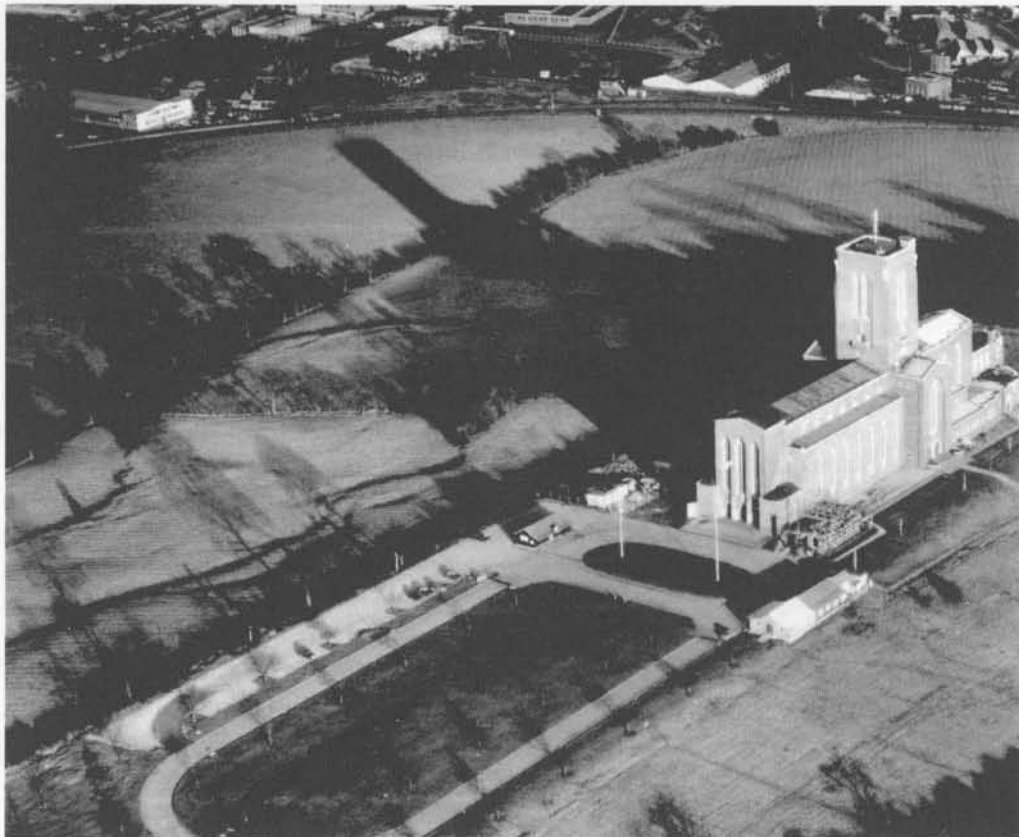
Fig. 2.12 Oblique air photo of Stag Hill landslide, Guildford
