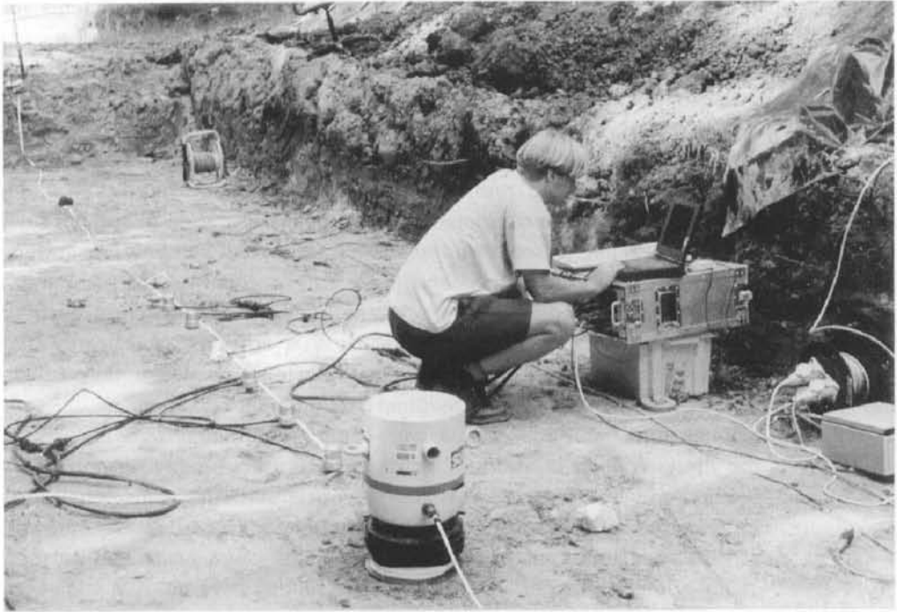
Fig. 4.69 Continuous surface wave system being used on site on a trial road subgrade. The computer-controlled vibrator is in the foreground with a line of six geophones behind (permission of GDS Instruments Ltd)
