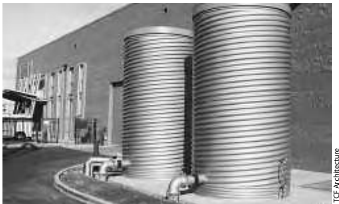
At the new Tacoma, WA, police facility designed by TCF Architecture, two 4,800-gallon tanks collect rainwater and recycle it for toilet flushing.
