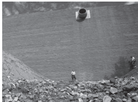
Figure 4-7. Walls with concrete block facing (right photo courtesy of R. Barrett)
