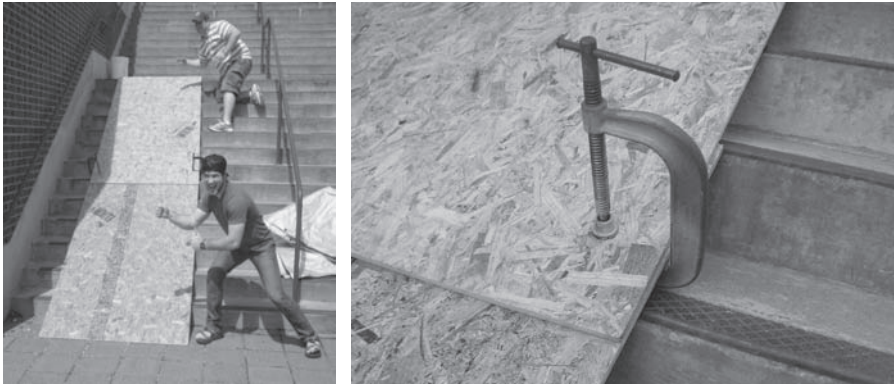
Figure 35-2. Left, boards set on stairs; right, detail of clamp holding boards together
