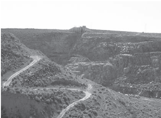
Figure 14-7. Teton Dam site showing heavily fractured rock abutment (Chadwick et al. 1976)
