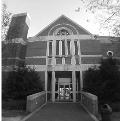
Figure 31-1. Civil engineering building at Auburn University, showing limestone, brick, concrete, and slate (roof). Also, the birthplace of Soils Magic
