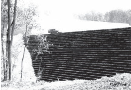
Figure 4-6. Wrapped face walls using geotextiles
