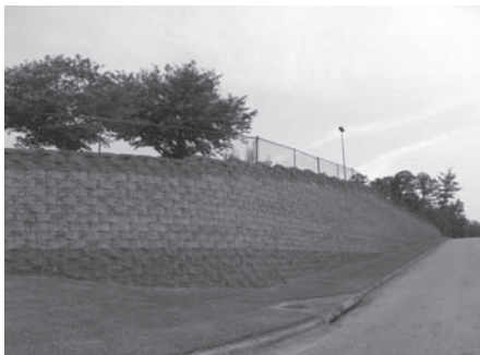
Figure 4-7. Walls with concrete block facing (right photo courtesy of R. Barrett)
