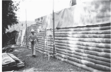
Figure 4-6. Wrapped face walls using geotextiles
