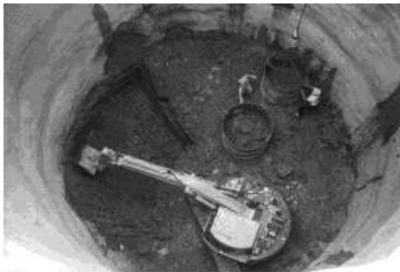
Figure 6.39 Shaft excavation in progress.
