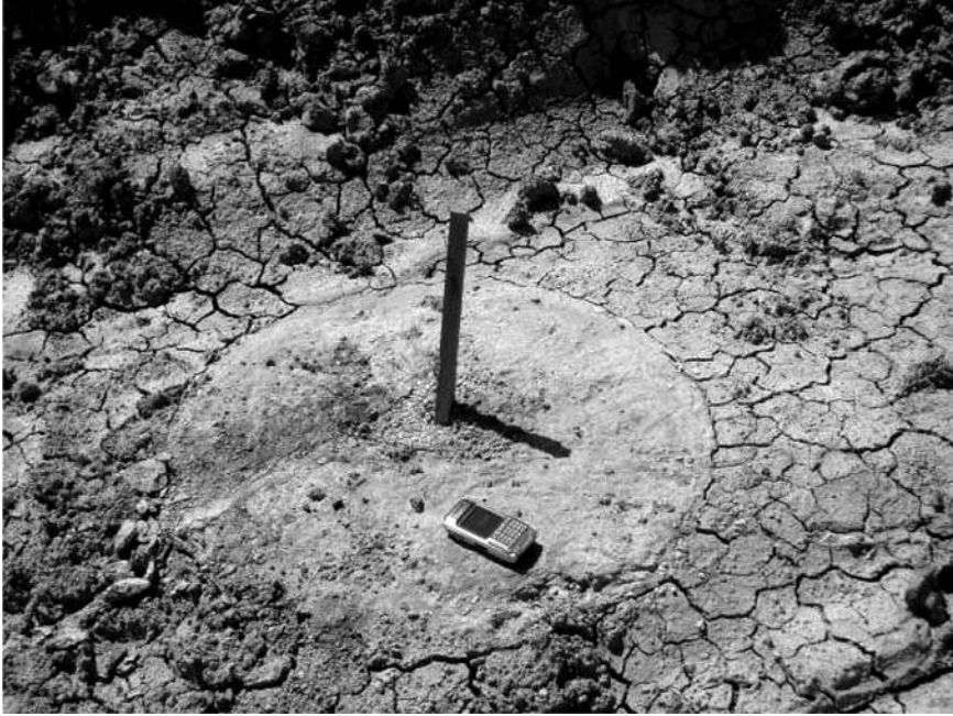
Figure 10.21 Exposed DSM column.
