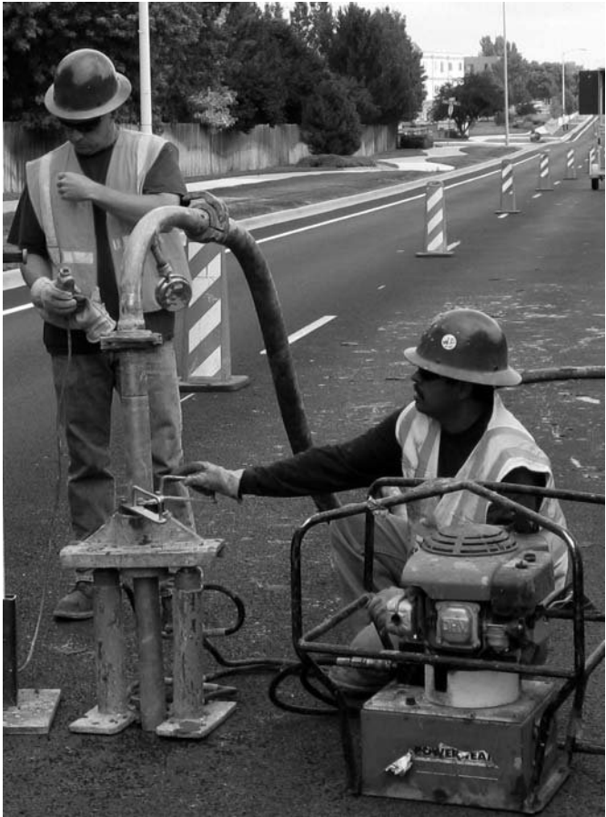
Figure 8.14 Hydraulic ram to extract LMG injection pipe. (Courtesy of Hayward Baker Inc.)
