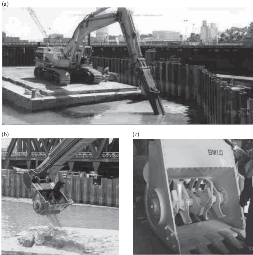
Figure 9.23 Shallow mixing equipment used at Fort Point Channel Site in Boston. (Courtesy of R. Jakiel.)
