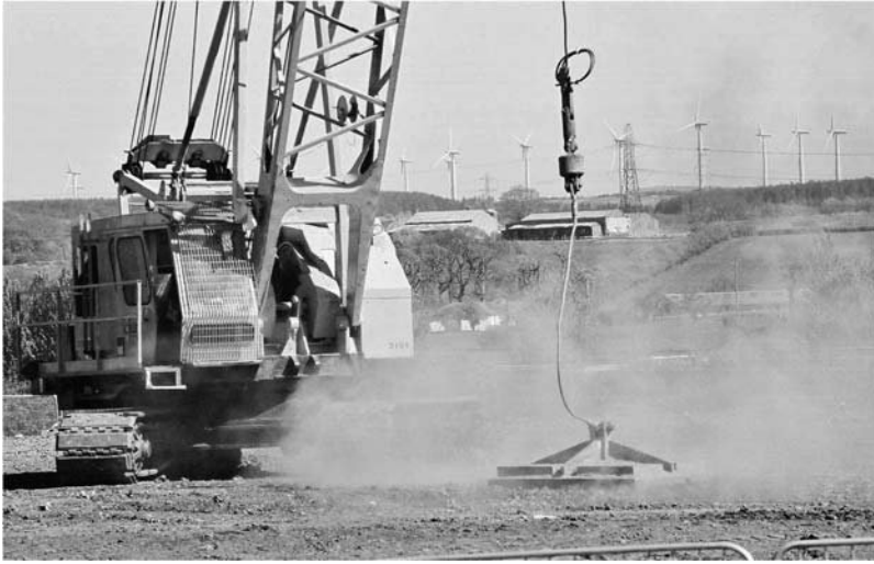
Figure 3.1 Typical crawler crane and equipment.
