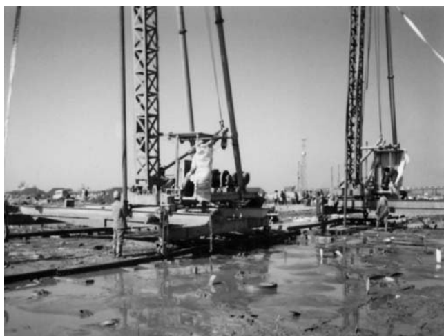
Figure 4.14 A light-weight truck-supported installation rig. (Courtesy of S.W. Yan.)
