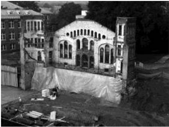
Figure 6.45 Excavated Avery Hall façade underpinned with jet-grouted soilcrete columns.
