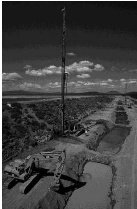
Figure 6.34 SuperJet grouting in progress at Wickiup Dam.
