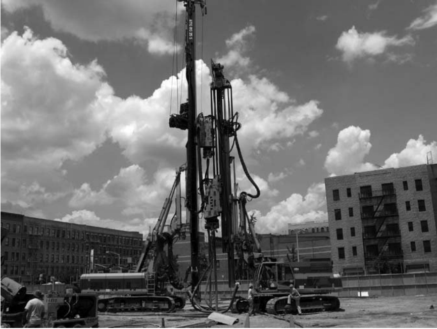
Figure 8.18 Large track-mounted drill rigs with telescopic masts installed the injection pipes in a single stroke to the maximum required treatment depth of 50 feet (15.2 metres). (Courtesy of Hayward Baker Inc.)
