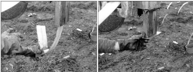
Figure 4.20 Use of an anchor plate for PVD installation. (Courtesy of J. Han.)
