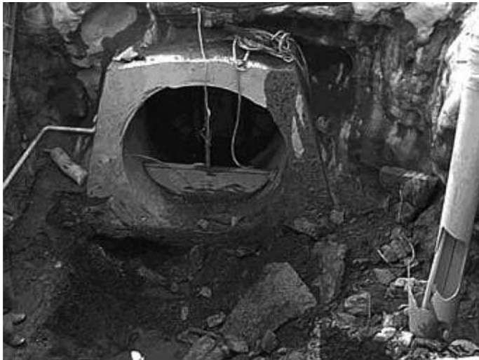
Figure 6.44 Soilcrete seal around and below the conduit with the bulkhead visible within the conduit.
