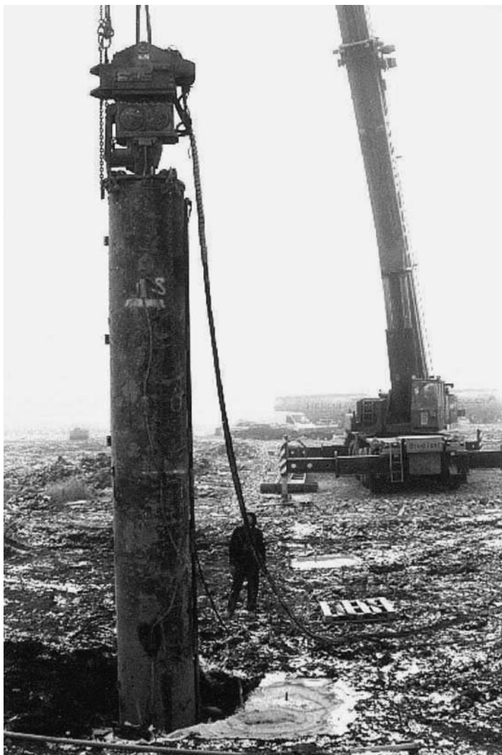
Figure 10.23 Extracted column. (From Axelsson, M. (2001). Djupstabilisering med Kalkcementpelare-Metoder for Produktionsmassig Kvalitetskontroll i Falt (Deep Stabilization with Lime Cement Columns – Methods for Quality Control in the Field), Report No. 8. Linköping, Sweden: Swedish Deep Stabilization Research Centre.)
