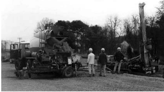
Figure 8.10 Concrete truck delivers LMG to grout site. (Courtesy of Hayward Baker Inc.)
