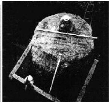
Figure 6.8 (a) Dual colliding jets. (b) Columns produced by dual colliding jets.
