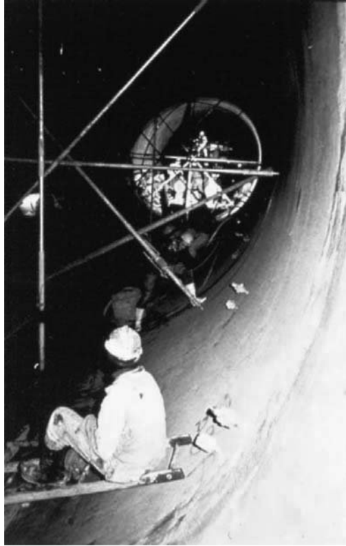
Figure 5.7 Drakensberg Pumped Storage Scheme, RSA, Tailrace Tunnel, Precompression grouting, ESCOM, Rodio SA, 1970s.
