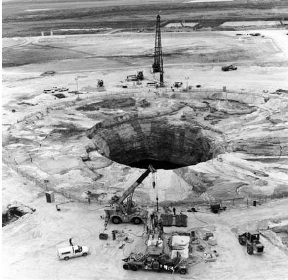
Figure 8.4 LMG to stabilise large sinkhole at a central Florida mining facility. (Courtesy of Hayward Baker Inc.)
