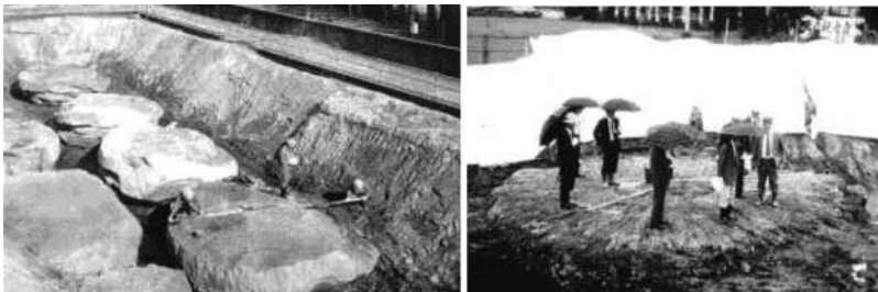
Figure 6.5 Exposed SuperJet columns during technology development.
