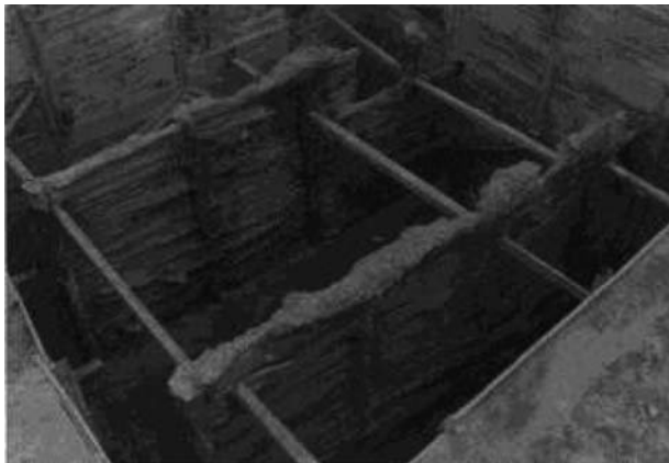
Figure 6.2 Exposed jet grout panels.
