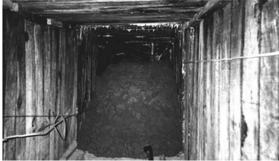
Figure 8.7 LMG used to fill a mine tunnel. (Courtesy of Hayward Baker Inc.)
