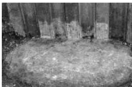
Figure 6.11 JACSMAN column abutting sheet piling.
