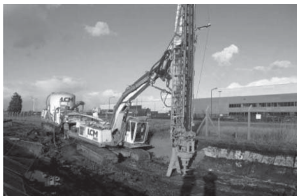
Figure 10.24 Installation of DSM. (Courtesy of Keller Géotechnique.)
