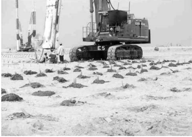
Figure 4.48 Extrusion of viscous pore water and mud during PVD installation. (From Chu, J., Bo, M.W. and Choa, V. (2006). Geotextiles and Geomembranes , Vol. 24, No. 6, pp. 339–348.)
