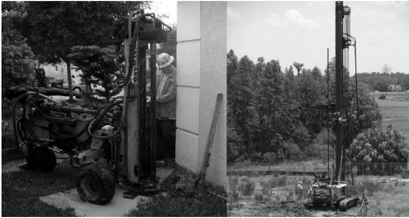
Figure 8.13 Small-wheeled and large-tracked drills to install LMG injection pipe. (Courtesy of Hayward Baker Inc.)
