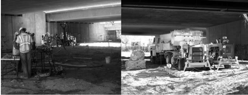
Figure 8.21 Small-tracked drill installing the injection pipes (left) and truck mounted batch plant producing LMG (right). (Courtesy of Hayward Baker Inc.)
