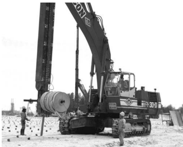
Figure 4.13 A static push-in type of PVD installation rig.
