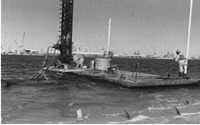
Figure 4.15 A floating raft for PVD installation in shallow water (From Chu, J., Bo, M.W. and Arulrajah, A. (2009). Soil improvement works for an offshore land reclamation. Proceedings of the Institution of Civil Engineers—Geotechnical Engineering , Vol. 162, No. 1, pp. 21–32.)
