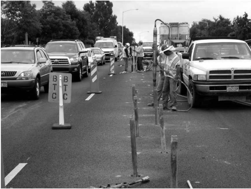
Figure 8.12 Hand equipment to install LMG injection pipe. (Courtesy of Hayward Baker Inc.)
