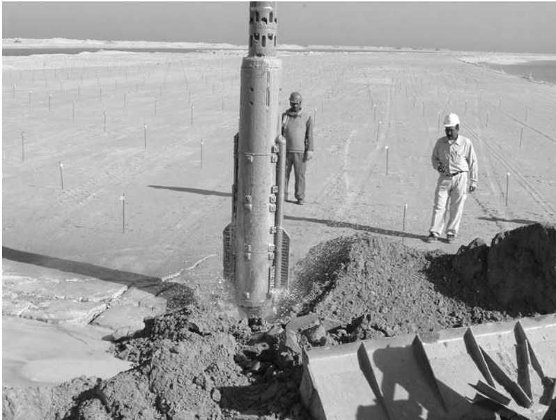
Figure 2.19 Compaction works at Palm Island.
