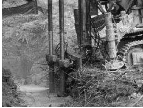
Figure 6.31 Dual axis jet grouting operation for the jet-grouted soilcrete barrier wall.
