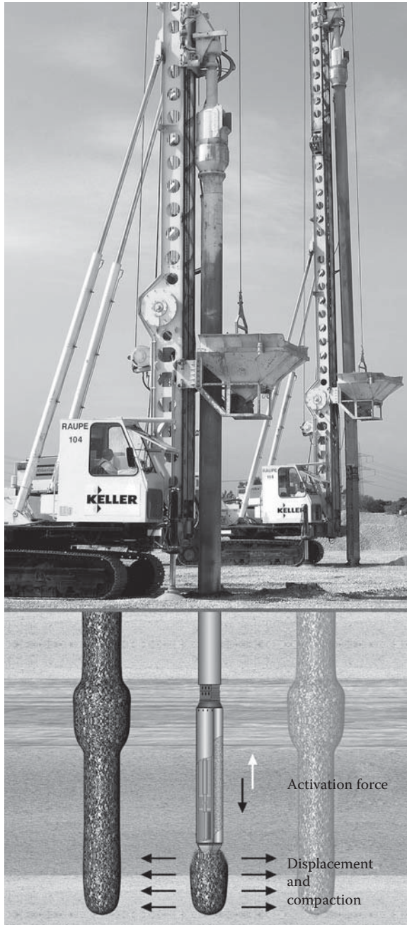
Figure 2.4 Vibro cat with activation force. (Courtesy of Keller Group.)
