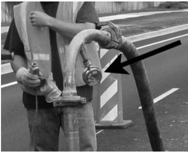
Figure 8.15 Pressure gauge and gauge saver near top of grout injection pipe. (Courtesy of Hayward Baker Inc.)
