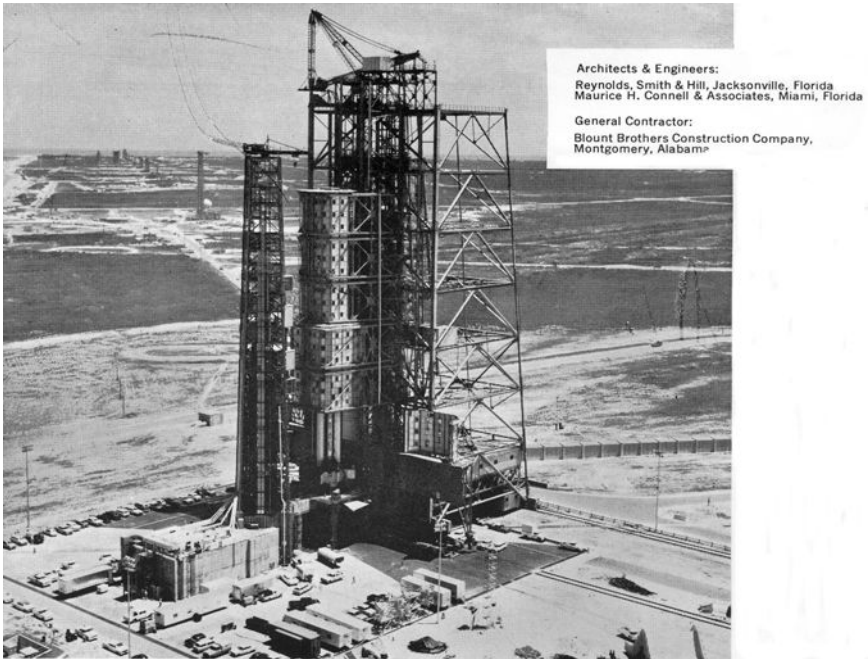
Figure 2.11 Saturn Rocket Launching Facility at Florida (Vibroflotation Foundation Company brochure)
