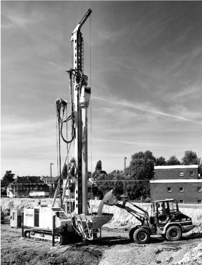
Figure 4.2 Vibrocat with bottom feed vibrator (by courtesy of Keller Group plc)
