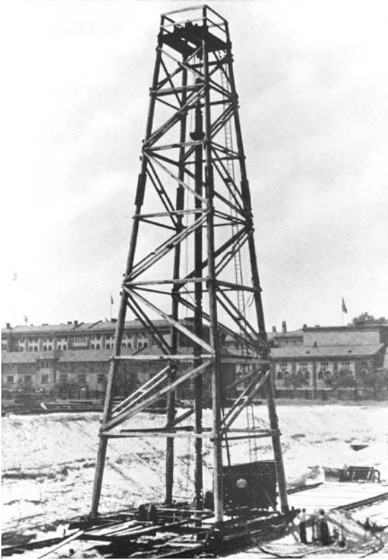
Figure 2.4 Vibro compaction employing wooden gantry, 1939
