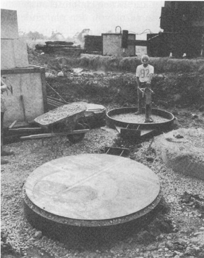
Figure 2.15 Preparation of a horizontal load test on vibro stone columns
