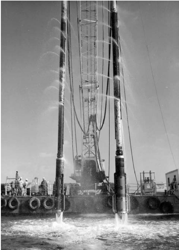
Figure 3.7 Crane-hung twin vibrators for underwater compaction (by courtesy of Keller Group plc)
