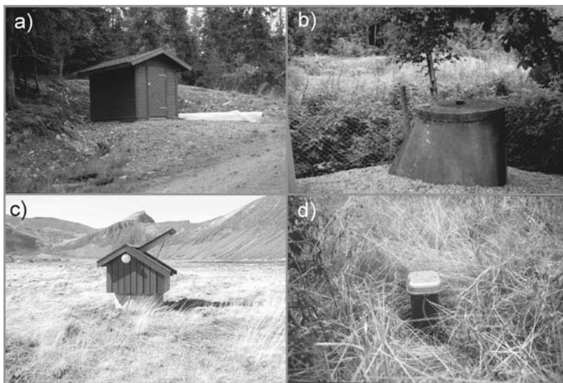
Figure 3. Examples of wellhead completions. a) Well-house, b) concrete well-protection (manhole), c) concrete well-protection with well-cover (small “house”) instead of a concrete lid and d) no protection except a proper cap on top of the casing.
