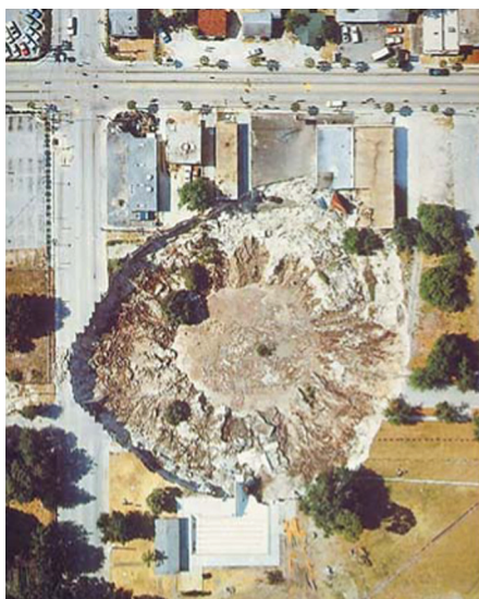
Chapter 17 – Figure 6 Collapse sinkholes, such as this one in Winter Park, Florida (1981), may develop abruptly (over a period of hours) and cause catastrophic damage (Galloway et al. , 1999).
