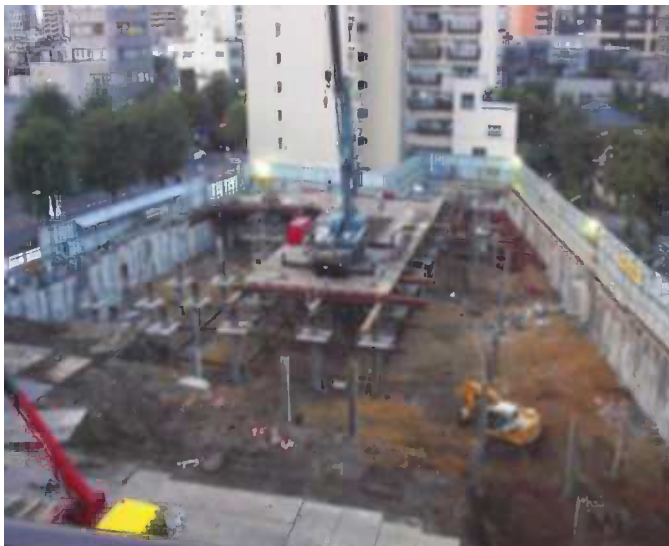
Chapter 16 – Figure 6 View of the construction site.
