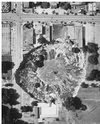
Figure 6 Collapse sinkholes, such as this one in Winter Park, Florida (1981), may develop abruptly (over a period of hours) and cause catastrophic damage (Galloway et al. , 1999) (See colour plate section).
