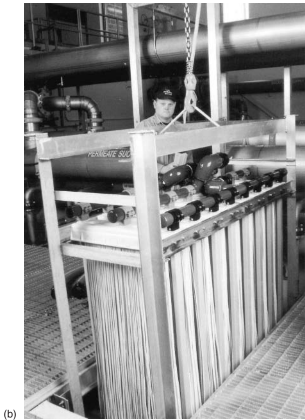
The modular filter rack is easily removed from the filter cell for convenient maintenance.
