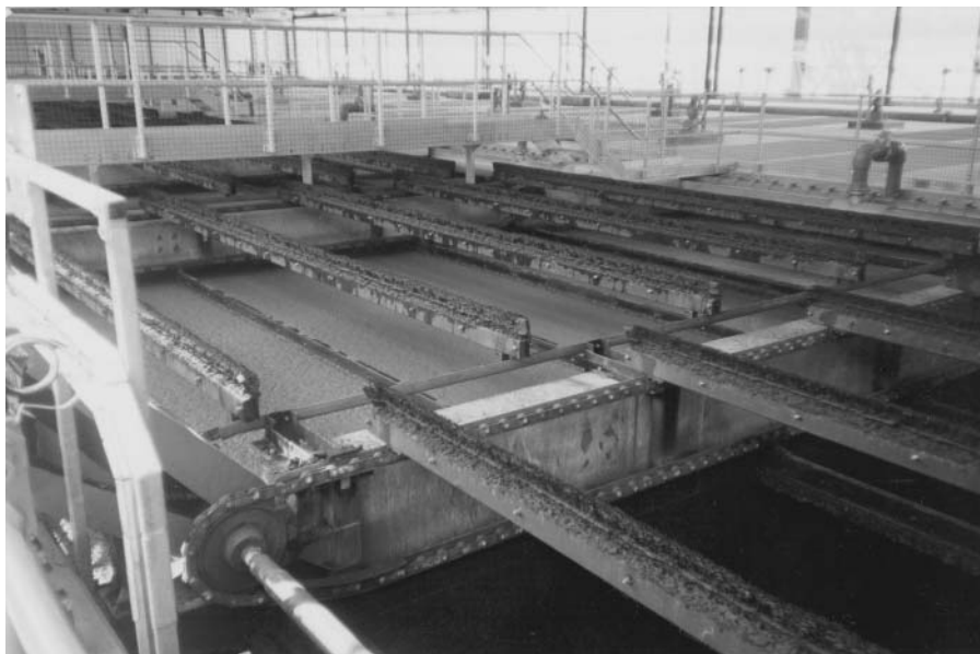
Fig. 11–27. Dissolved air flotation system at the Arvika Water Treatment Plant in Sweden (Courtesy of The F. B. Leopold Company Inc.)
