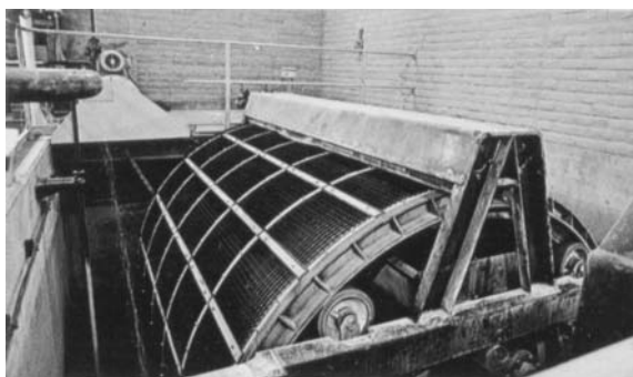
Fig. 8-12. Microscreen installation (Courtesy of USFilter-Rex and LinkBelt Intake Products)
