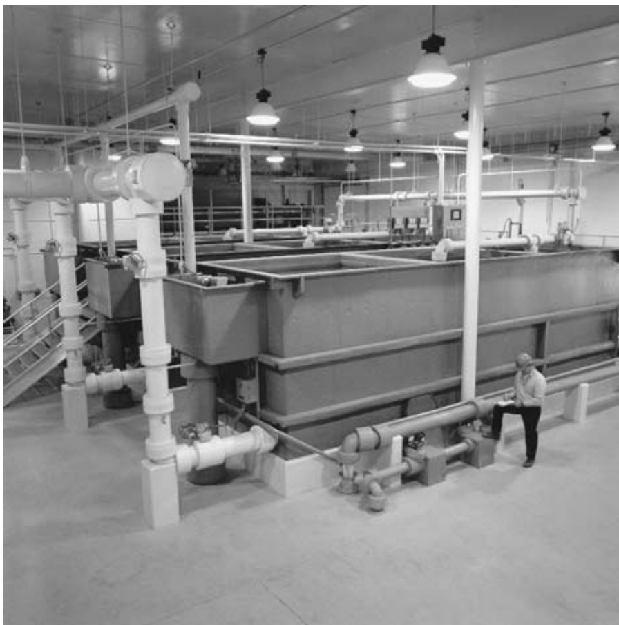
Fig. 25-11. Photo of 700-gpm Pacer II package plant (Courtesy of Roberts Water Technologies)
