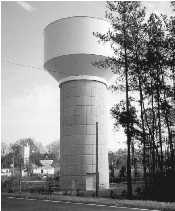
Fig. 27-6. Elevated concrete and steel tank
