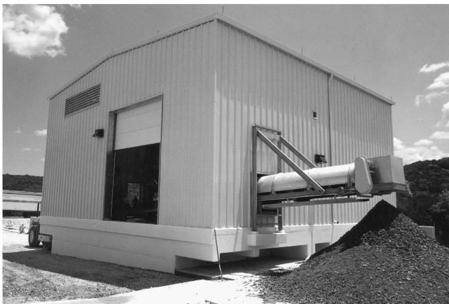
Fig. 23–18. Alum sludge cake discharging from belt filter press at Cedar Park, Texas (Courtesy of Ashbrook-Simon-Hartley)
