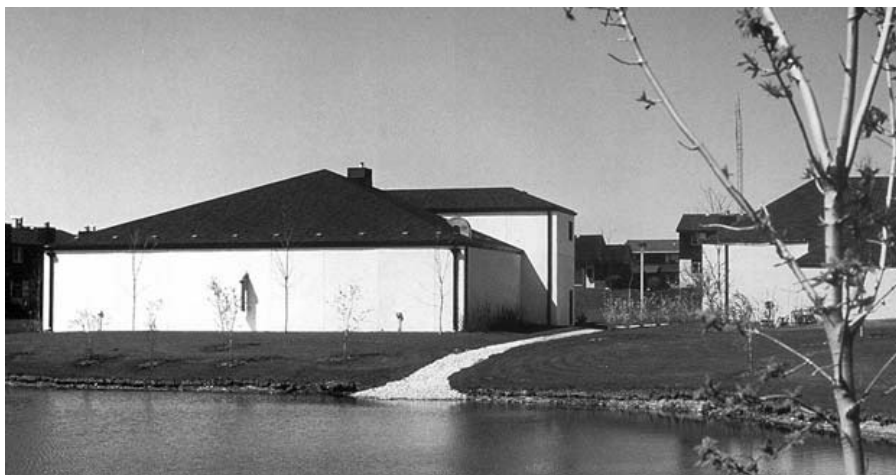
Fig. 27-5. Disguised concrete tanks
