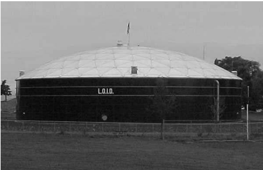
Fig. 27-4. Geodesic dome (Courtesy of Northwest Permastore Systems, Inc.)
