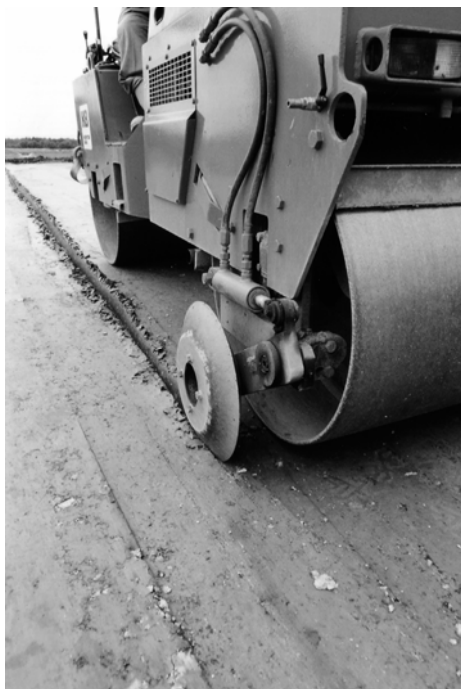
Fig. 11.3. A groove is milled into the surface of a compacted clay liner into which the sensor cable is laid. The extent of preparatory work on the subgrade of the geomembrane depends highly on the subgrade properties. In any case one has to meet the requirement, that indentations imprinted on the geomembrane by the cable and electrodes have to fall short of the acceptable limits (see Sect. 8.3.1)
