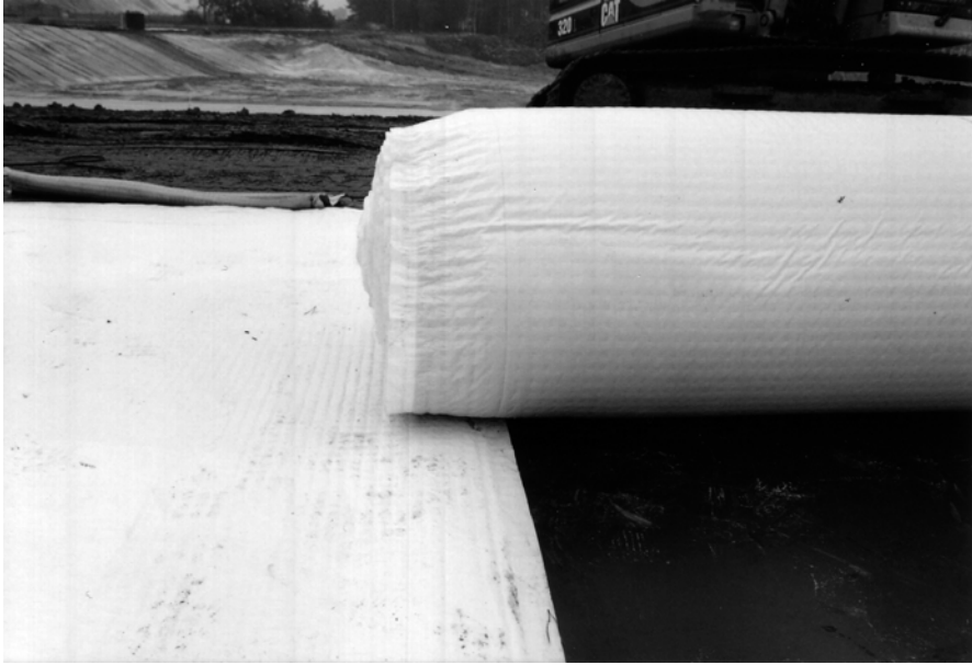
Fig. 8.1. The installation of the sand-filled protective mat or geocontainer (MDDS mat) on a geomembrane is shown in Fig. 9.9. This picture illustrates a technical weaving trick in the production of the double fabric with spacers, into which the sand is filled. The double fabric is woven in such a way that it thins out toward the edges in a wedge-shaped way and the rolls are installed in a manner that the two wedges lie on top of one another. Thus a sharp joint edge or a sharp-edged overlap can be avoided and the protective effect can be ensured within the joint range without any restriction
