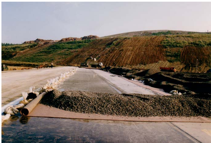
Fig. 9.10. This photograph shows the anchoring bar or fixing berms. On the front end of the geomembrane a thick nonwoven geotextile was unrolled as a protective layer and on top of it a heap of gravel was applied. Thus the geomembrane is fixed. Courtesy Schicketanz Consulting Engineers, Aachen
