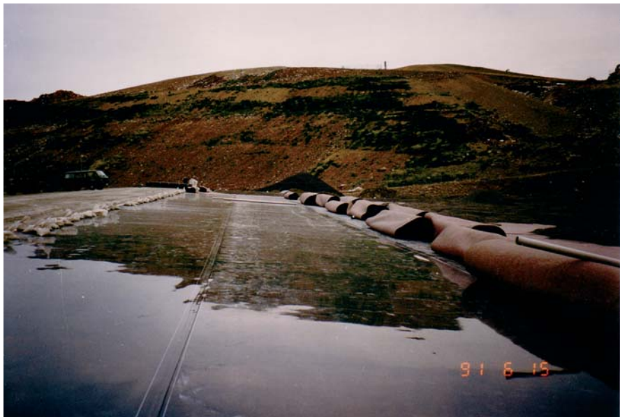
Fig. 9.12a. This and the following photographs demonstrate that using the anchoring technique, complete flatness can be achieved for the geomembrane. Courtesy Schicketanz Consulting Engineers, Aachen
