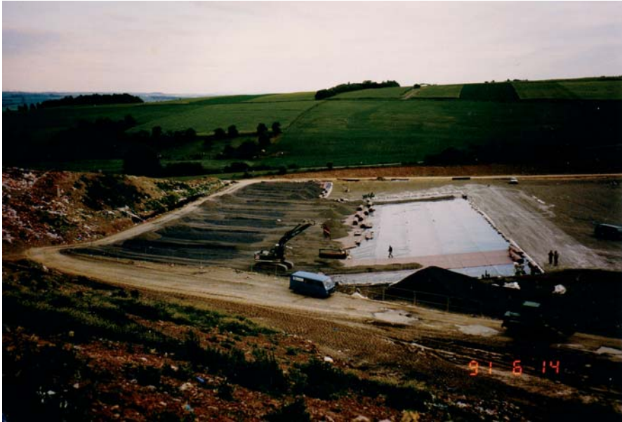
Fig. 9.11. In the background of the four installed geomembranes the anchor bar is already completed. In the front the gravel filling is being applied with an excavator early in the evening. With evening cooling after sunset the four geomembranes will become completely flat. The nonwoven geotextile rolls are then unrolled over the whole surface and the gravel filling applied. Courtesy Schicketanz Consulting Engineers, Aachen
