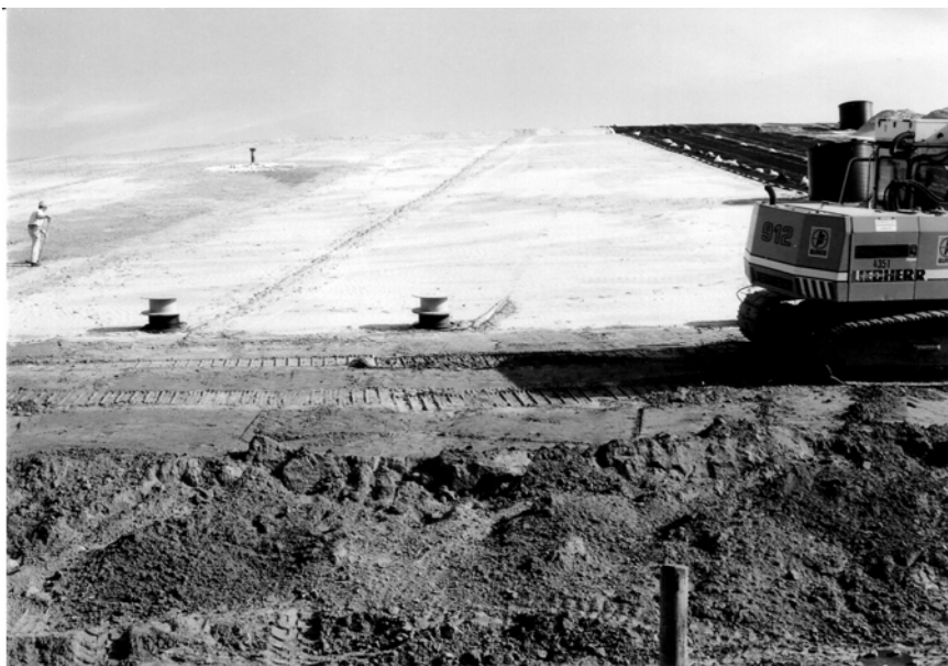
Fig. 11.5. View of the subgrade prior to the installation of the geomembrane with the cables installed in a regular distance of about 5 m
