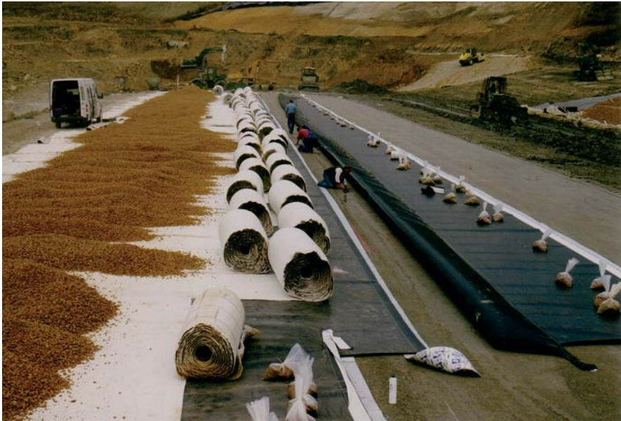
Fig. 9.9. This photograph illustrates the different stages of composite liner construction. In the far background the subgrade of the landfill liner system is being prepared and right in the background the compacted clay liner is being built. On the surface of the completed mineral layer a geomembrane has been unrolled. Small defects in the surface are being manually eliminated even after unrolling the geomembrane. The geomembrane is then aligned and pulled flat. In this construction project MDDS sand mats of the Gebrüder Friedrich GmbH company are used as a protective layer, which cover the installed geomembranes and ballasted with drainage gravel. The anchoring technique becomes particularly simple using the sand mat rolls since no fine-gravel mineral protective layer needs to be installed. Courtesy of Gebrüder Friedrich GmbH
