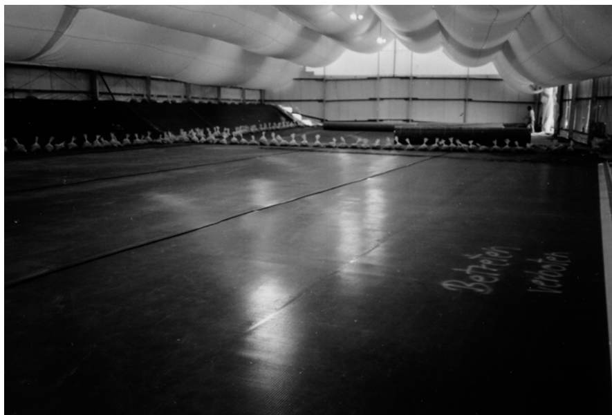
Fig. 9.4. In a large heated tent a composite liner was constructed in the middle of winter. Anchoring technique (Riegelbauweise) can ensure a complete intimate contact between geomembrane and mineral layer even under these conditions (Sect. 9.3.2) (Krath and Schwarz 1993; Schicketanz 1995). Courtesy Schicketanz Consulting Engineers, Aachen
