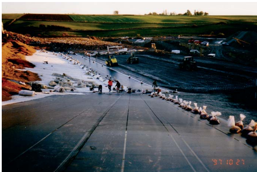
Fig. 9.12c. Complete flatness can be achieved even on long and steep slopes, as this photograph shows. Courtesy Schicketanz Consulting Engineers, Aachen
