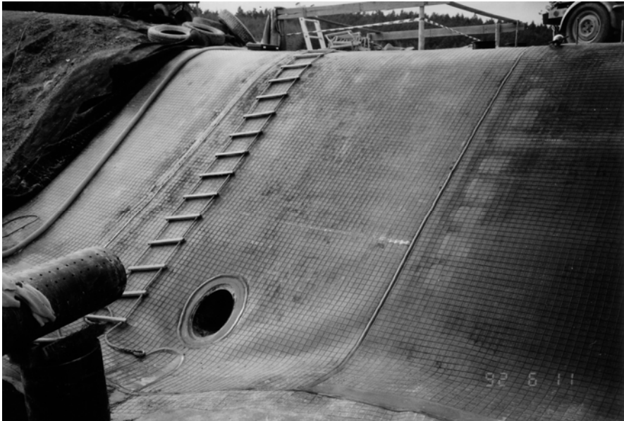
Fig. 9.12b. This photograph shows that the anchoring technique provides complete flatness even in critical areas (slope toe and pipe penetration constructions). In such places where hand-welded extrusion fillet seams occur in higher frequency and standing leachate can be expected, special care and high technical installation skills are required. Only experienced, particularly qualified and well-equipped specialist installation companies can master this task. Courtesy Schicketanz Consulting Engineers, Aachen
