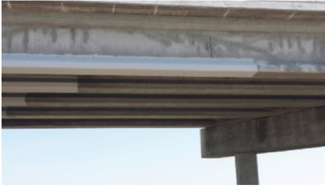
Figure 2.82 Repair of Prestressed Concrete Beam With FRP.
