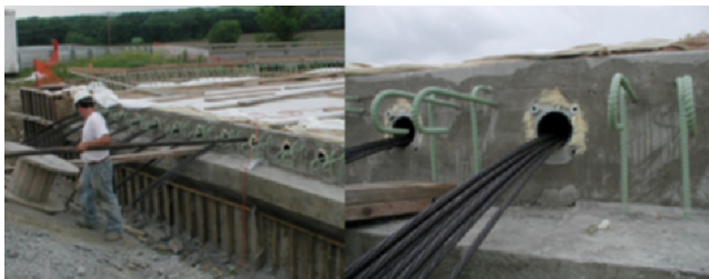
Figure 2.72 Posttension Ducts in Haunched Slab.
