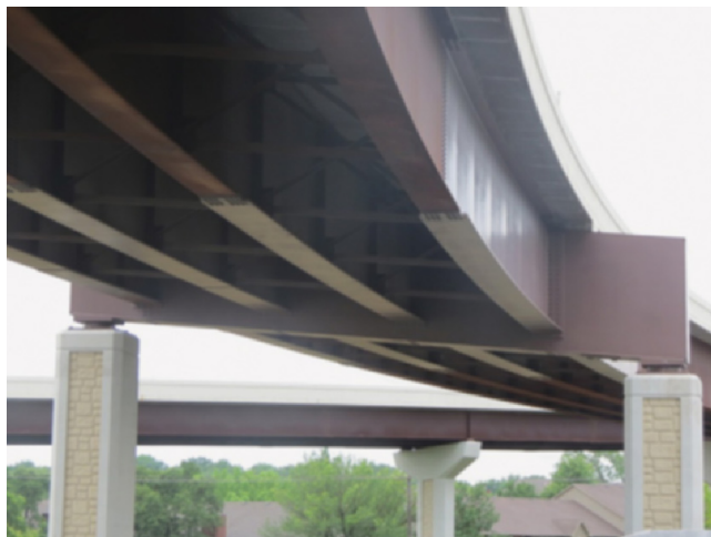
Figure 2.19 Steel Pier Beam on Straddle Bent.
