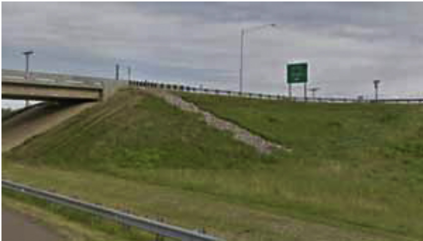
Figure 4.4 Rock Flume-Off of Bridge Approach.
