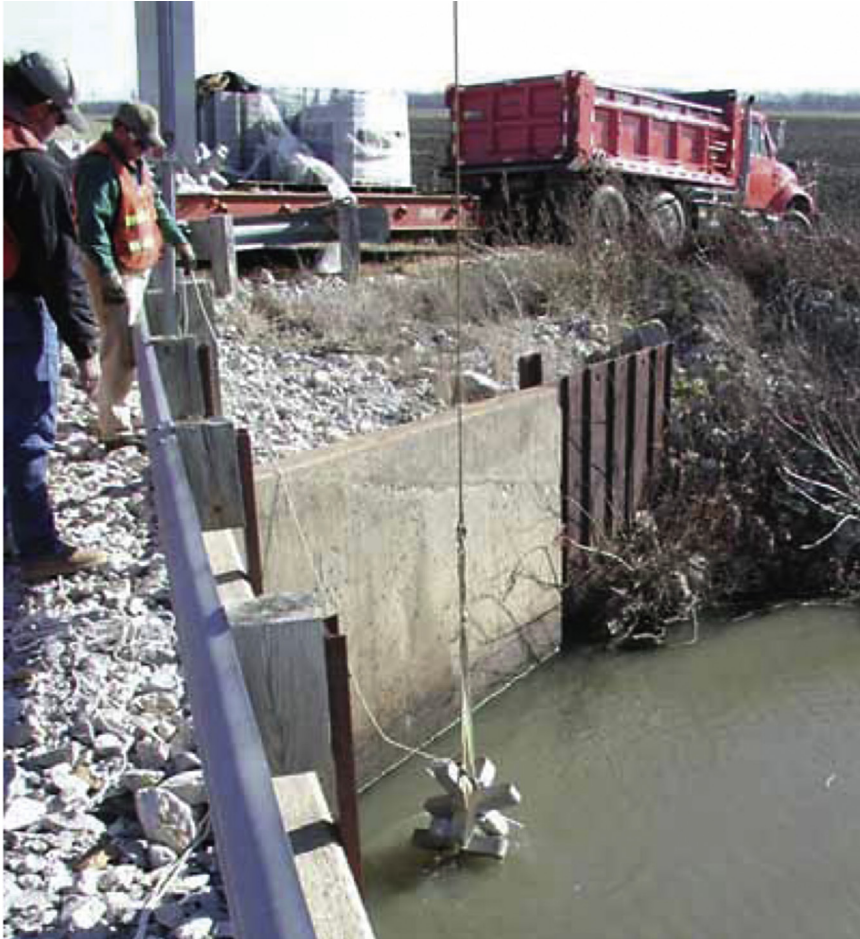
Figure 4.14 Maintenance Forces Placing “A-Jacks.”
