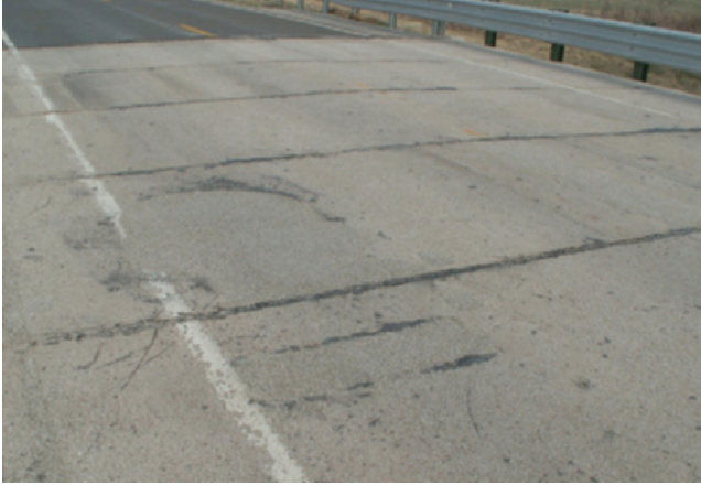
Figure 2.31 Wearing Surface of Extruded FRP Deck Panels.
