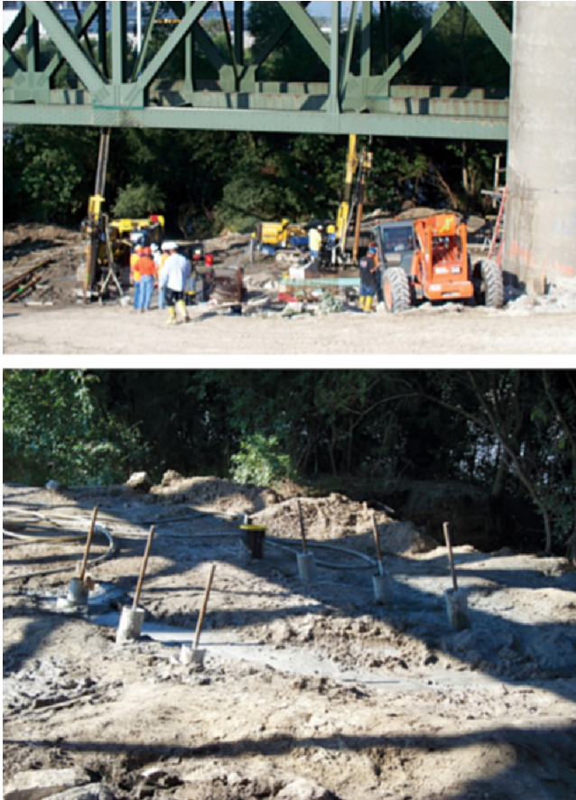
Figure 2.23 Installation of Micropile.
