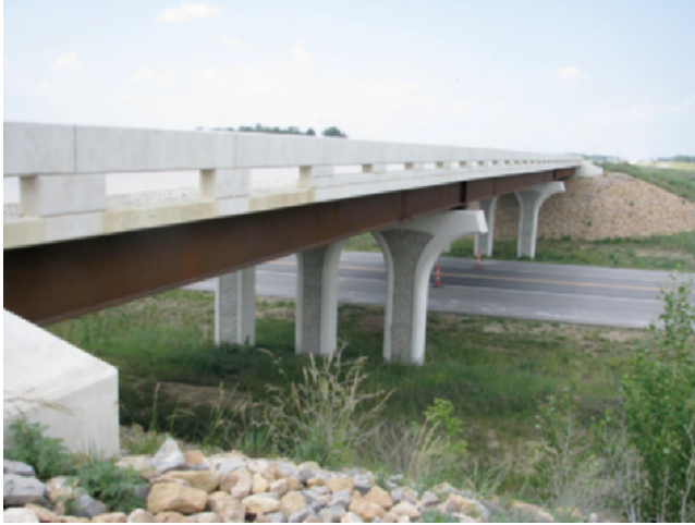
Figure 2.38 Steel Girder Bridge.
