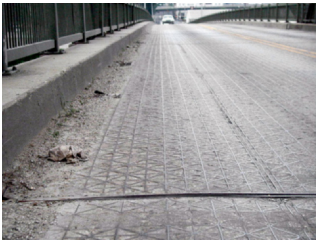
Figure 2.30 Filled Steel Grate Deck.
