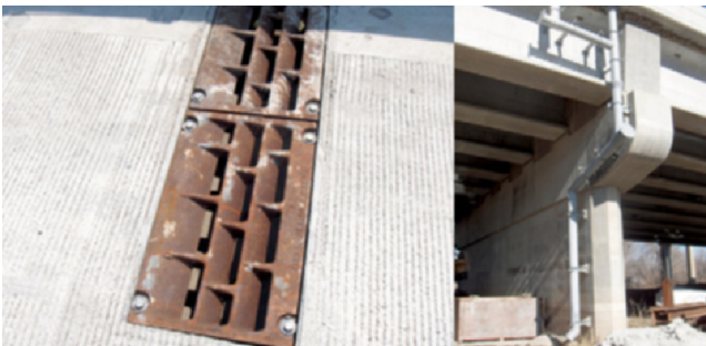
Figure 2.32 Deck Drain.
