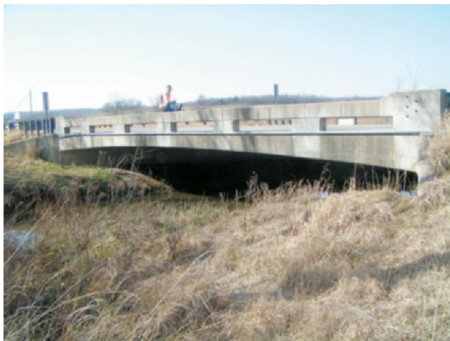
Figure 2.37 Single Span Reinforced Concrete Haunched Slab Bridge.
