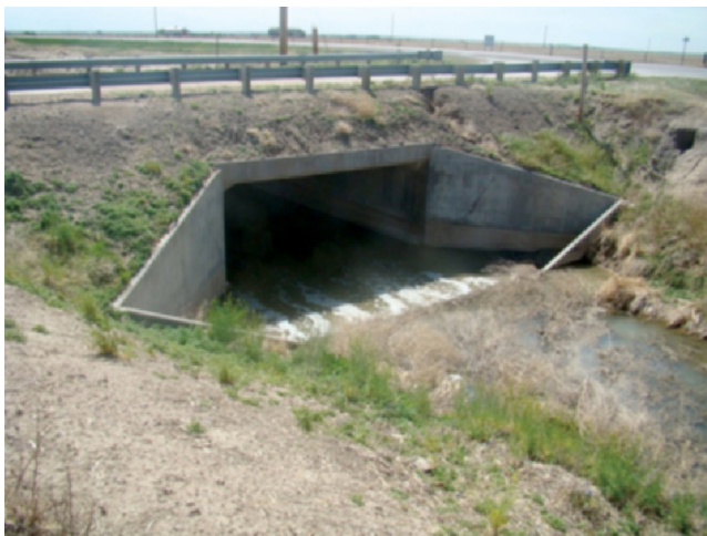
Figure 2.1 Typical Single Cell Culvert Structure.
