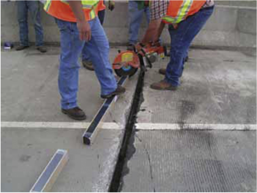
Figure 4.20 Installation of Pressure Relief Joint.
