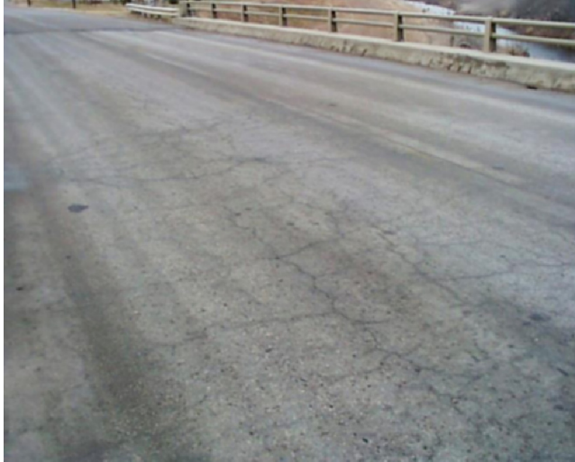
Figure 2.63 Map Cracking.
