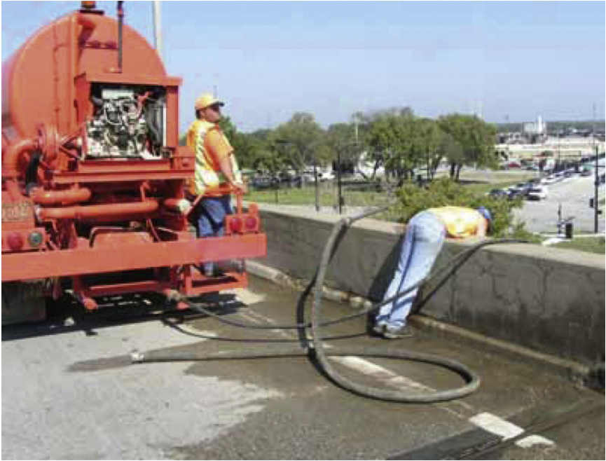
Figure 4.3 Flush Truck in Operation.
