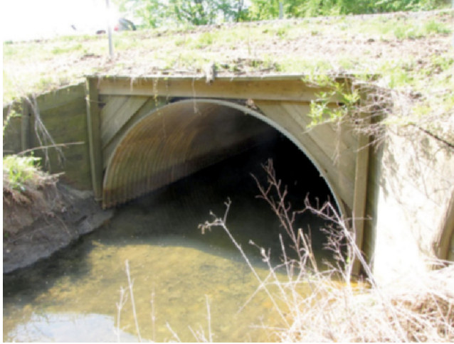
Figure 2.8 Timber Headwall on Corrugated Metal Pipe.
