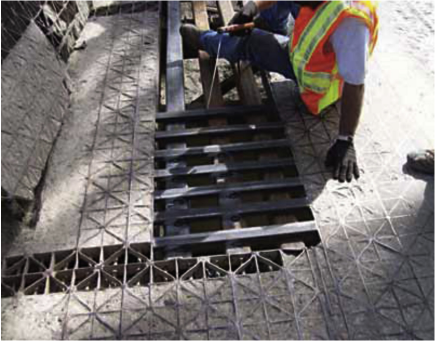
Figure 5.32 Repair of Steel Grid Deck.
