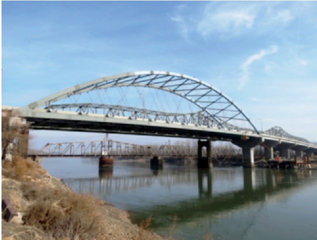
Figure 2.48 Network Tied Arch Bridge.
