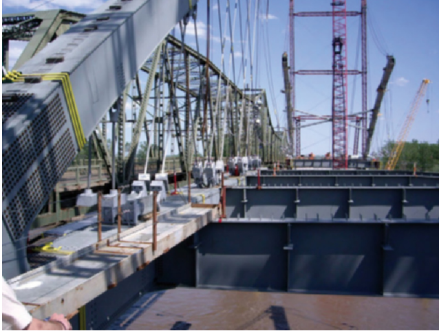
Figure 2.74 Steel Cables for Network Arch.
