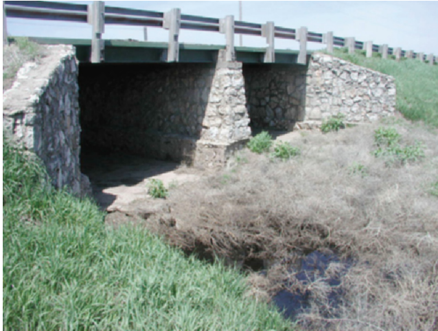
Figure 2.81 Stone Masonry Substructure.
