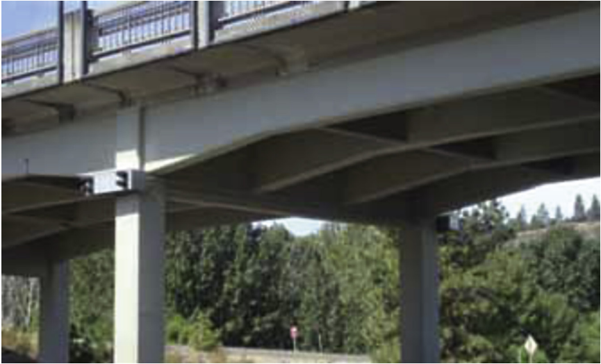
Figure 5.55 Posttension Retrofit of Pier Cap.
