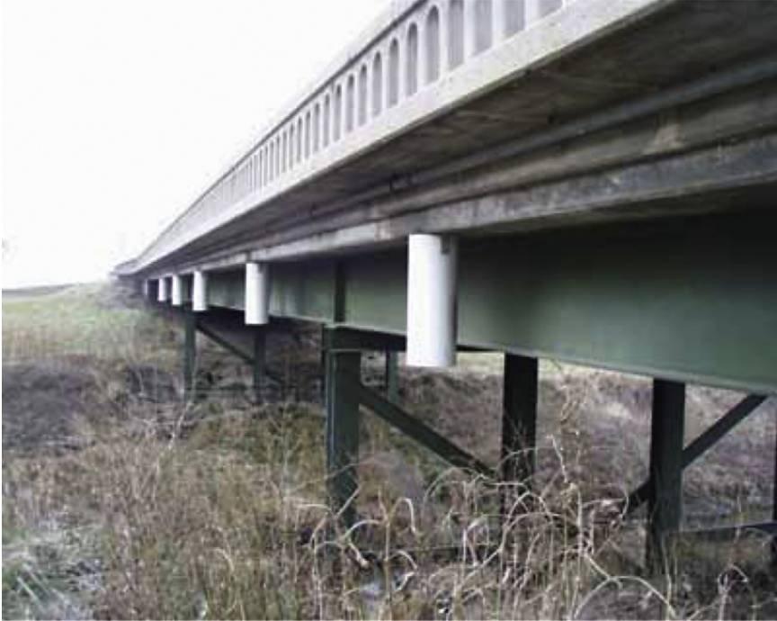
Figure 4.5 Drain Extension Retrofit.
