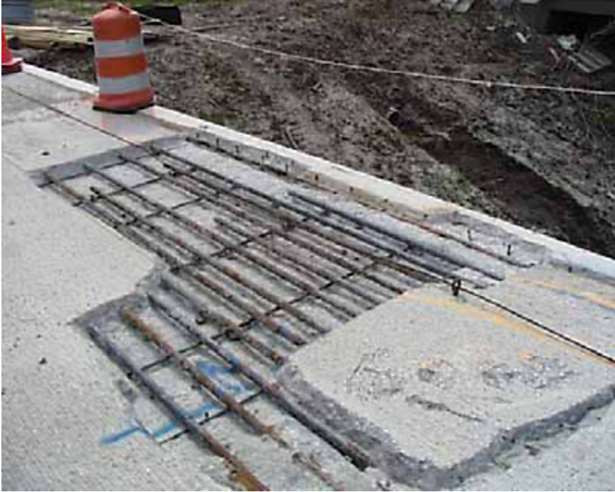
Figure 4.7 Area Prepared for Partial Depth Patching.
