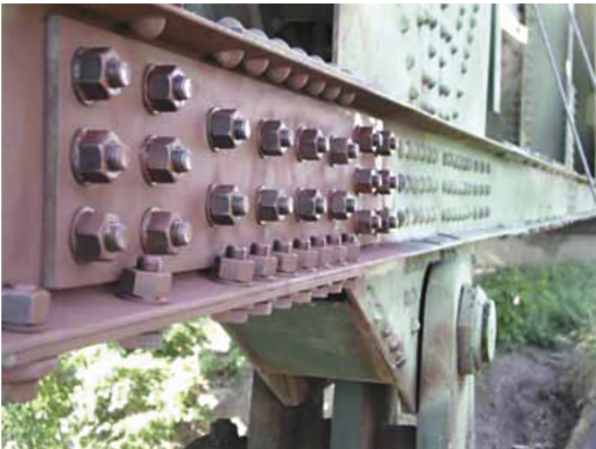
Figure 5.20 Repair Splice in Truss Chord.
