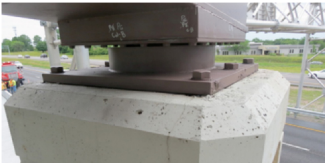
Figure 2.36 Pot Bearing.
