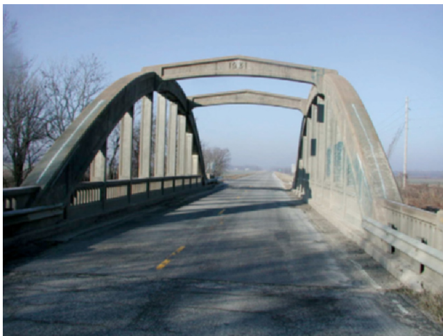
Figure 2.47 Reinforced Concrete Arch Bridge.
