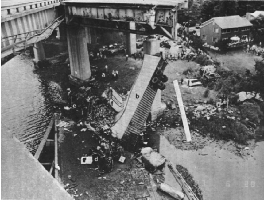
Figure 1.11 Collapsed Section of Mianus River Bridge. (From 1983 NTSB Report [16]).
