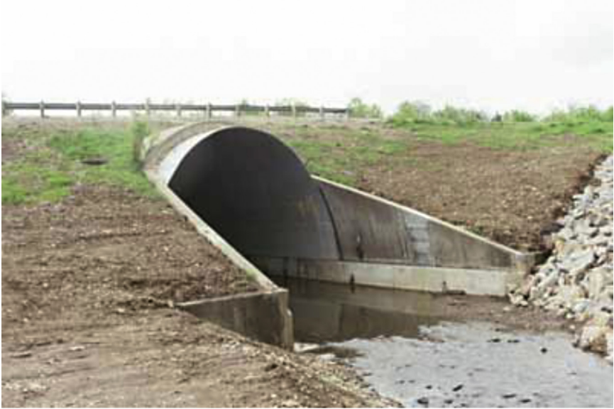
Figure 5.66 Reinforced Concrete Arch Culvert Lined With Corrugated Steel.
