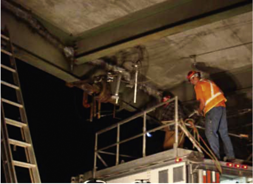
Figure 5.24 Restraint Applied to Girder Being Heat Straightened.
