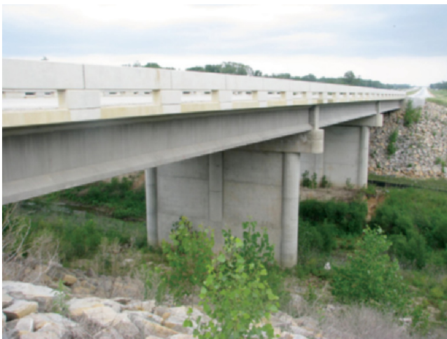
Figure 2.39 Prestressed Concrete Beam Bridge.
