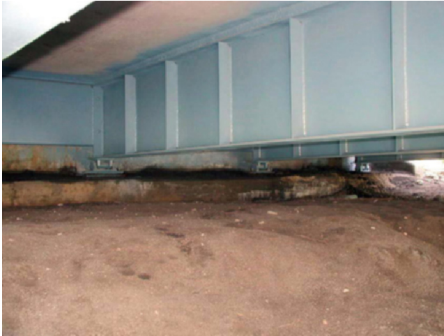
Figure 2.13 Bearing Seat on Abutment Backwall.
