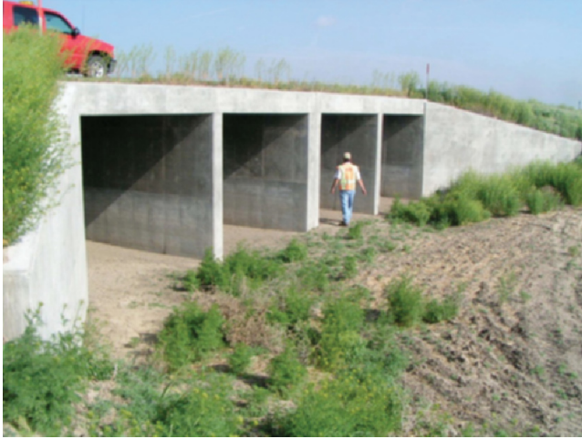
Figure 2.2 Multiple Cell At-Grade Box Bridge.
