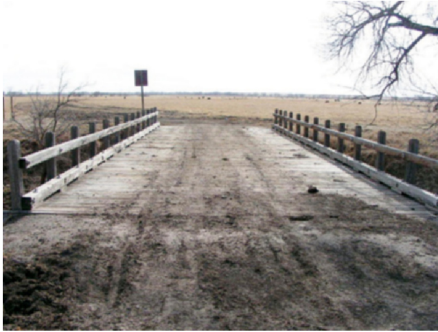
Figure 2.29 Timber Deck.
