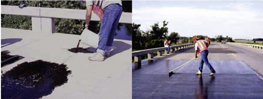
Figure 4.10 Deck Sealing Operation.
