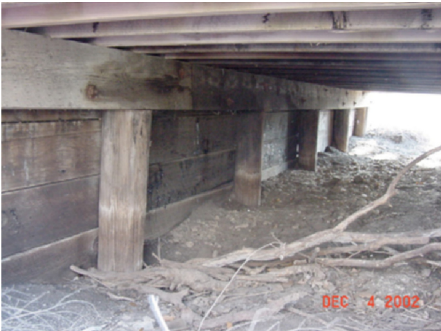
Figure 2.79 Short Span Timber Bridge.
