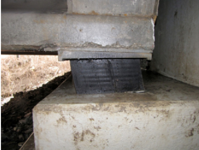
Figure 2.35 Reinforced Elastomeric Bearing.
