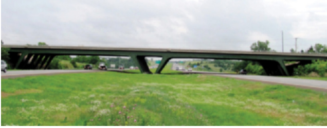
Figure 2.42 Welded Steel Rigid Frame Bridge.
