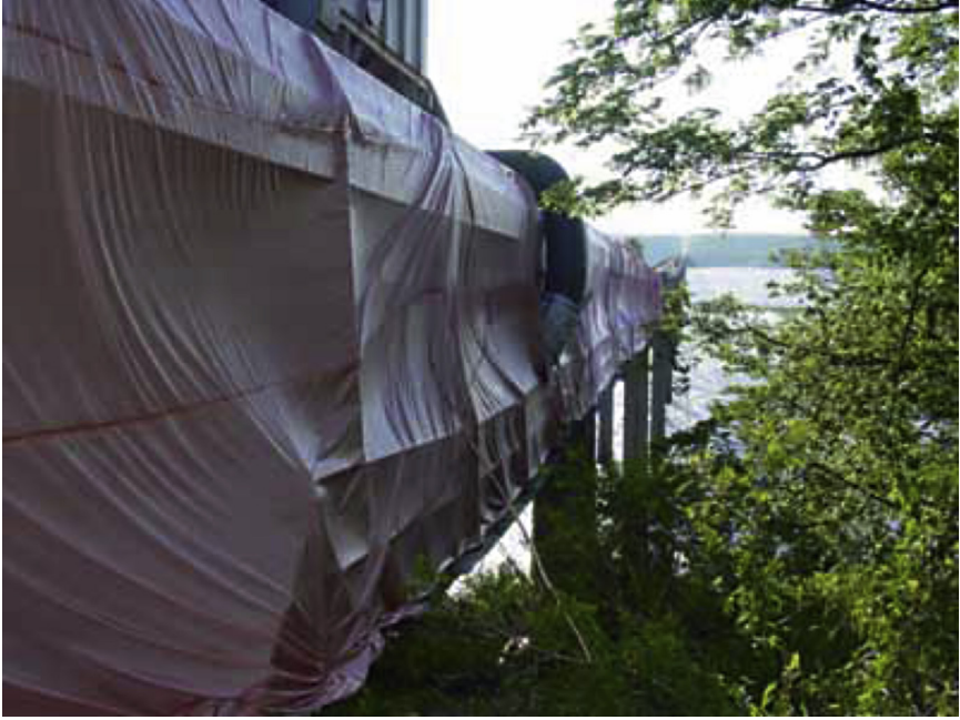
Figure 5.53 Containment for Paint Removal on Steel Girder Bridge.
