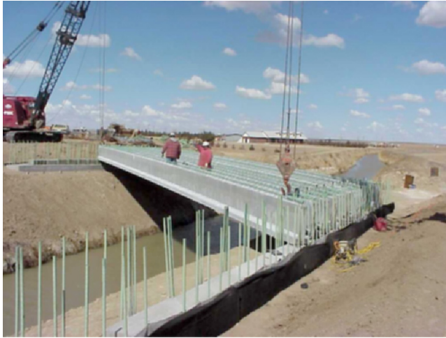
Figure 2.71 Construction of Prestressed Concrete Inverted-T Beam Bridge.
