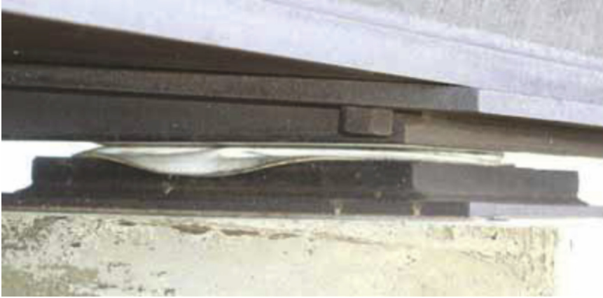
Figure 5.46 Teflon Sliding From PTFE Bearing.
