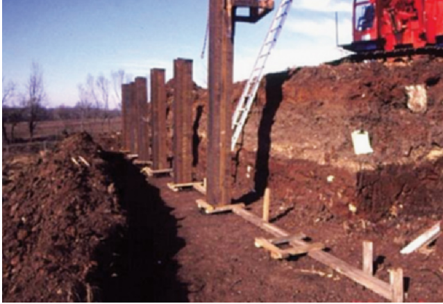
Figure 2.20 Steel H-Piles.
