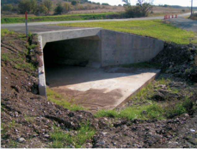
Figure 2.6 Reinforced Concrete Box With Concrete Apron.
