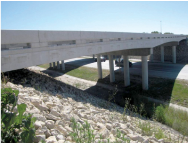
Figure 2.43 Reinforced Concrete Haunched Slab on Columns.
