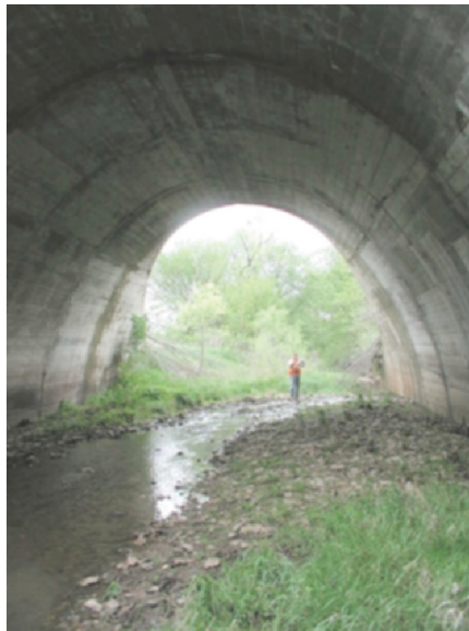
Figure 2.5 Inside of Reinforced Concrete Arch.
