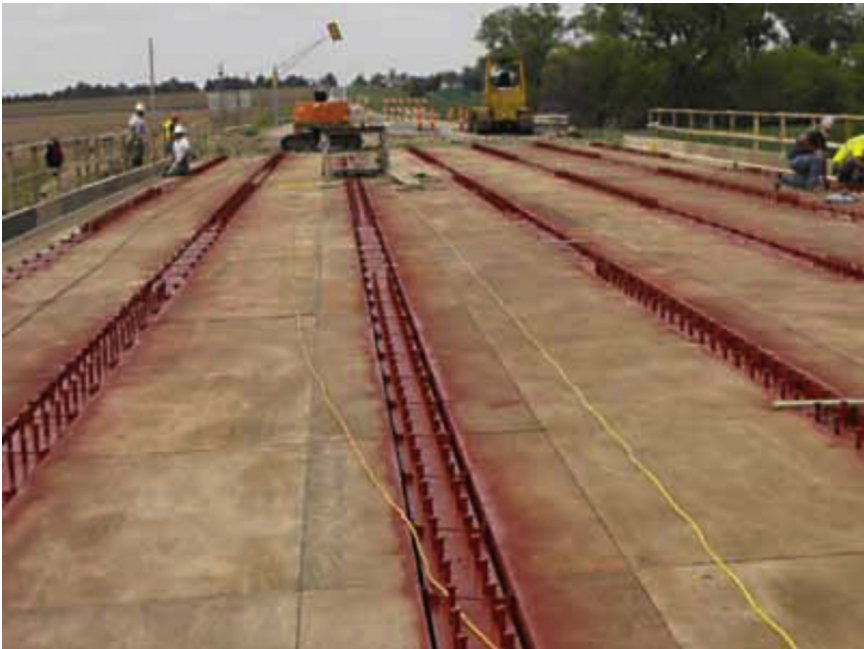
Figure 5.67 Deck Forming for Redeck Project.
