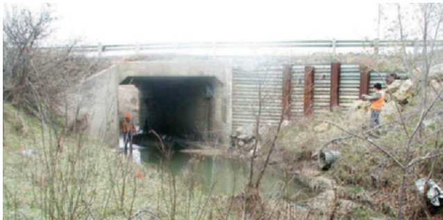
Figure 2.9 Concrete Wingwall and Temporary Wingwall.
