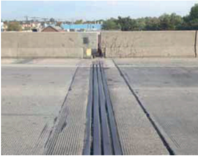
Figure 5.38 Modular Joint Expansion Joint.
