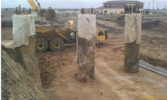
Figure 2.22 Drilled Shafts.
