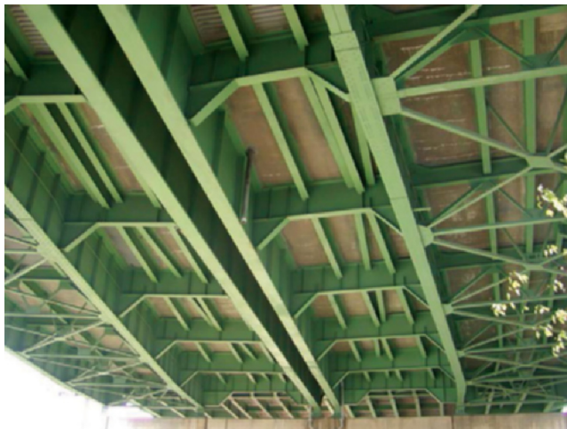
Figure 2.41 Stringer and Floorbeam System.
