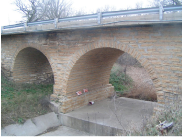
Figure 2.46 Stone Arch Bridge.
