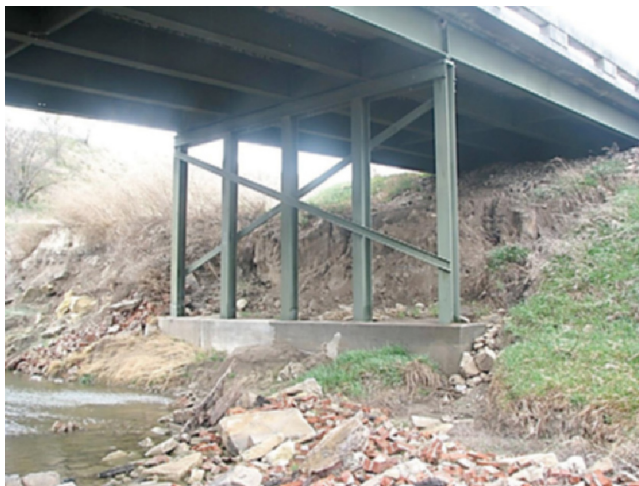
Figure 2.73 Steel Pile Bent.
