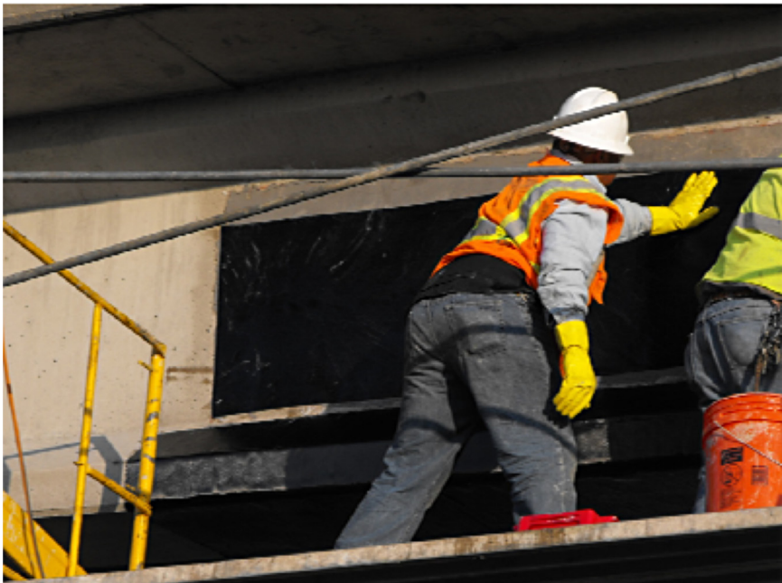
Figure 5.56 Installation of FRP Repair on Prestress Concrete Beam.
