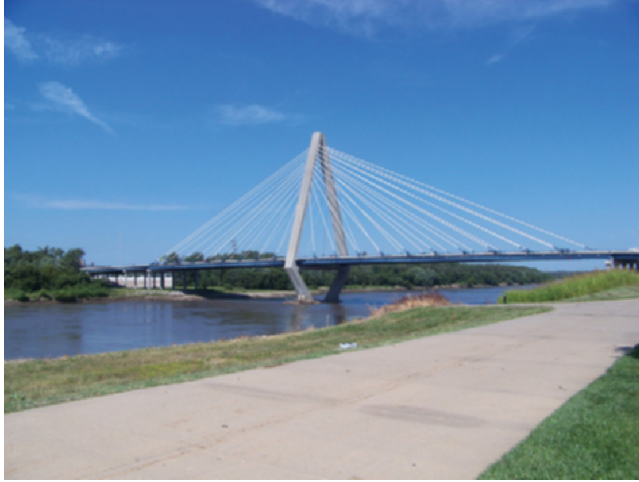
Figure 2.49 Christopher Bond Bridge – Cable Stayed.
