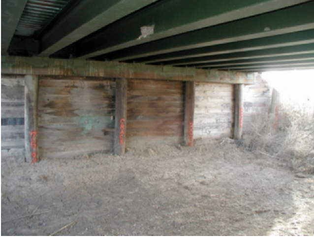
Figure 2.78 Timber Abutment Bent.
