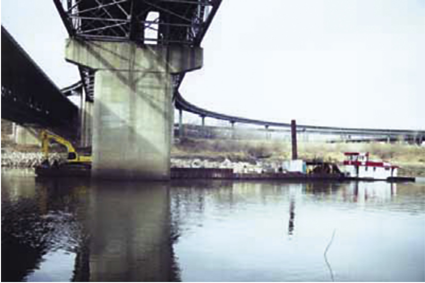
Figure 5.61 Placing Rock Around Pier in Missouri River.
