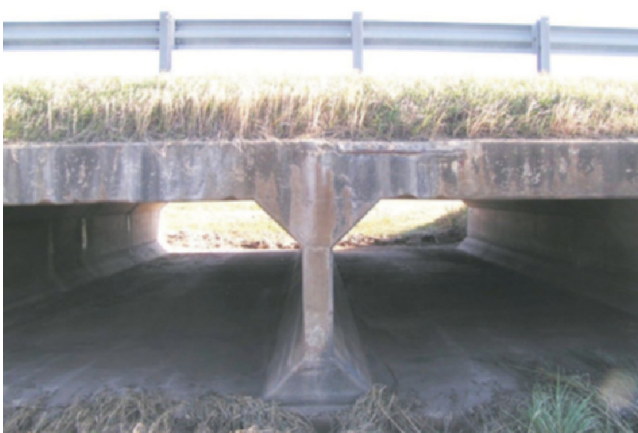
Figure 2.3 Fillet on Reinforced Concrete Box Culvert.
