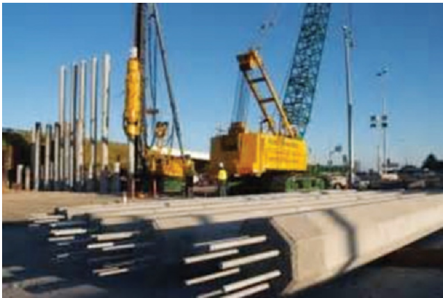
Figure 2.21 Concrete Piles.
