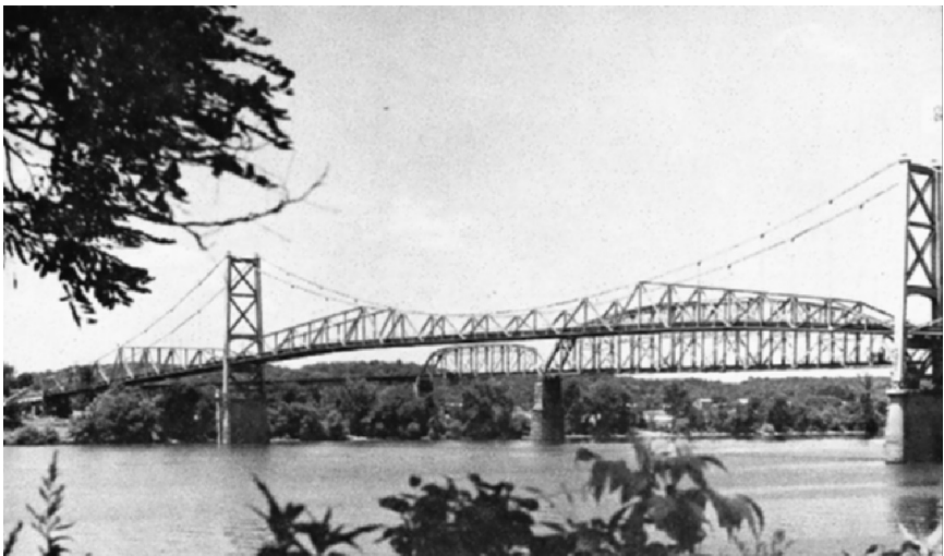
Figure 1.8 The Silver Bridge (in Foreground) . (From 1968 NSTB Report [14]).
