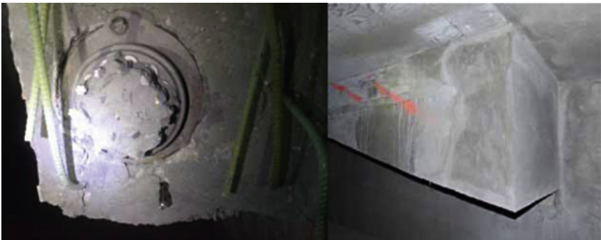
Figure 5.59 Repair of Posttensioning Anchorage.
