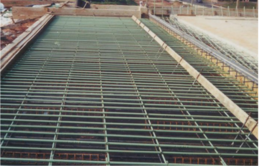
Figure 8.3 Reinforcing steel imbedded in the concrete slab.
