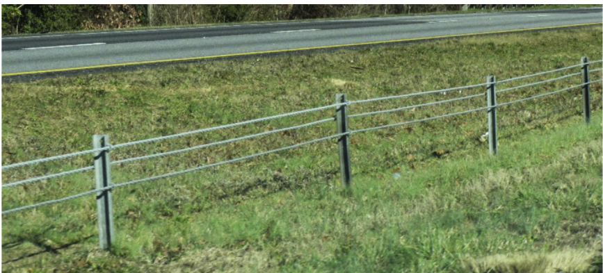
Figure 4.19 Flexible barrier (three-strand cable).
