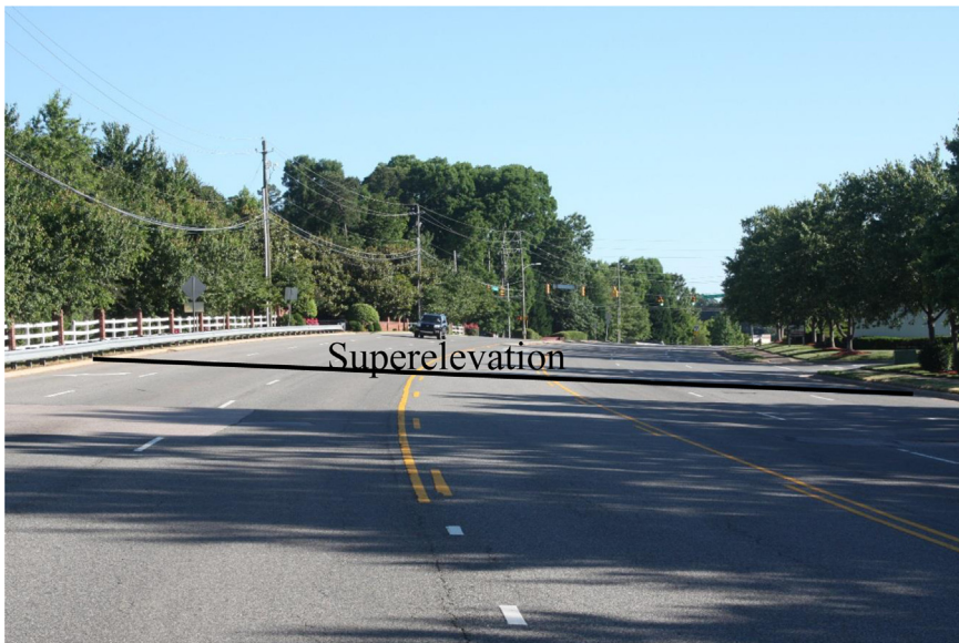
Figure 4.1 Superelevation in horizontal curve.
