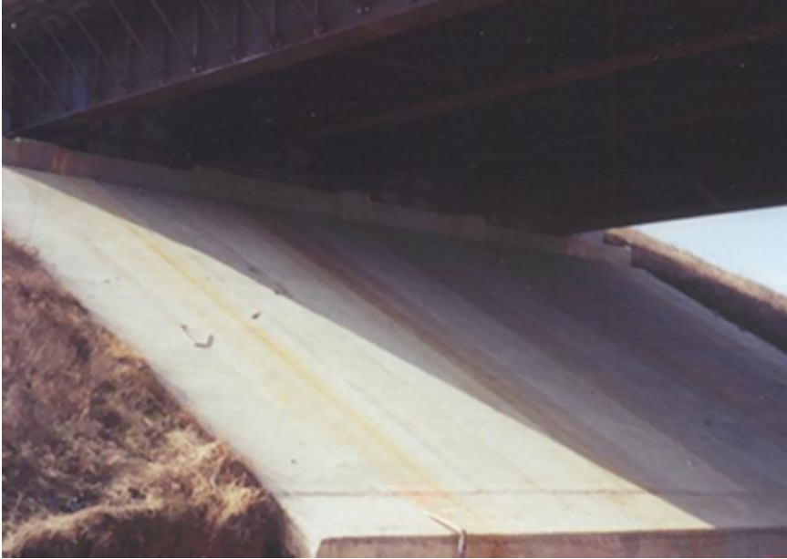
Figure 8.8 Typical slope protection.
