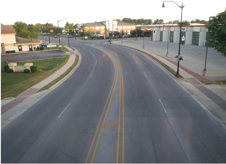
Figure 4.4 Collector roadway with pedestrian facilities and frequent access points.
