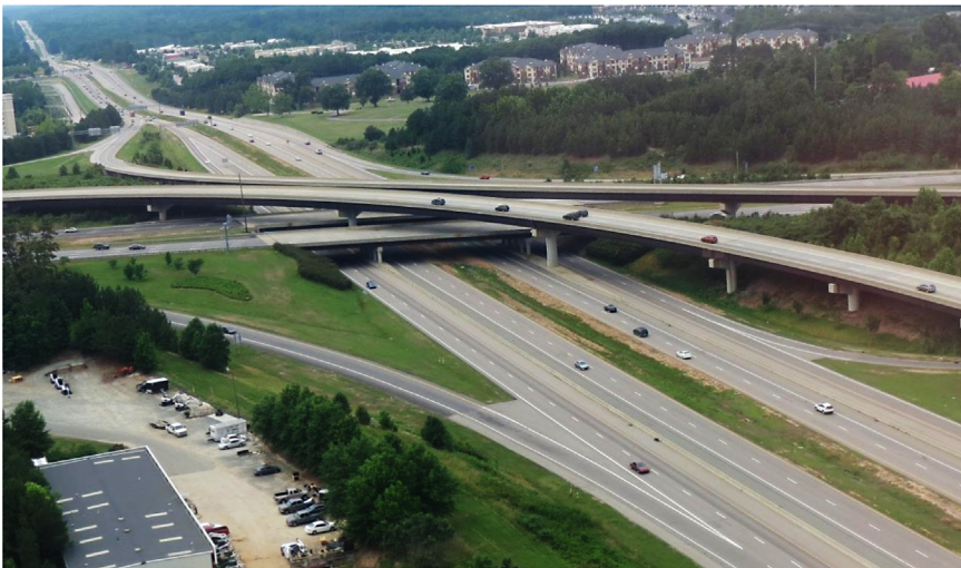
Figure 4.42 Interchange with directional ramps from one roadway.
