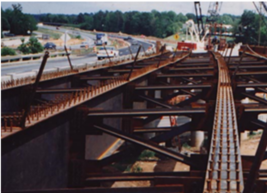
Figure 8.5 Diaphragm bracing for the steel girders.
