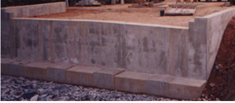
Figure 8.6 Typical end bent.
