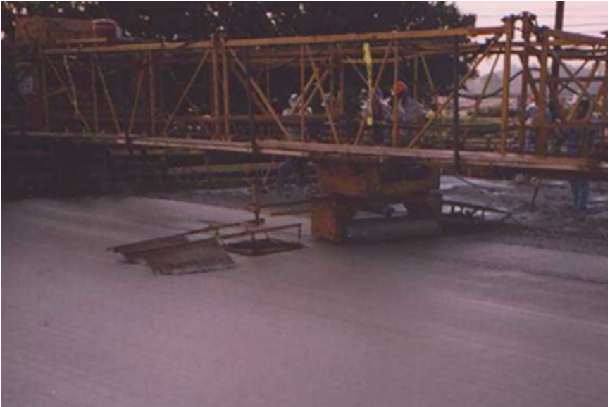
Figure 8.4 Concrete decking being screed.
