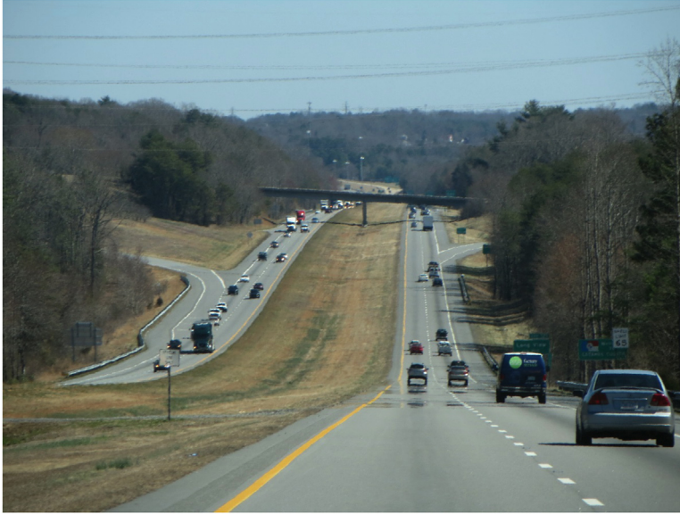
Figure 4.3 Typical rural freeway section with wide median.
