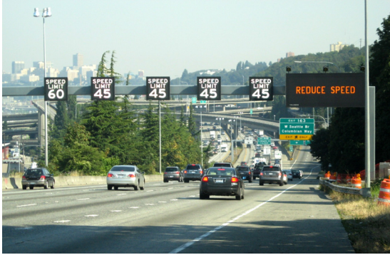
Figure 5.35 Variable speed limits used in Washington state in the United States. Source: http://www.wsdot.wa.gov/ .
