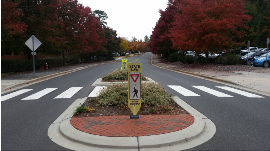
Figure 4.8 Horizontal feature for pedestrian refuge and speed reduction at crosswalk.
