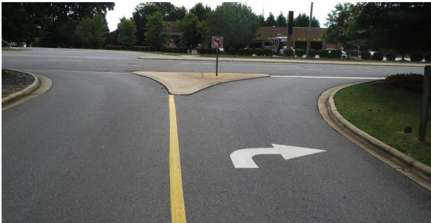
Figure 4.30 Channelization to restrict left turns.
