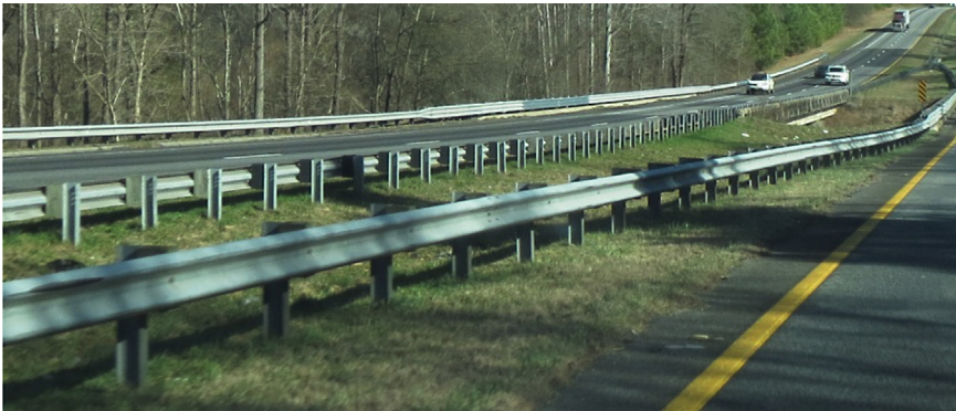
Figure 4.21 Semirigid barrier (W-beam with steel post and wood block).
