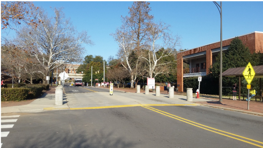
Figure 4.9 Vertical feature for pedestrian crossing and speed reduction at crosswalk.
