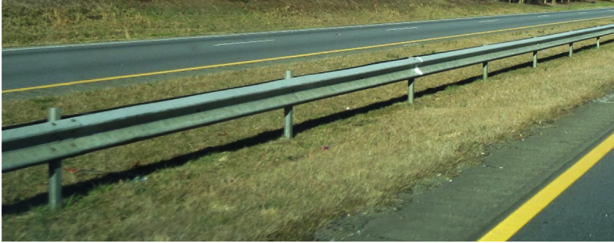
Figure 4.20 Flexible barrier (W-beam with weak steel post).
