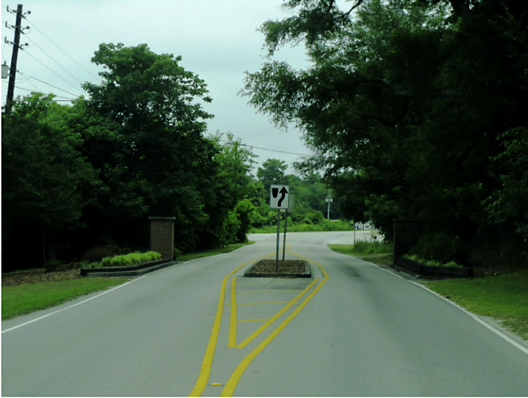
Figure 4.7 Horizontal feature for transition to low speed residential area.
