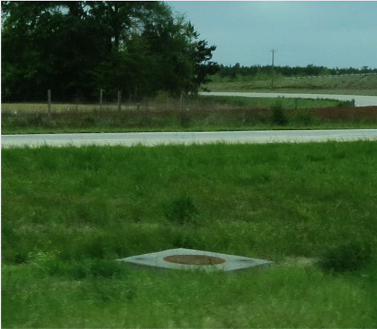
Figure 4.18 Raised concrete drop inlet in highway median.
