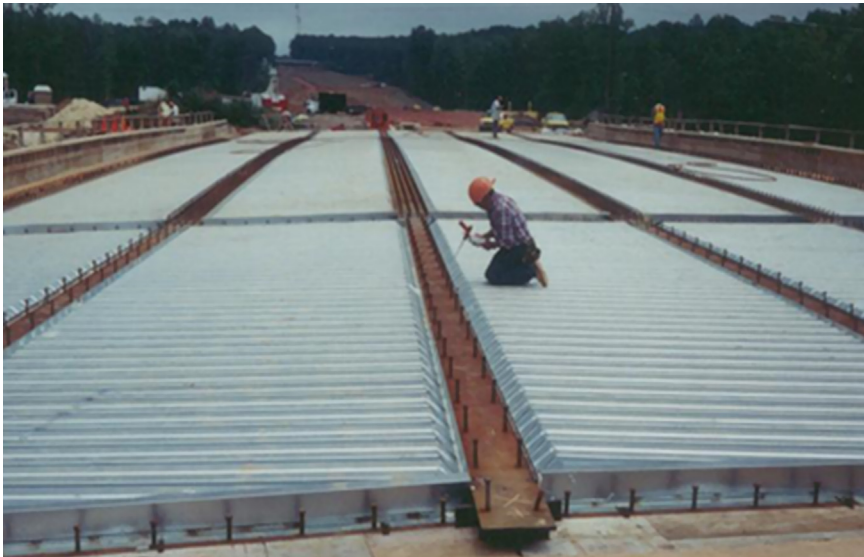
Figure 8.2 Deck forms being installed.
