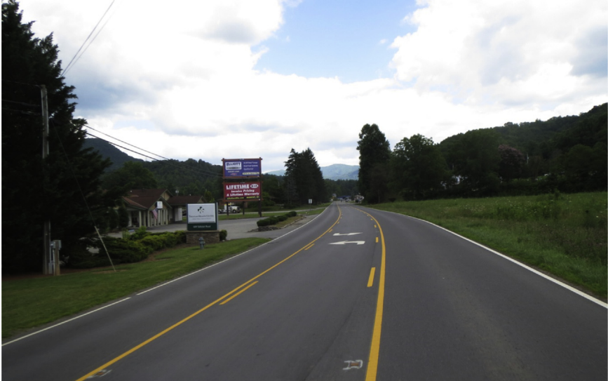
Figure 4.17 Three-lane configuration with two-way left-turn lane.
