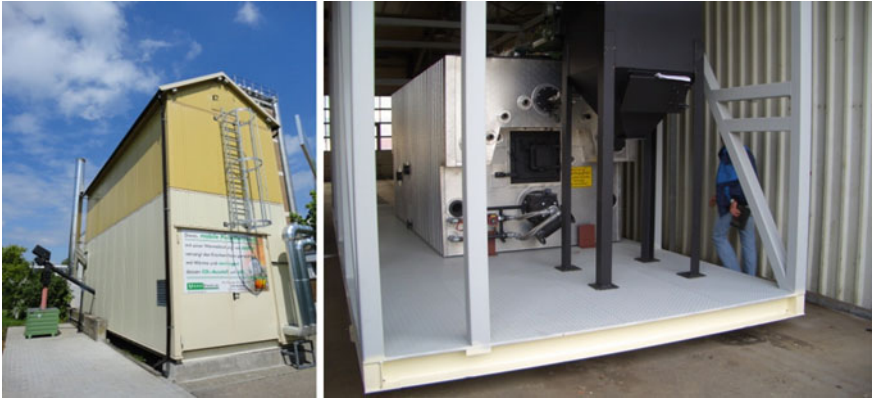
Fig. 7.26 880 kW pellet boiler by Weiss in a container, supplied by Mann Naturenergie GmbH & Co. KG, Langenbach [13]
