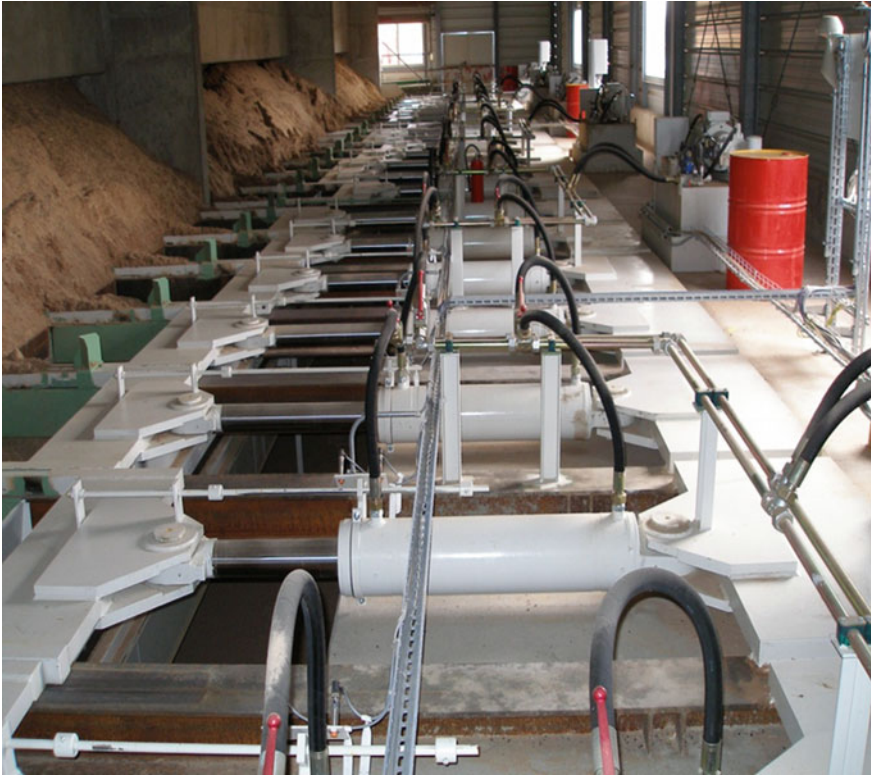
Fig. 6.16 Push-floor and hydraulic cylinders for chips, by Rudnick & Enners [2]
