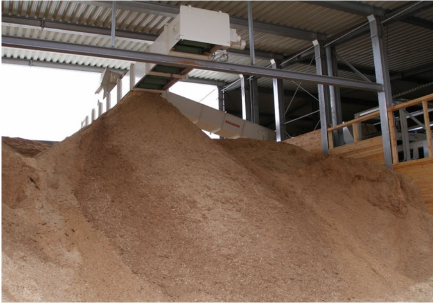
Fig. 6.15 Wet-chip store filled by scraper chain conveyor, weather protected [2]
