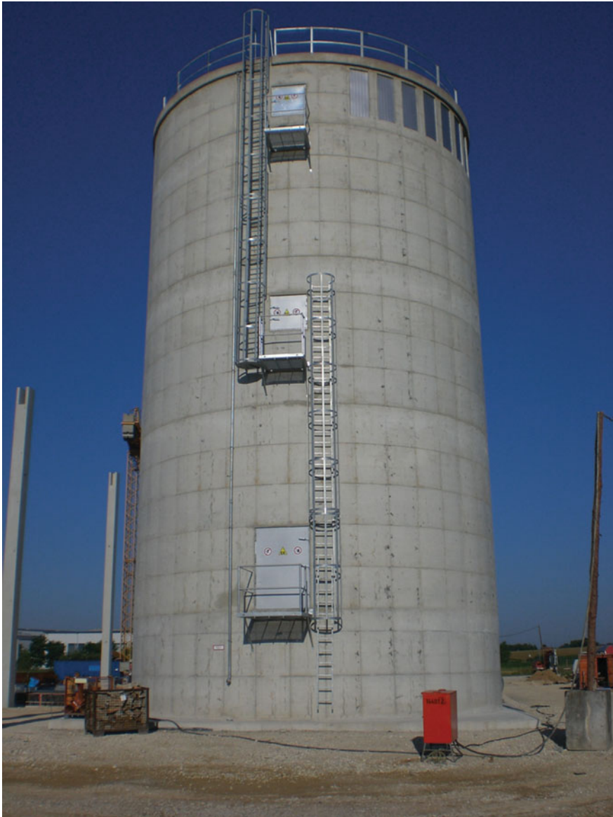
Fig. 6.37 Reinforced concrete shavings silo by Wolf System GmbH [7]
