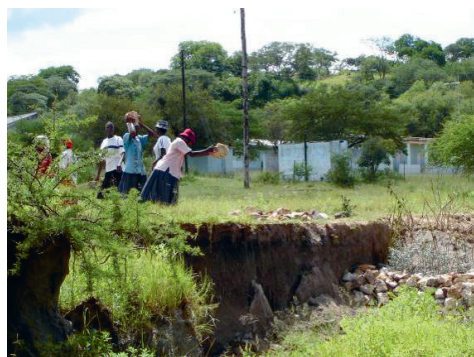
Figure 5.4 Women fill a part of the Gobalidanke gully with stones
