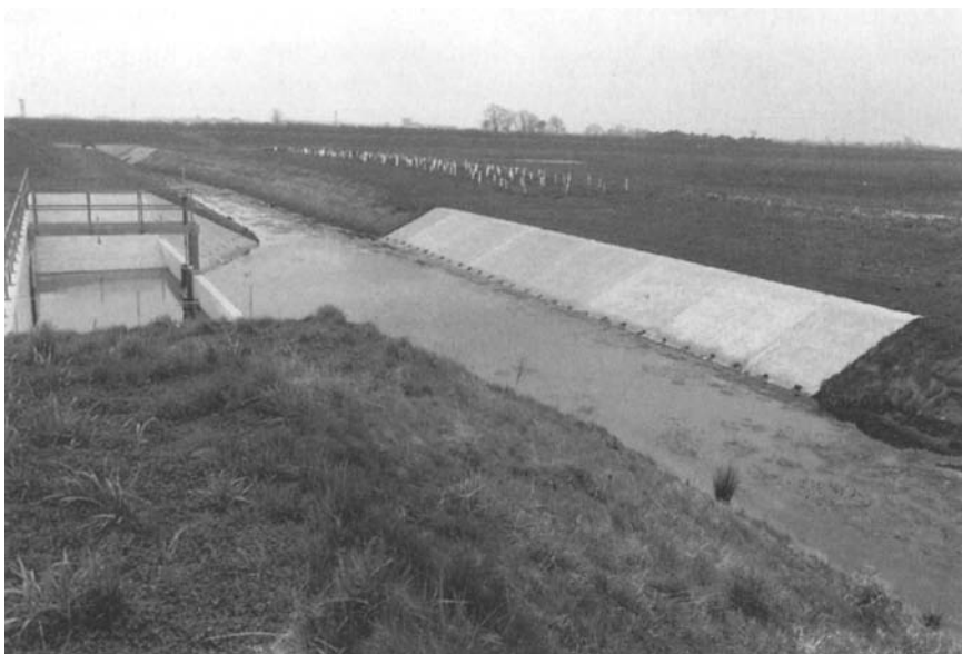
Plate 7.1 (b) At high flows water which would normally flood Lincoln is now released on to this floodplain farmland (photo M. D. Newson).
