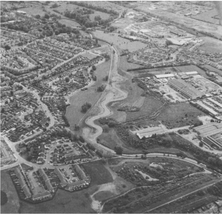
Plate 6.4 The restored River Skerne, Darlington, UK, showing the introduced meanders and rehabilitated floodplain (photo copyright AirFotos, Newcastle upon Tyne).
