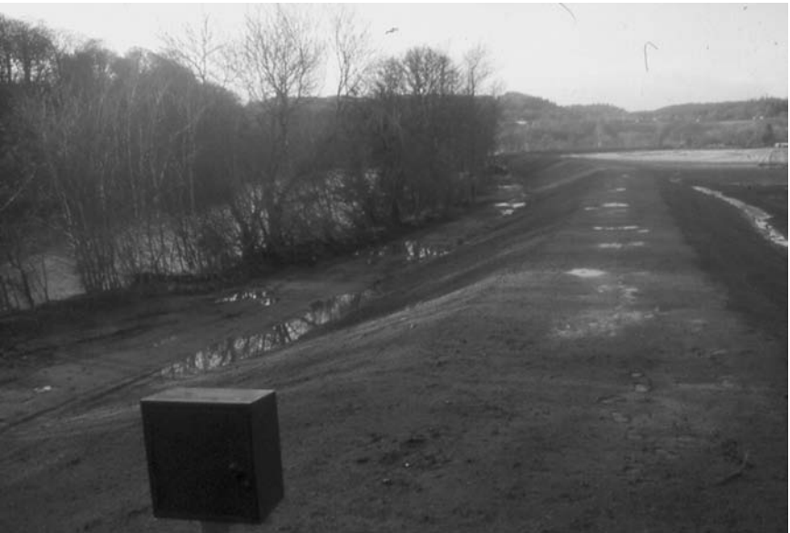
Plate 7.2(b) The new flood bank completed.
