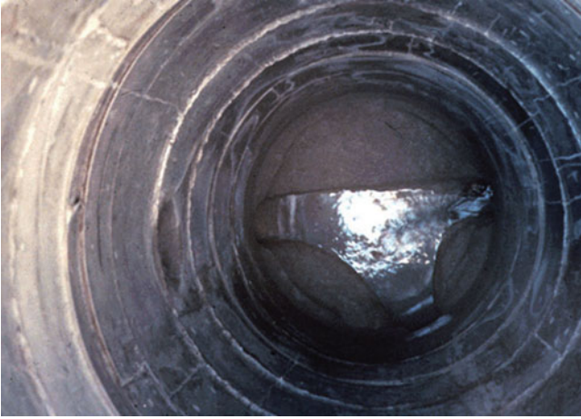
FIGURE B-14. Formed-in-Place Installation.
