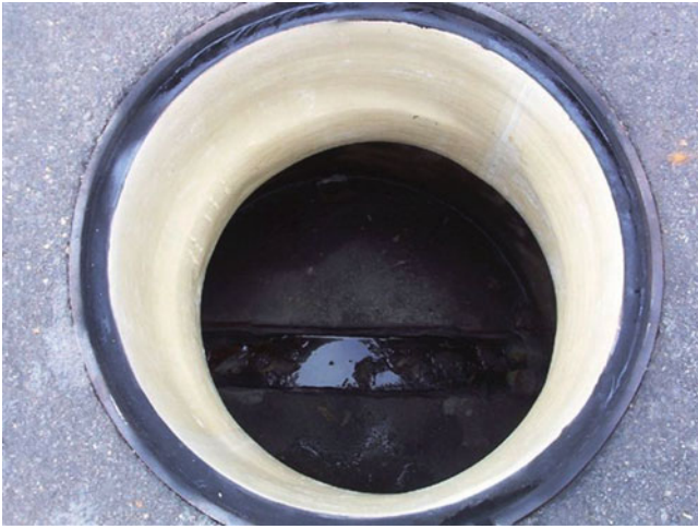
FIGURE B-9. Cured-in-Place Manhole Seal.
