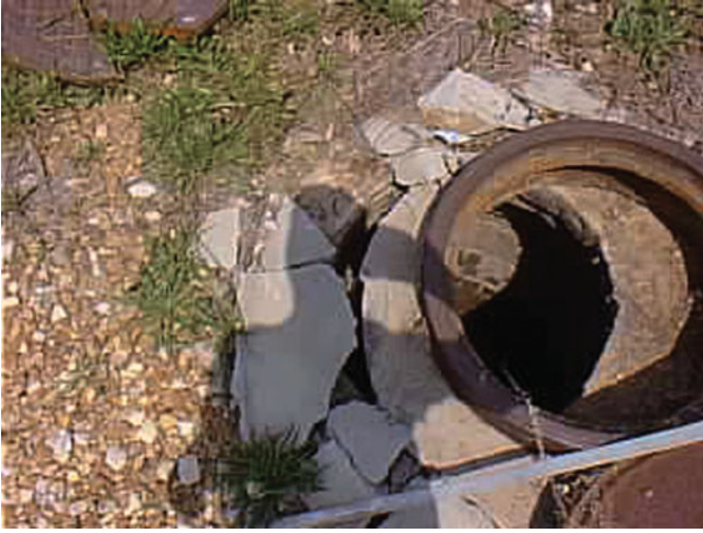
FIGURE B-1. Displaced Ring.
