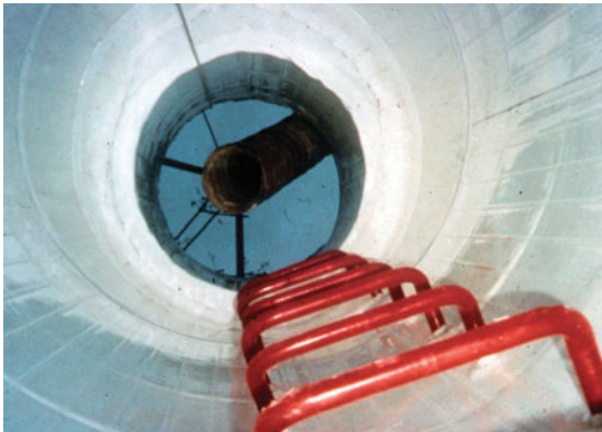
FIGURE B-15. Thermoplastic Liner Installed with Formed-in-Place Concrete.
