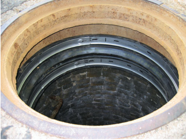
FIGURE B-7. Mechanical Seal.
