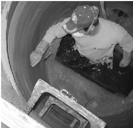
FIGURE 7-2. Cement Thickness Inspection.
