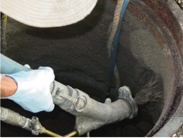
FIGURE B-12. Shotcrete Application.
