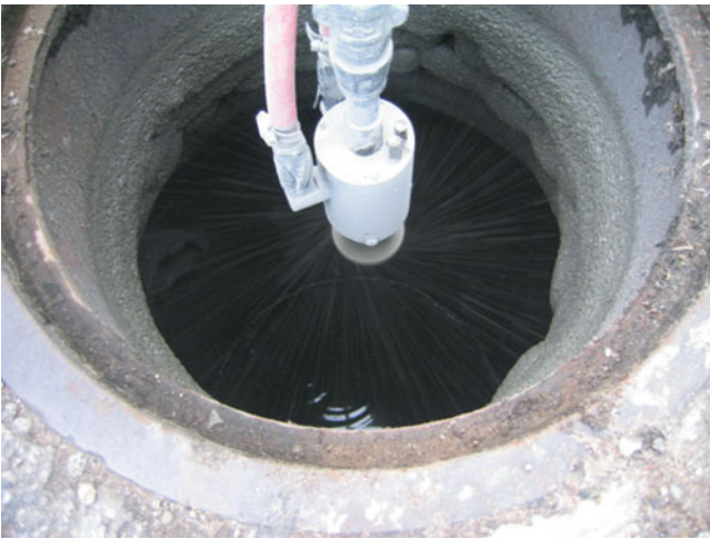
FIGURE B-13. Spincast Application.
