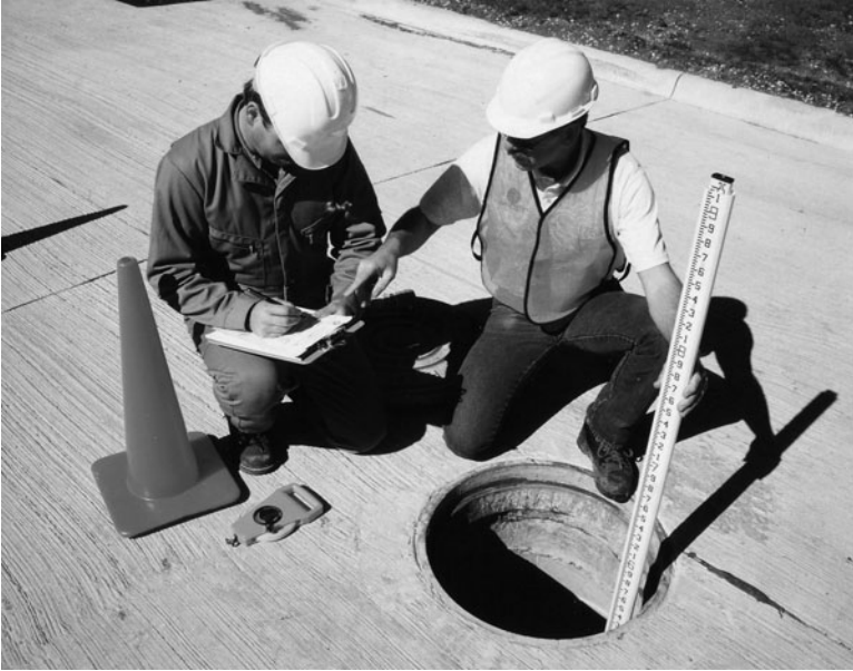
FIGURE 3-3. Using a Survey Rod to Obtain Rim-to-Invert Distances.
