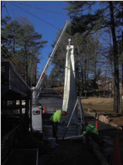
FIGURE B-19. Cured-in-Place Manhole Liner.
