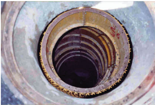
FIGURE B-14. Formed-in-Place Installation.
