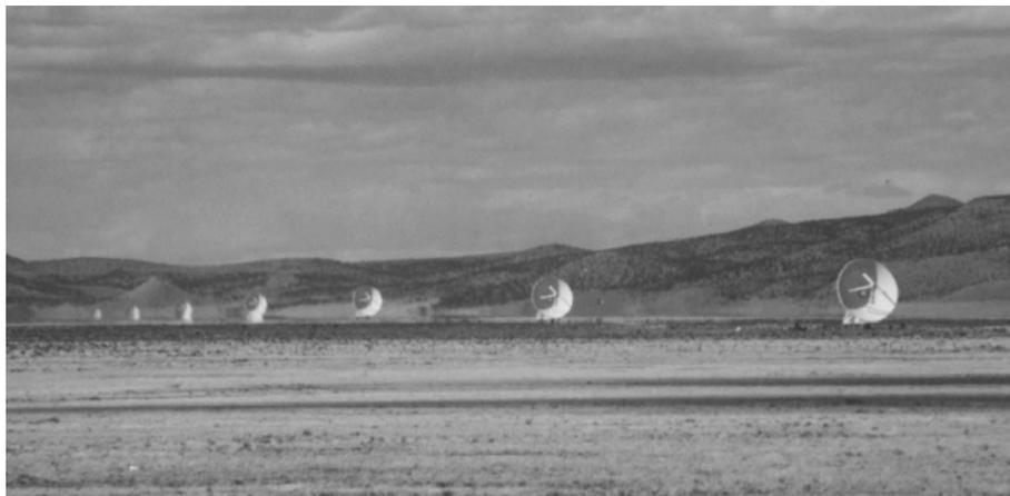
**Fig. 4.10.** The antennae of the north arm of the Very Large Array stretch into the distance, distorted by a summer mirage on the high plains of New Mexico. The whole instrument includes 27 dishes, which can be deployed in a Y-shaped pattern spanning as much as 36 km in extent. Since its completion in 1978, the VLA has been a centerpiece of radio astronomy not only for US investigators, but for astronomers worldwide.
