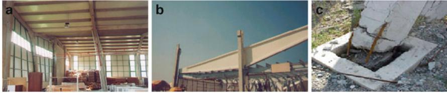
**Fig. 8.2** Observed damages. (a) Out of plane deformations of plane frames; (b) Collapse of a rigid roof beam; (c) Plastic hinge at column base
