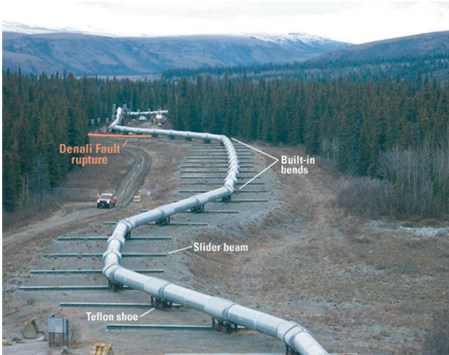
**Fig. 10.8** Trans-Alaska Oil Pipeline and Denali Fault crossing (USGS 2003)
