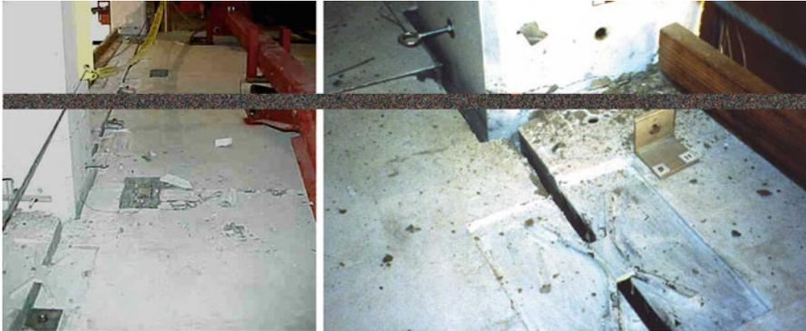
**Fig. 13.15** “X-connectors” between precast floor (pre-topped double-tee) units and frames as implemented in the PRESS Five Storey Building (Priestley et al. 1999)
