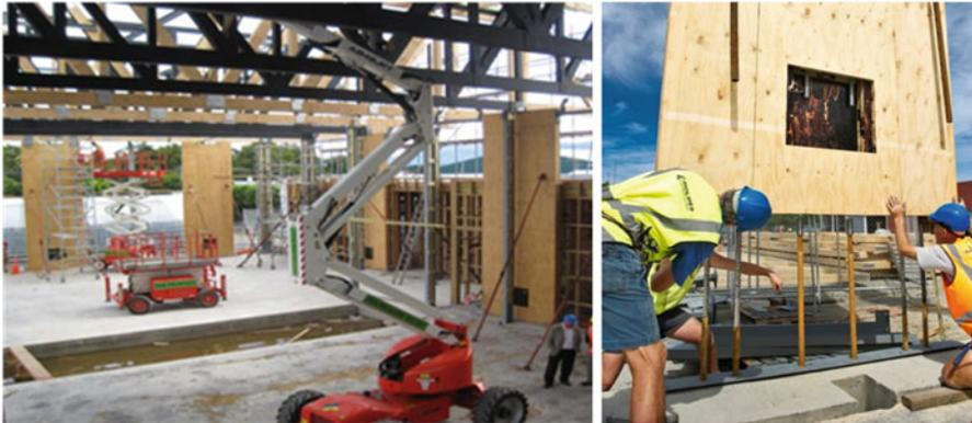
**Fig. 13.28** Carterton Events Centre, New Zealand. Single-storey building with LVL truss roof (Designed by Opus International: Dekker et al. 2012)
