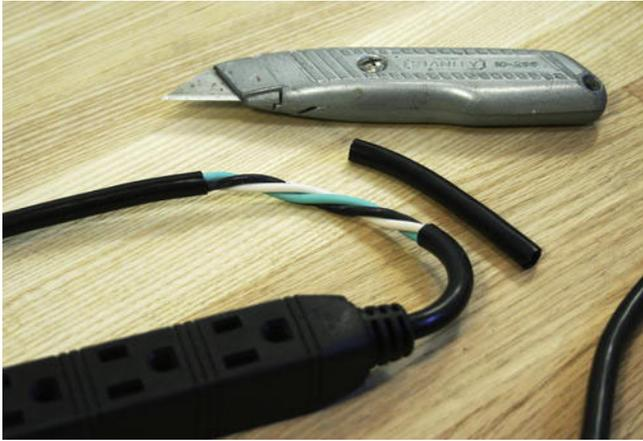
**Figure 7-6.** Outer insulation removed from power cable
