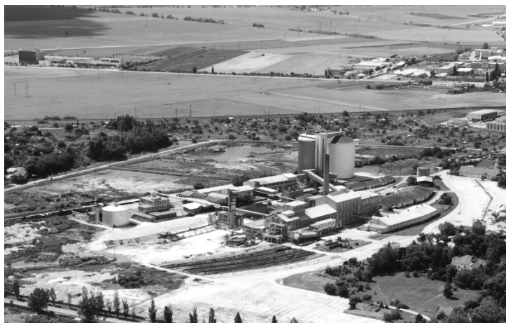
Fig. 1. Industrial plant location
